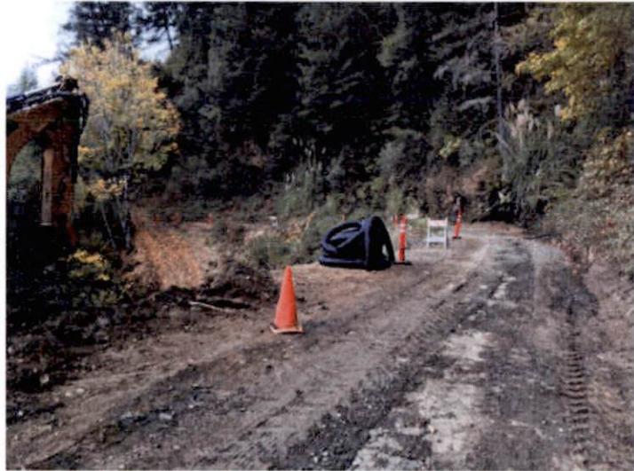
Photo No. 13. Emergency road repair at slide, very unstable roadbed.
