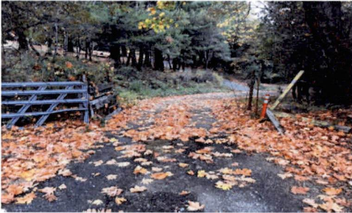
Photo No. 8. 12'- wide cattle guard, gravel surface, with inter-visible turn outs.
