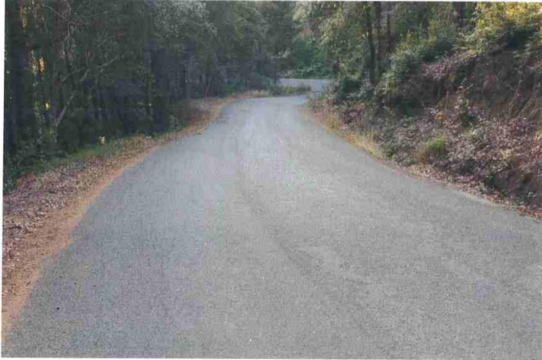
Photo 16. Mile 1.5: 20-ft road width with 1-ft shoulders.
