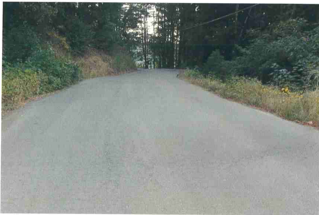
Photo 8. Mile 1.2: 24' width, 1' shoulders.
