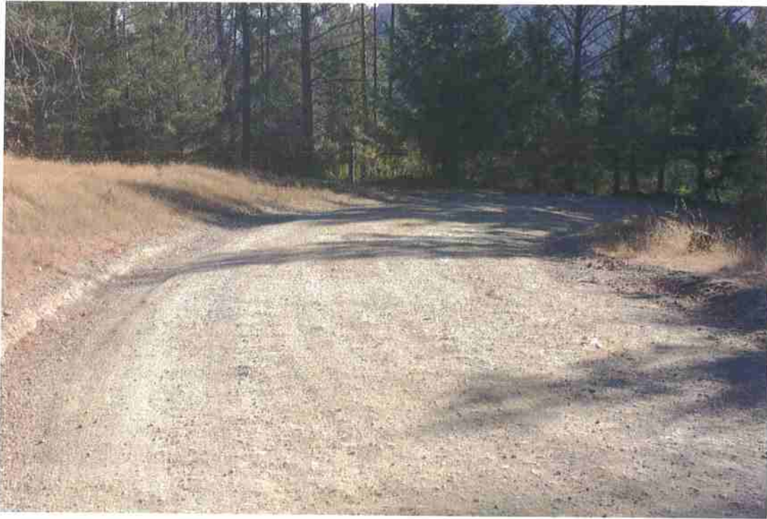
Photo 3. Mile 0.3: 20-ft road width with 2-ft shoulder.
