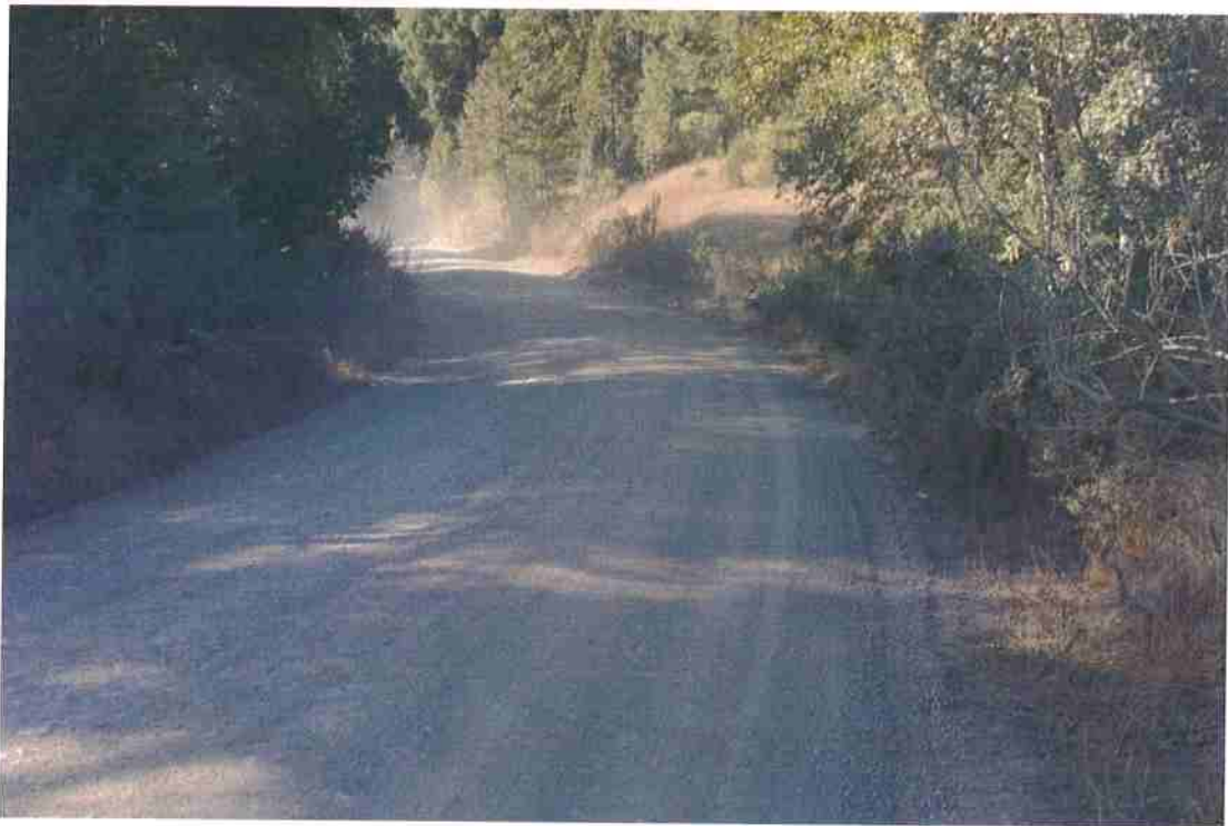
Photo 18. Mile 1.5: 18-ft road width with 1-ft shoulders.
