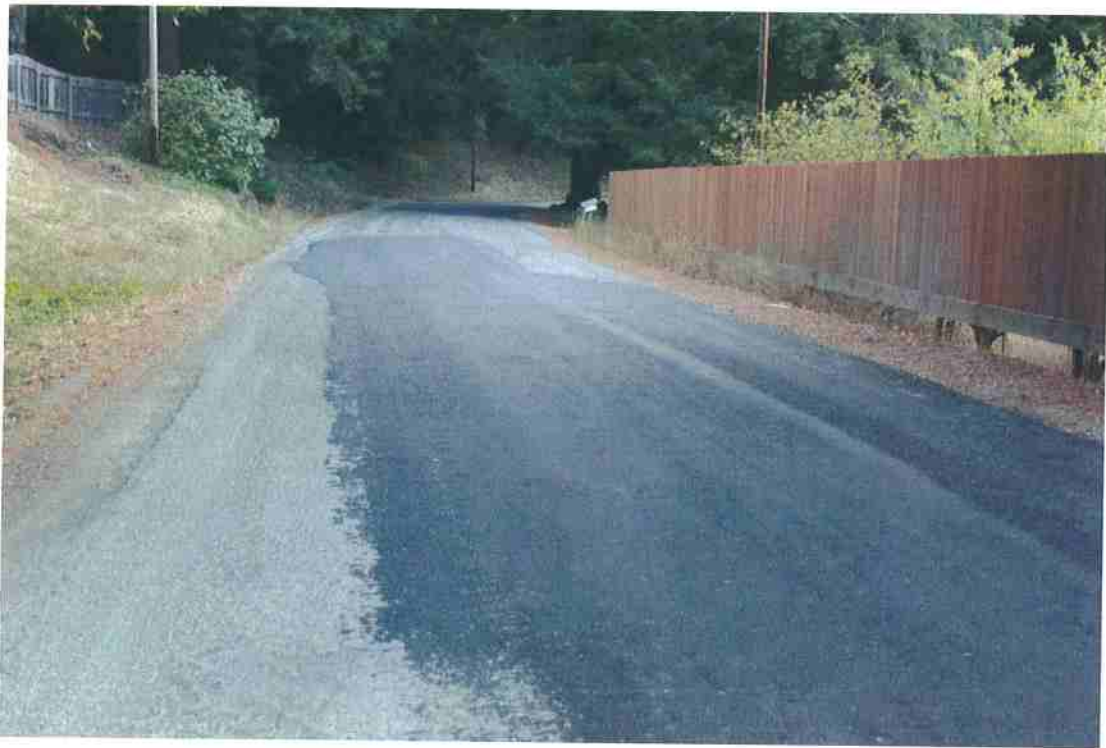
Photo 10. Mile 1.4: 22' width, 2' shoulders.
