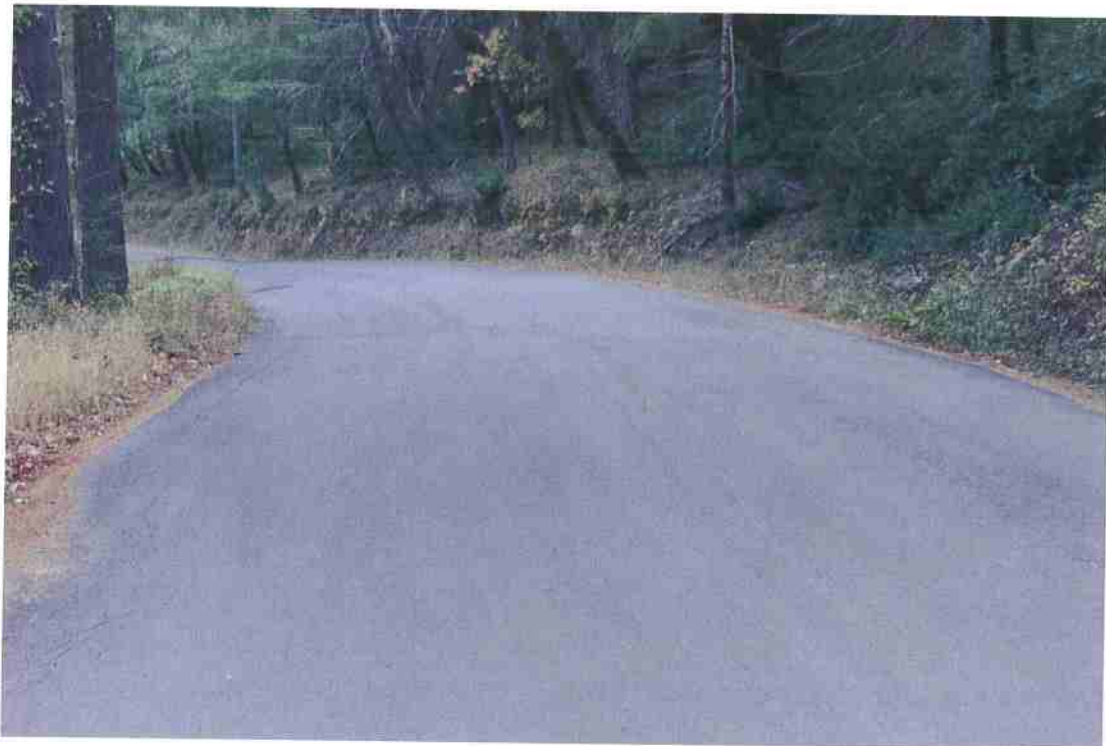
Photo 12. Mile 1.1: 20-ft road width with 2-ft shoulders.
