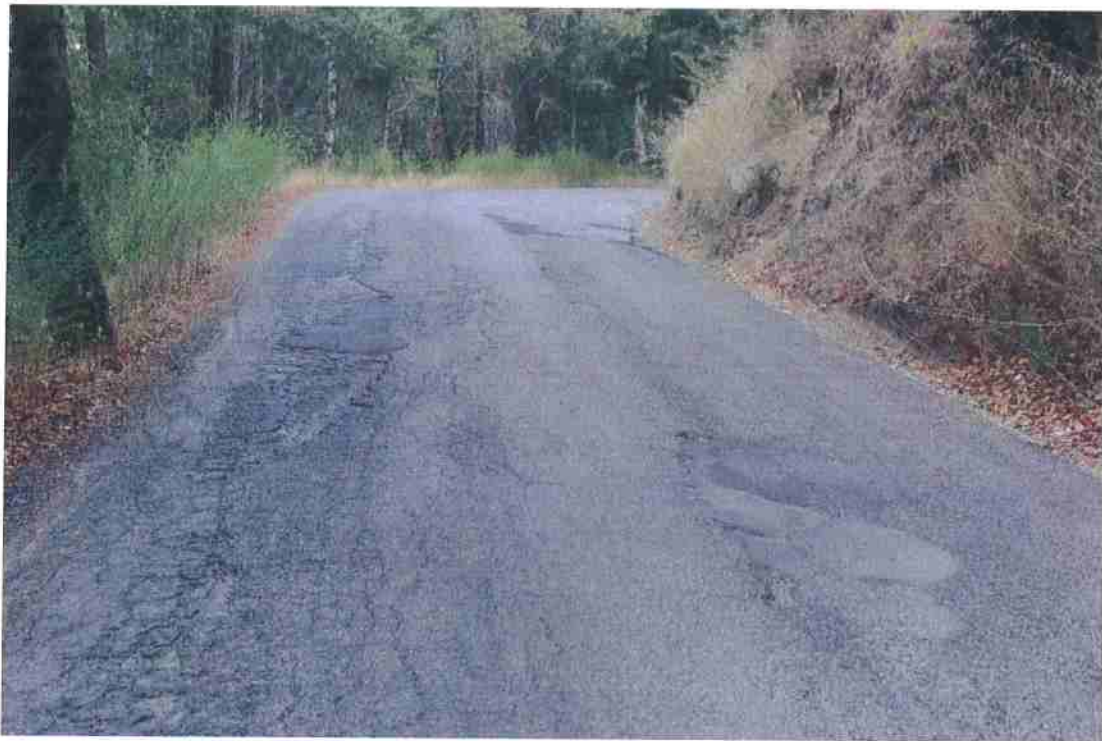
Photo 6. Mile 0.5: 18-ft road width with 1-ft shoulders.
