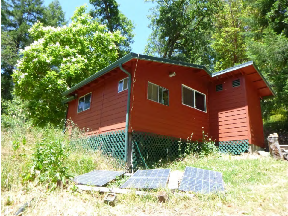
Photo 5. Red Cabin, Looking Northwest.
