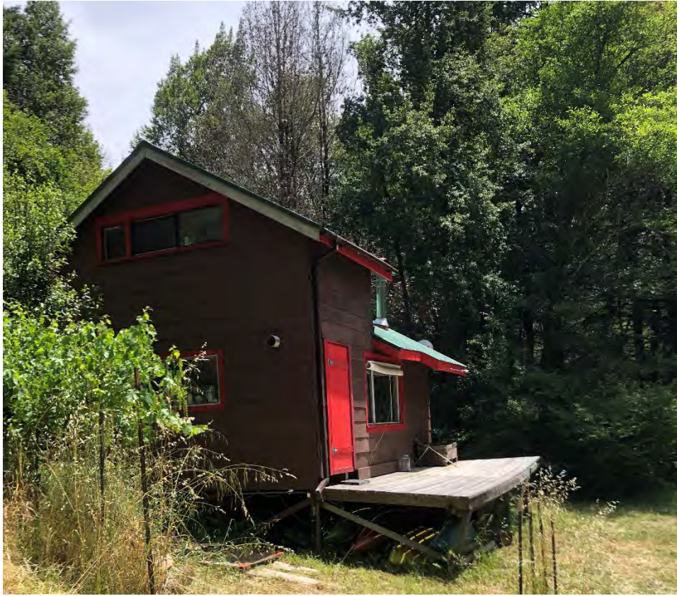
Photo 7. Creekside Cabin, Looking Southeast.
