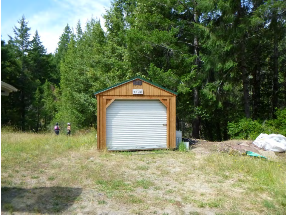
Photo 9. Shed1 is located near (south) Cultivation Area 1, Looking West.
