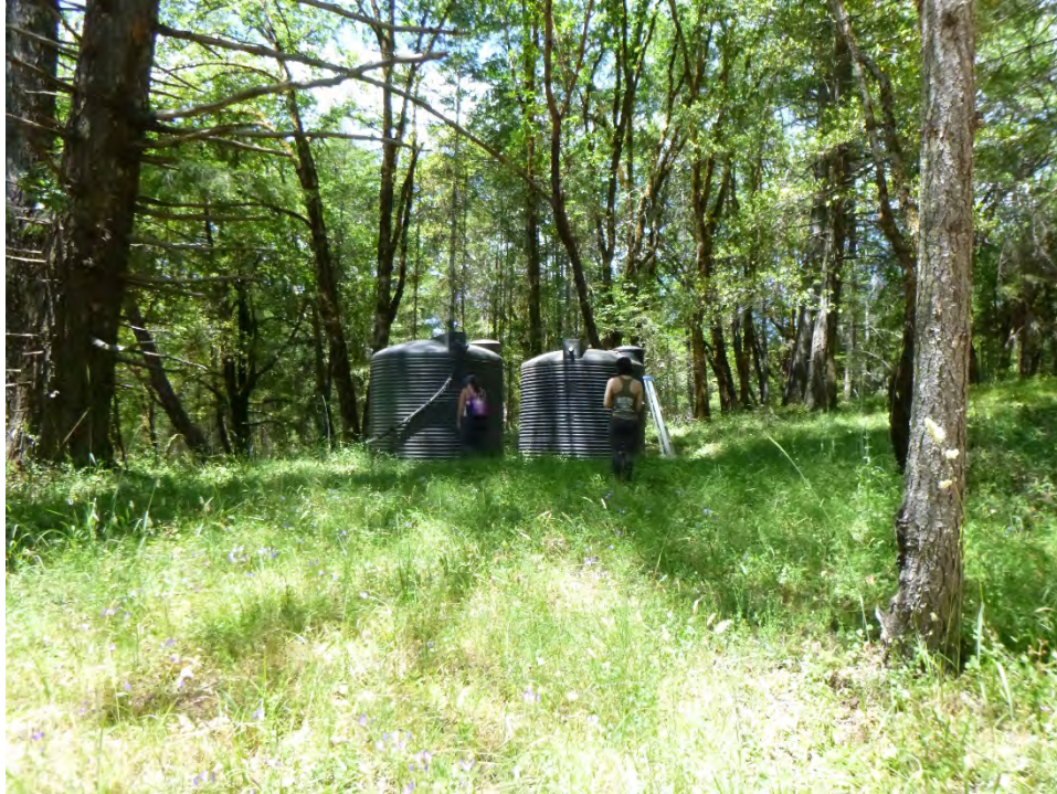
Photo 15. Water storage North (2 x 2.5K), Looking West.
