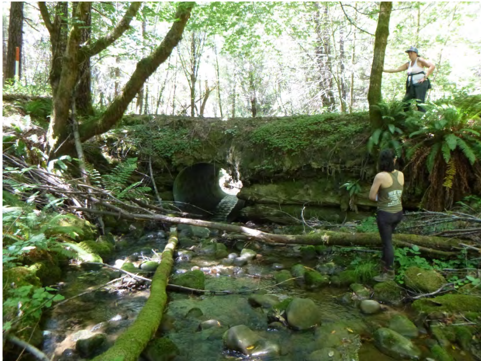
Photo 12. Miller Creek Road crossing over Buck Gulch, Looking Downstream.
