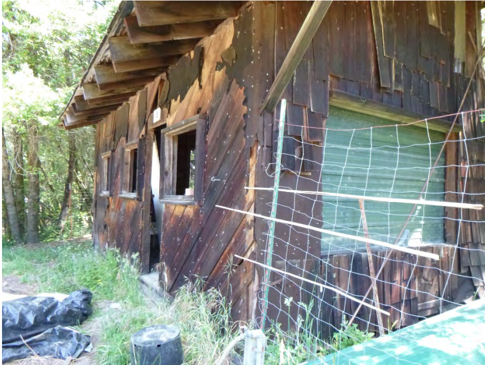
Photo 8. Shed3. Unused legacy structure adjacent to Cultivation Area 1, Looking North.
