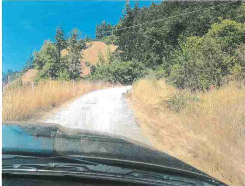
Figure 14: Turnout area to the right to allow vehicle passing, ~STA 59+38FT.
