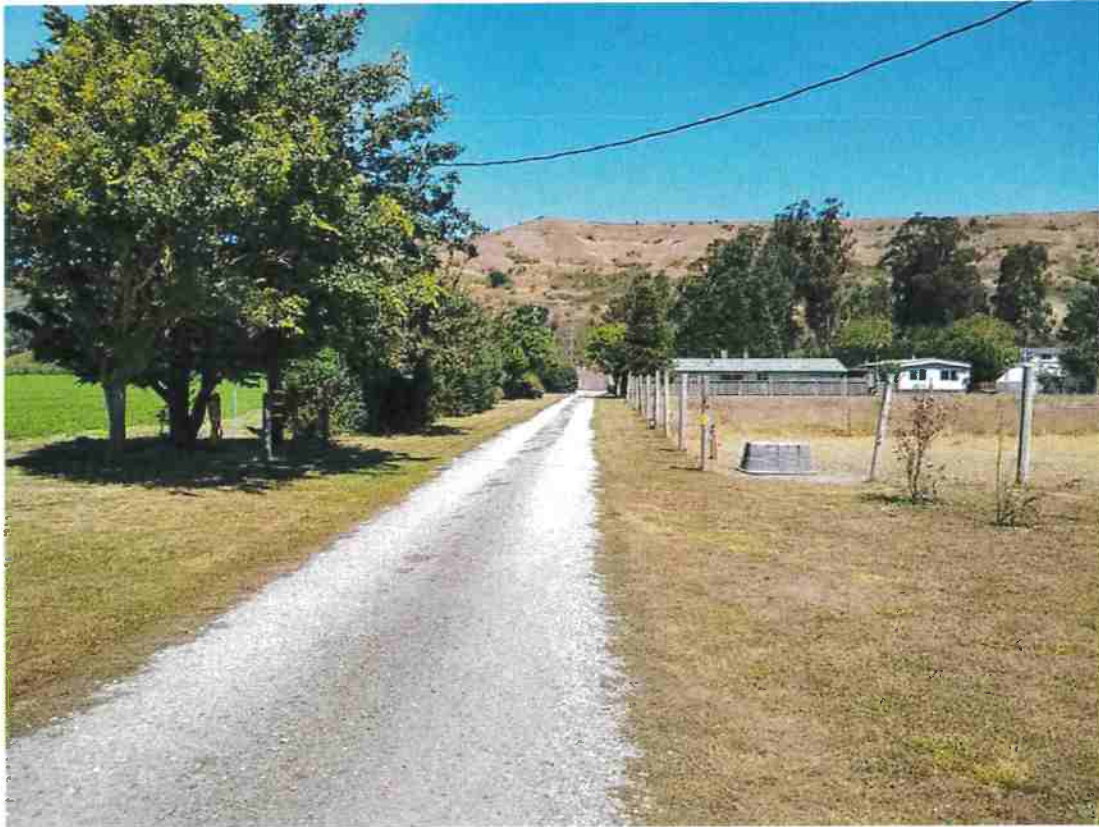
Figure 3: A representative portion of access road on the parcel displaying flat, vegetated shoulders.
