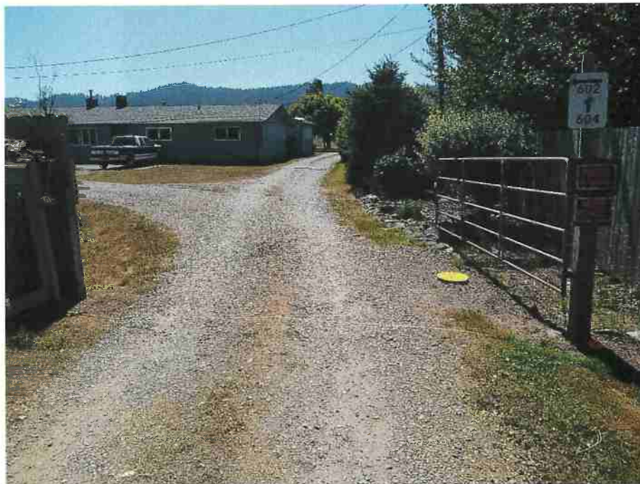
Photo 4. Mile 0.10 looking south. Gate is a pinchpoint at 16.5 ft wide. Hillcrest Drive ends at the residence. The first turnout is proposed to be constructed across from the residence. Turnout construction and brush removal will open a line of site to the remainder of the Road.
