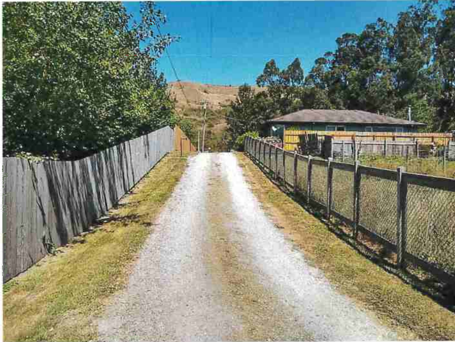
Photo 3. Mile 0.10 looking north: 10.5 ft road width with 3.5 and 2.5 ft shoulders
