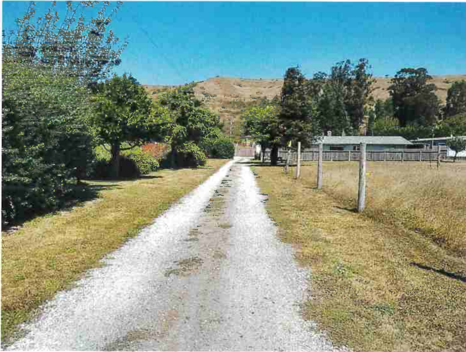
Photo 5. Mile 0.16 looking north: 10.5 ft road width with 6 ft shoulders.
