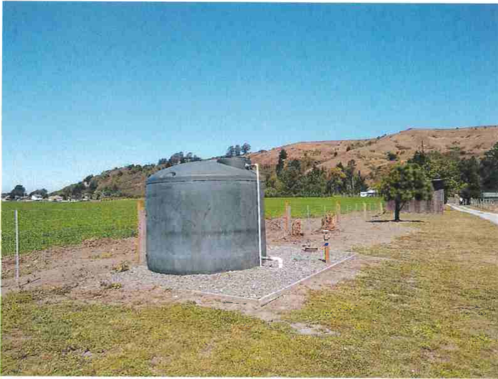
Photo 5. Emergency water tank with fire hose fitting. water.
