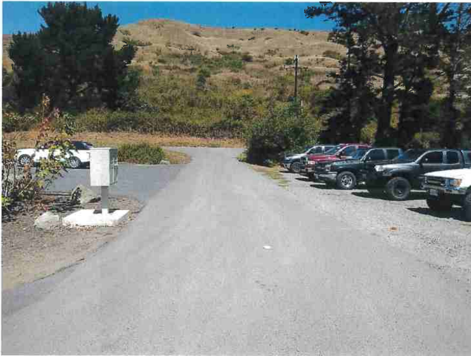
Photo 1. Mile 0.025 looking north to intersection with SR-36. Paved roadway is 16 ft wide.
