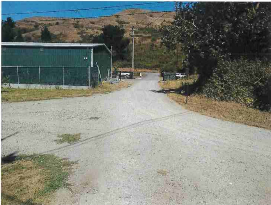
Photo 2. Mile 0.063: Gravel roadway is 14 ft wide with 4 ft shoulders. Hillcrest Drive is intersected by an unnamed road that provides an alternate access to SR-36 to the west.
