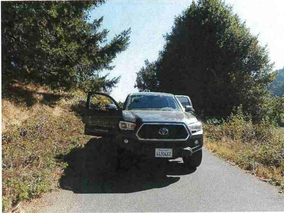
Figure 5: RP4. 14' Paved road width; Inboard ditch and location of lead-out ditch (Left in Image). Image shown facing East.
