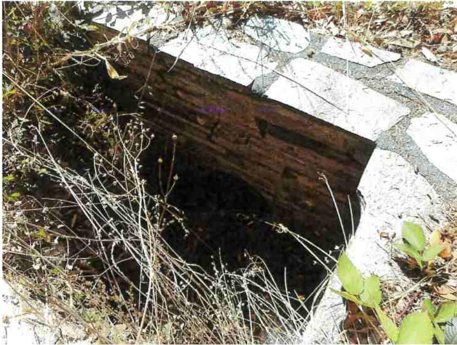
*Figure 7: RP4. Outlet of 12' ditch relief culvert.*
