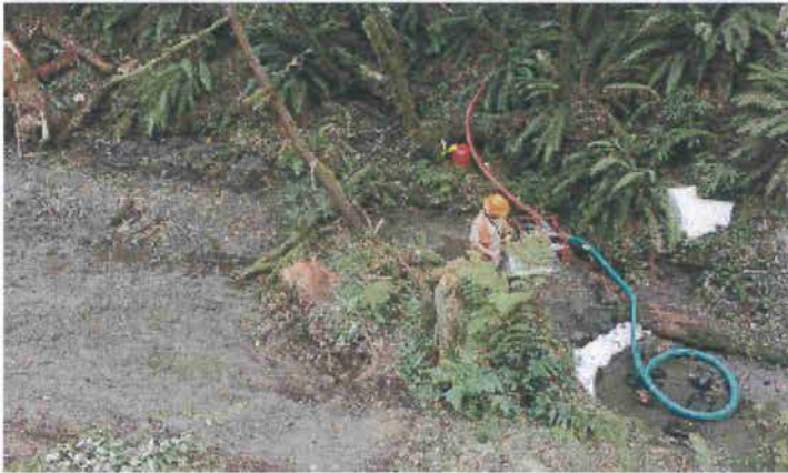
FIGURE 198. Sand bag retention dam on this small stream was used to pond streamflow so it could be pumped around a culvert installation site. The green intake hose is screened to keep out rocks and debris while the red pump hose extends several hundred feet around the project work area.
