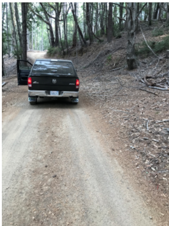
Figure 8. Depicts Turnout/Pass Point #6, general road surface conditions and debris in need of clearing to enhance functionality of turnout.
