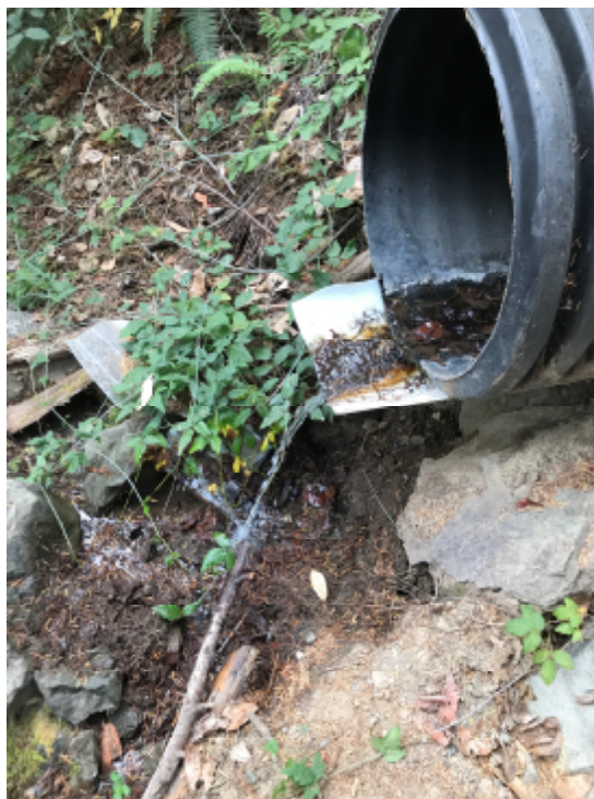
Figure 3. 24" HDPE culvert near Turnout/Pass Point #2. Depicts perched configuration and evidence of previous undermining.
