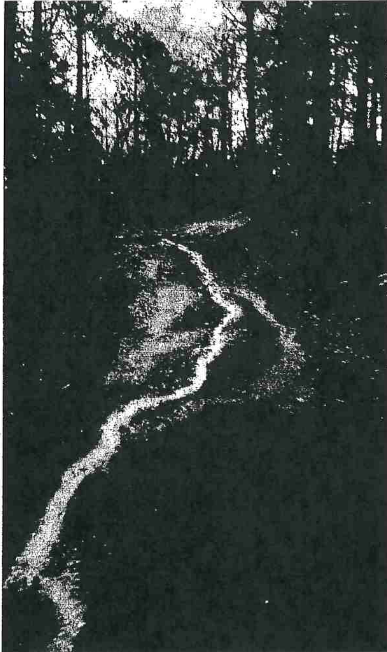
Picture 1: This is a photograph of Road Segment 1 described above. Road runoff being channeled along the road surface needs to be drained from the road surface by the installation of small drain dips. Dips need to be large enough that traffic will not destroy them. Photo date 1-19-2016.
