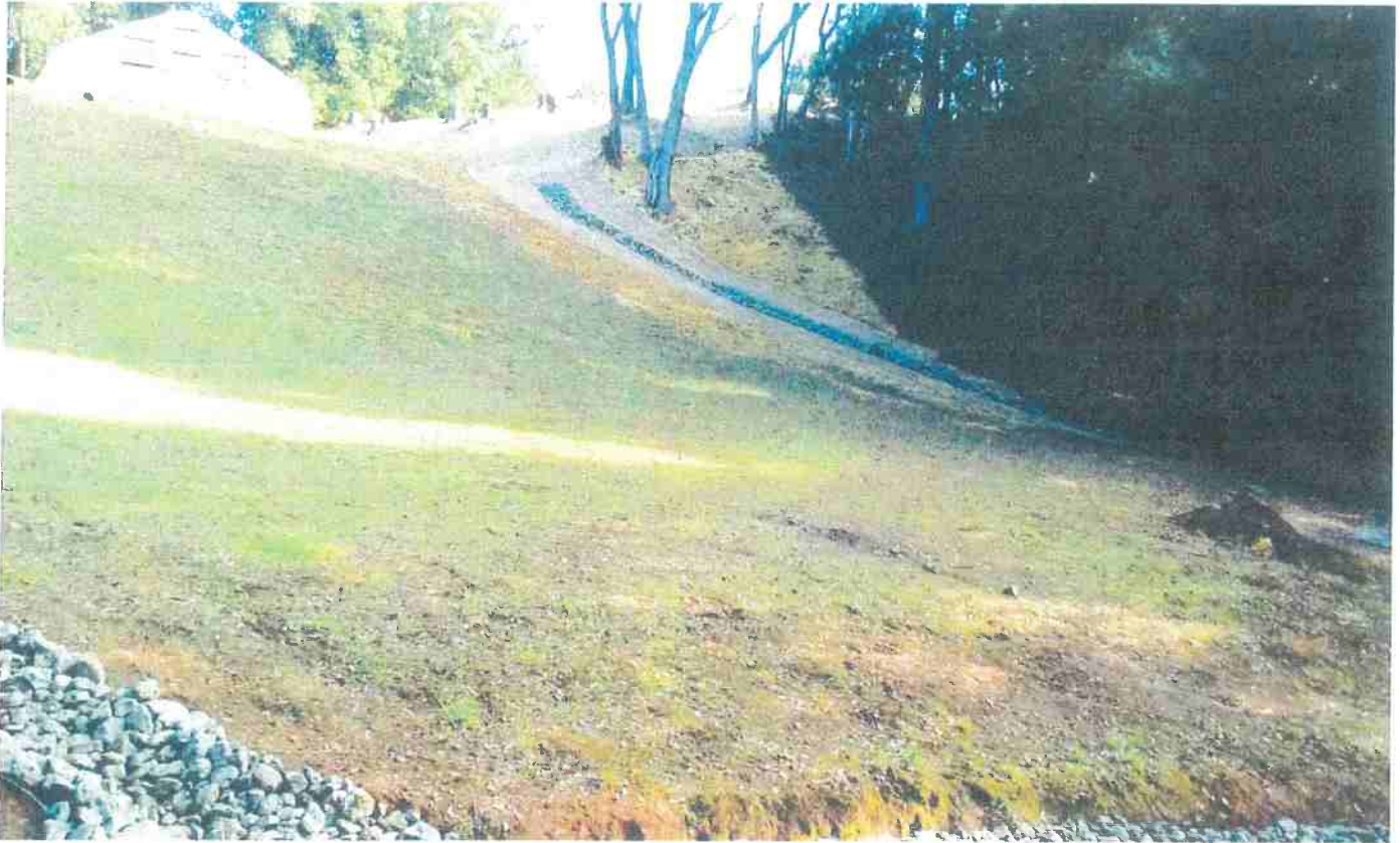
Picture 10: This is a picture of the newly rock lined drainage ditch (Map Point 2.5) that drains a "French drain" outlet that collects from the surface of the developed cultivation area. It ends above a swale that contains the top of a Class III watercourse and a Class II spring and POD. Photo date 12/2/2016
