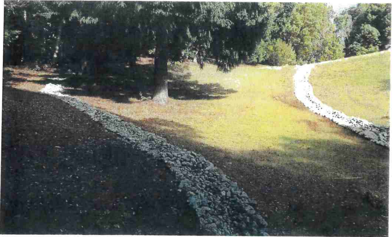
Picture 3: This is a picture of the newly rock lined drainage channels located upslope of Map Point 2. The channel on the left extends from the outlet of an existing ditch relief culvert. The channel on the right extends from the surface of the developed cultivation area. Photo date 12/2/2016
