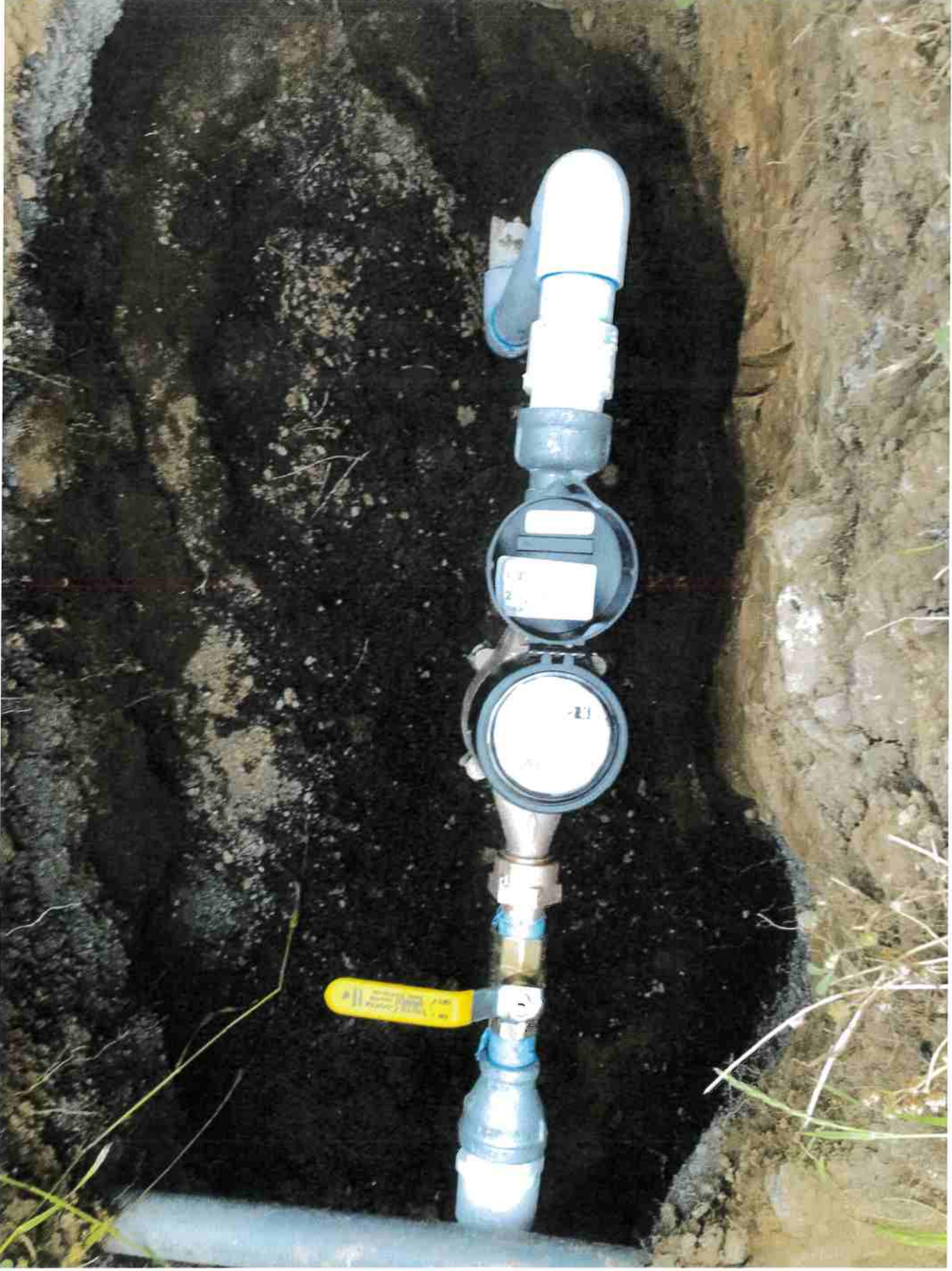
Item 1: Wellhead at Greenhouses 4 and 5
