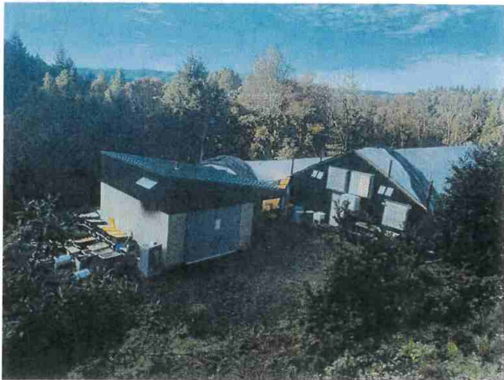
Photo 8: Site I. Photo date 1-17-2022.
