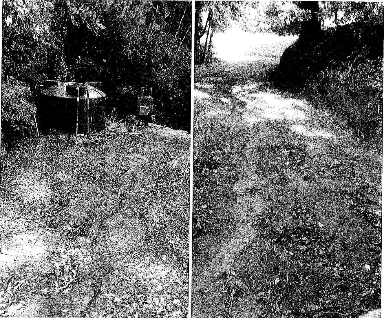
Pictures 1 and 2: These are the pictures taken along the segment of Map Point 2 prior to the recent rock lining of the inside ditch. The picture on the left shows the south end of the road segment identified as Map Point 2 on the WRPP Map. The picture on the right is taken from south end of this road segment and is looking up the road in a northerly direction. The recent October rainfall has caused the runoff to overflow the inside ditch and over the fill at the end of the road. The Discharger had recently installed erosion control "Jute" Netting on the face of the road fill. Photo date 11/3/2016
