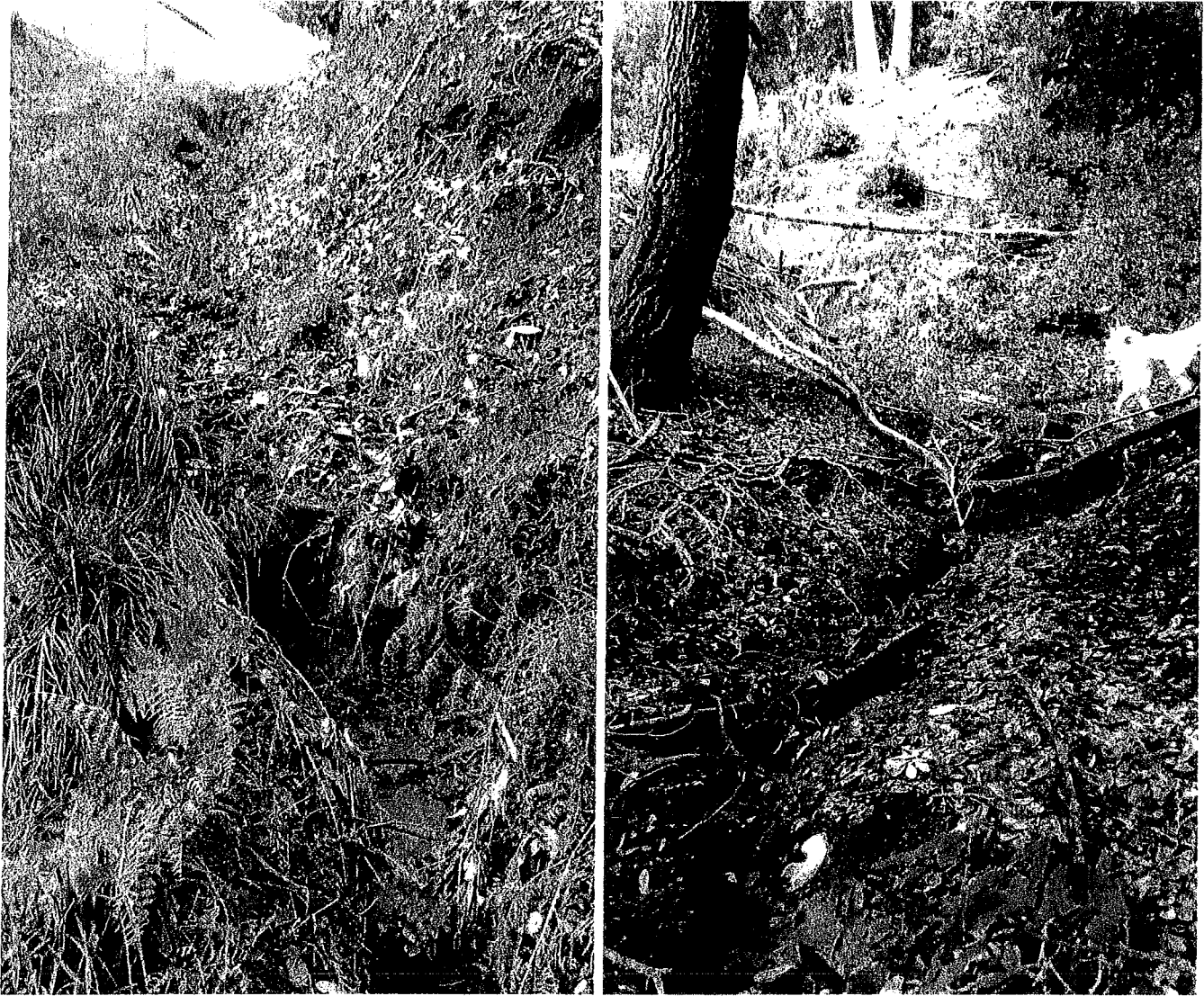
Pictures 13 and 14: These are pictures taken at the southeast of Map Point 6. It shows the eroded gully between the end of the road and the Class III watercourse. The dog in the picture on the right is pointing up the natural Class III watercourse. Photo date 12/2/2016
