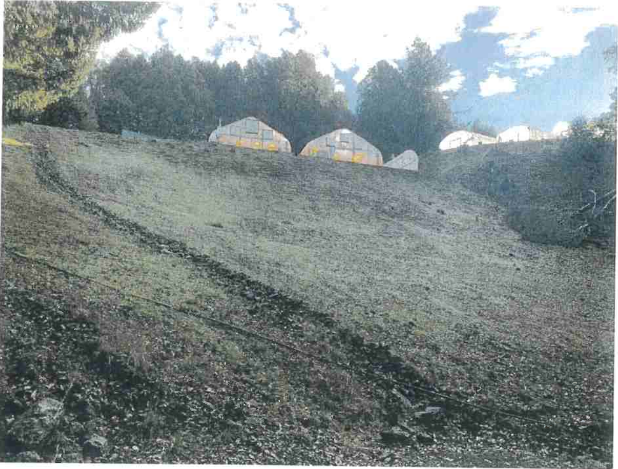
Photo 3: Site B center and Site A distant left. Note rocky V-ditch constructed to accommodate storm-water runoff from the graded flat. Photo date 1-17-2022.
