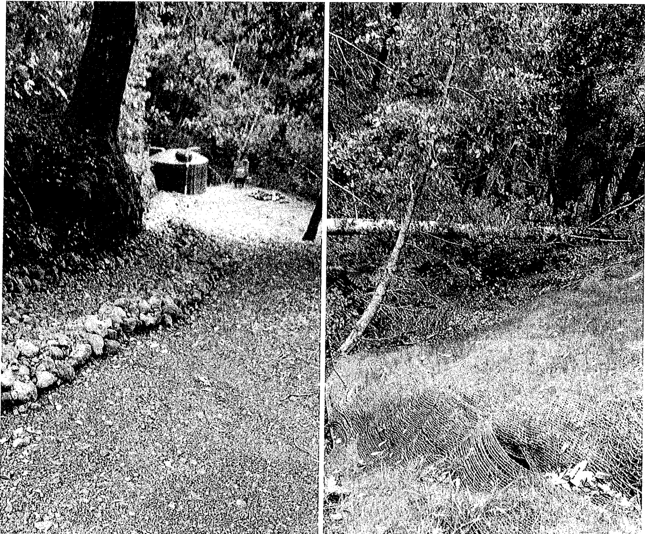
Pictures 8 and 9: The picture on the left shows recently widened and rock lined ditch. A rolling dip shall be installed just prior to the end of the road, to drain the road surface and the ditch towards the right so that it no longer can drain over the fill slope straight off of the end of the road. The picture on the right shows the grassed over jute netting placed on the fills beyond the end of the road. Photo date 2/13/2017
