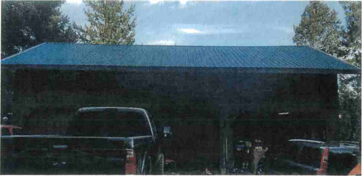
Photo 16: Garage near the main residence
