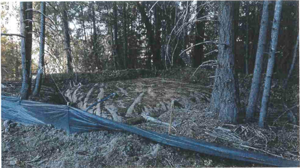
This is an example of a containment pit which will assist in mitigating the impacts if this storage bladder failed.
