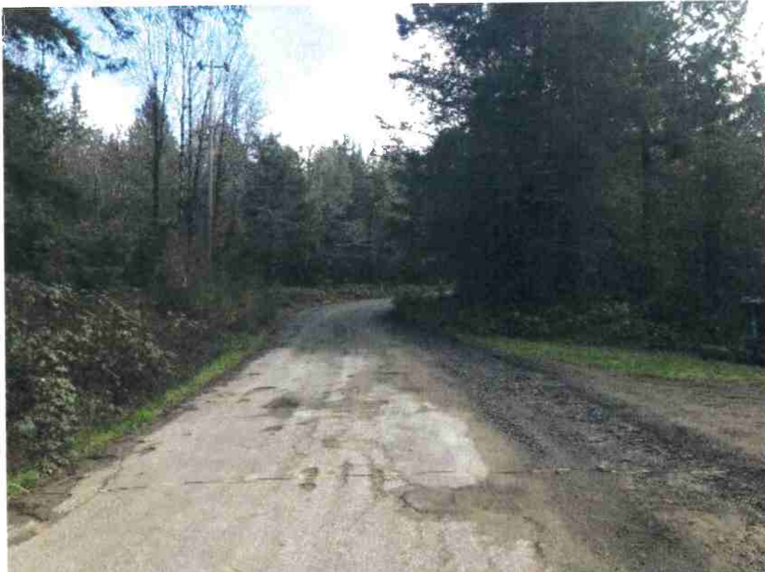
Photo #6-Approximate road width: 18 feet (does not include driveway)
