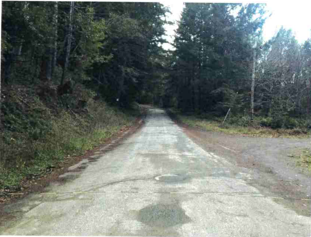
Photo #8-Approximate road width: 18 feet (does not include driveway)
