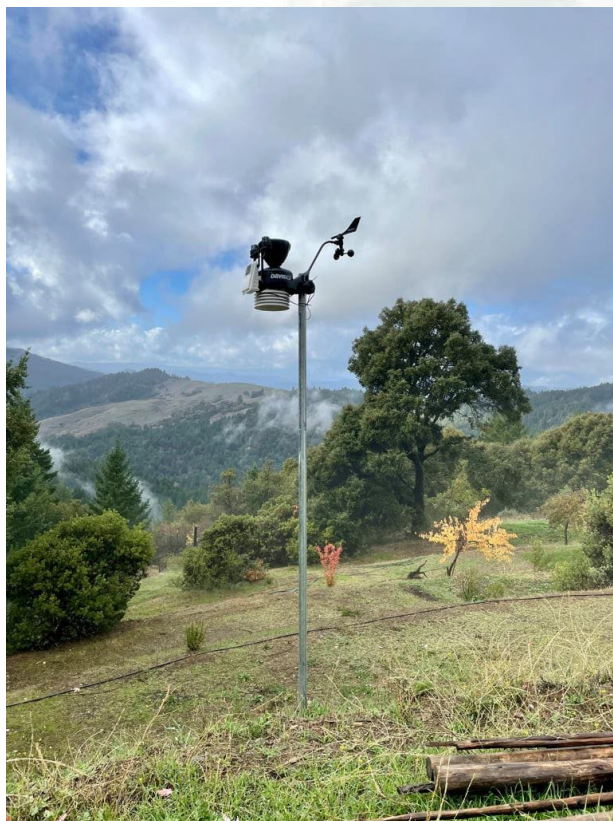
Installed Weather Station
