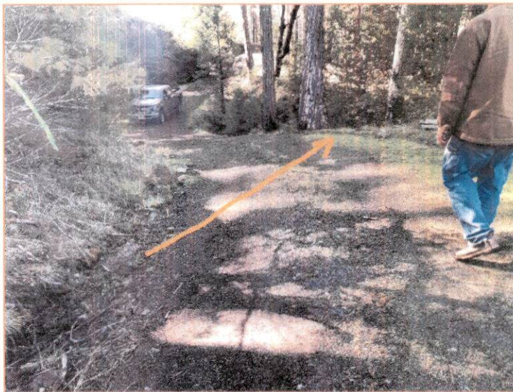
RP8) Install rocked rolling dip or replace failing DRC.
