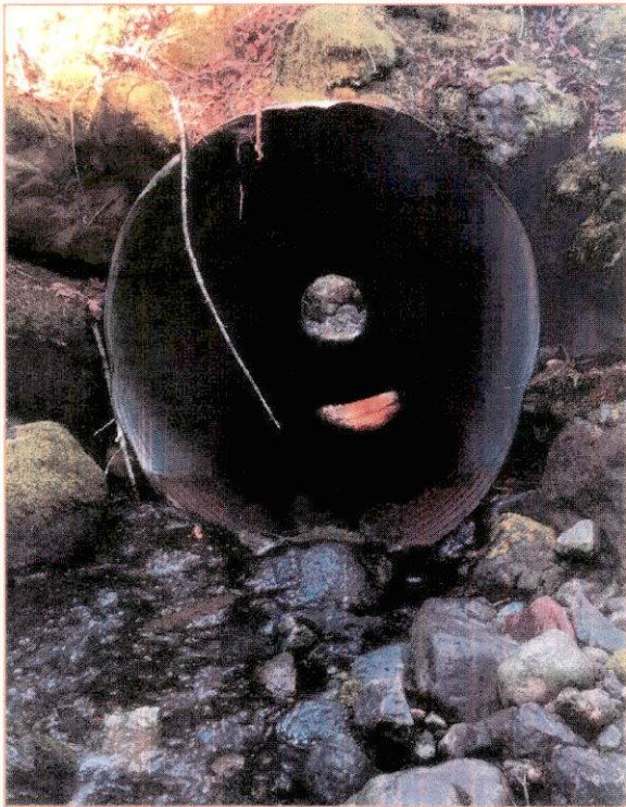
RP7) View of inlet on a class II stream.
