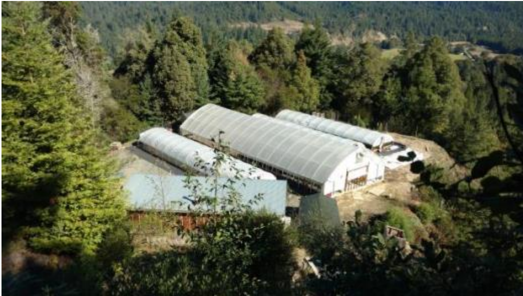
Figure 1. Site A looking northeast.
