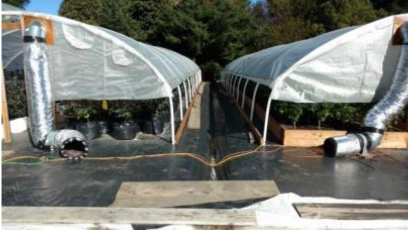
Figure 9. Drainage ditches on site A, ditches run from the south to the north edge.
