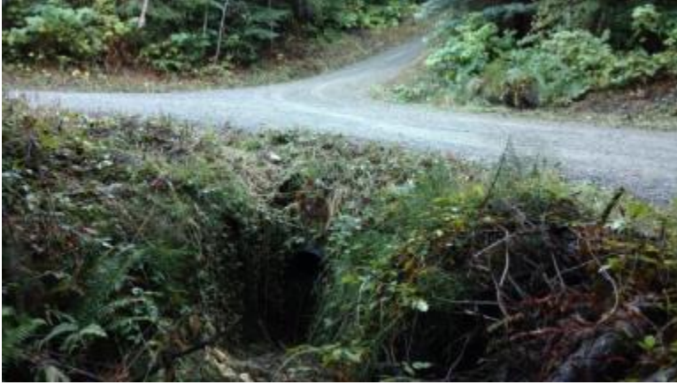
Figure 2. Road Point 2, photo taken below culvert outlet looking uphill.
