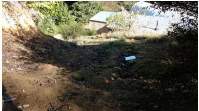
Figure 8. Road point 6, skid trail above site A.
