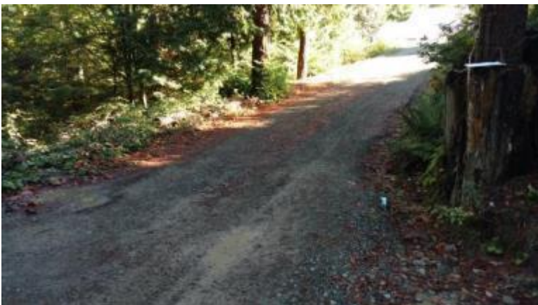
Figure 4. Road Point 3. looking north, culvert inlet to the right.
