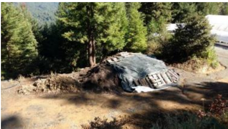
Figure 13. Road Point 9.2, Soil storage pile.
