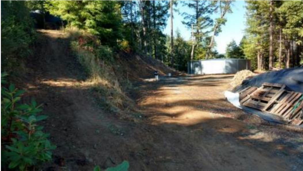
Figure 11. West arm of site B, looking west. Showing road point 9 (area needing rocked), and on the left road point 9.3 skid trail.
