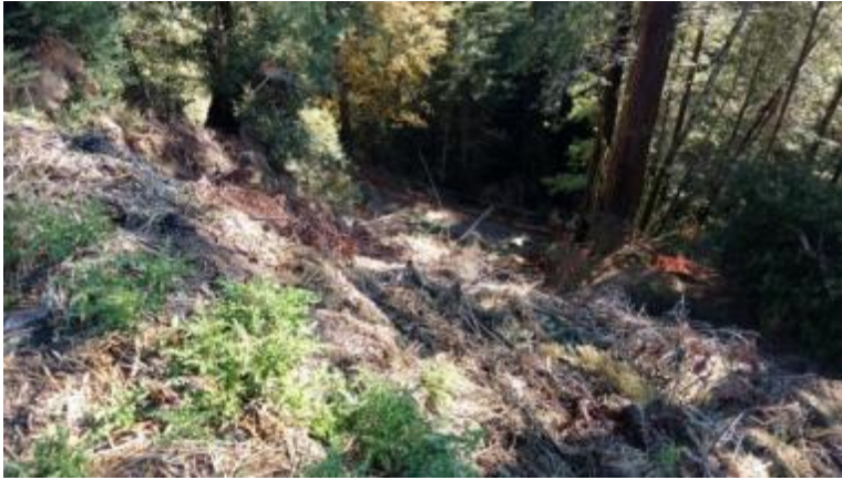
Figure 5. Road Point 5, at the top of the large slide looking downhill toward the county road.
