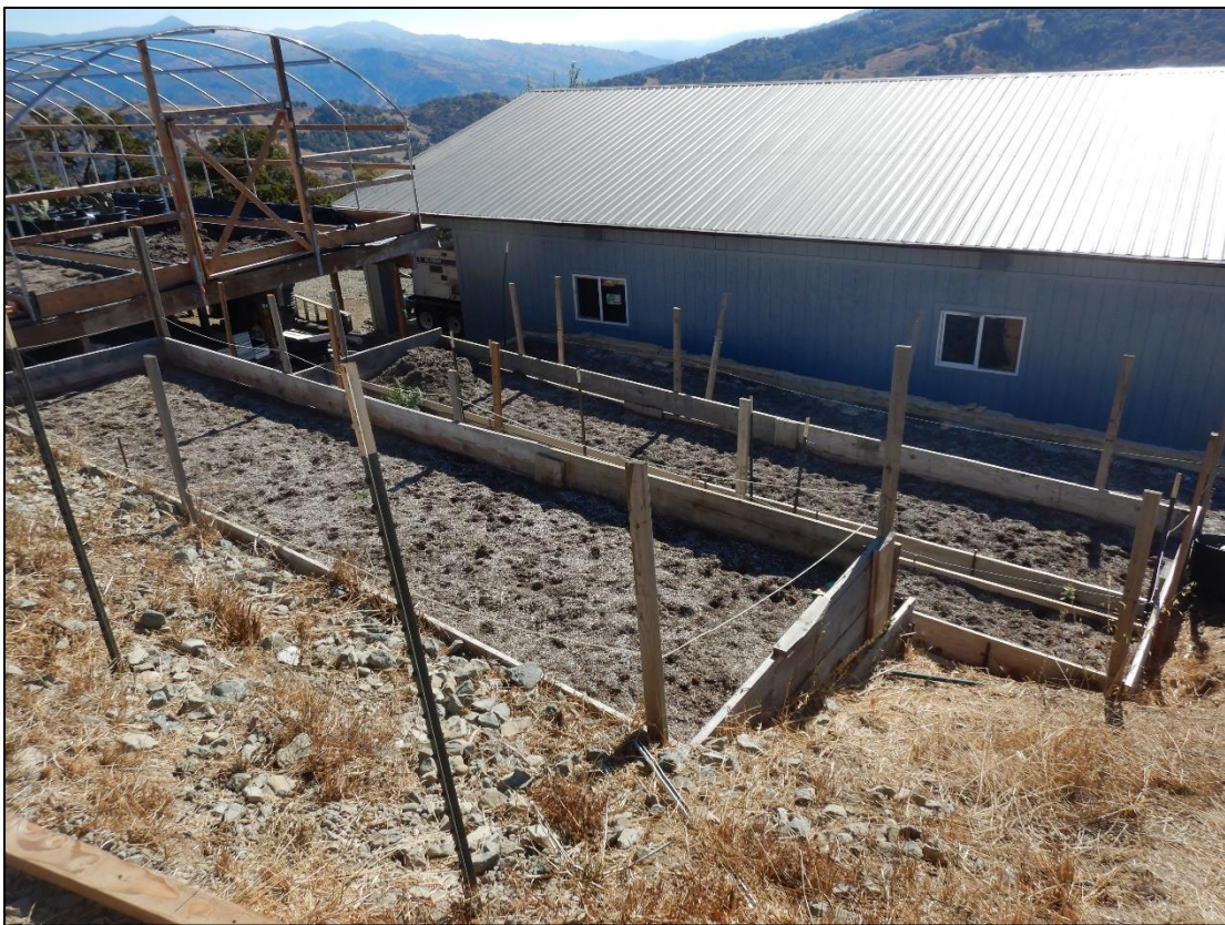
Photo 12. A portion of the Pre-Existing Cultivation Site which was measured to have a slope, prior to ground disturbance, of approximately 25% (Map 2).
