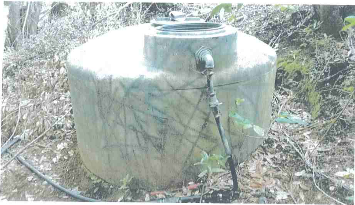
Picture 9: 550-gallon hard plastic water storage tank. Photo date 6-13-2017.
