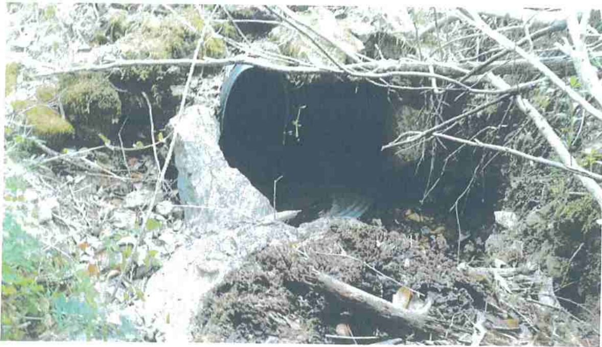
Picture 3: Crossing inlet. Photo date 6-13-2017.
