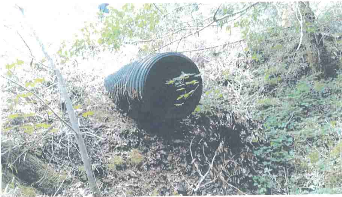
Picture 4: Crossing outlet. Photo date 6-13-2017.
