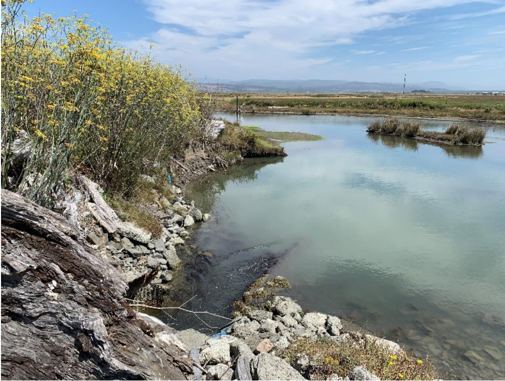
Photo 3. Inboard side of the tidegate.
