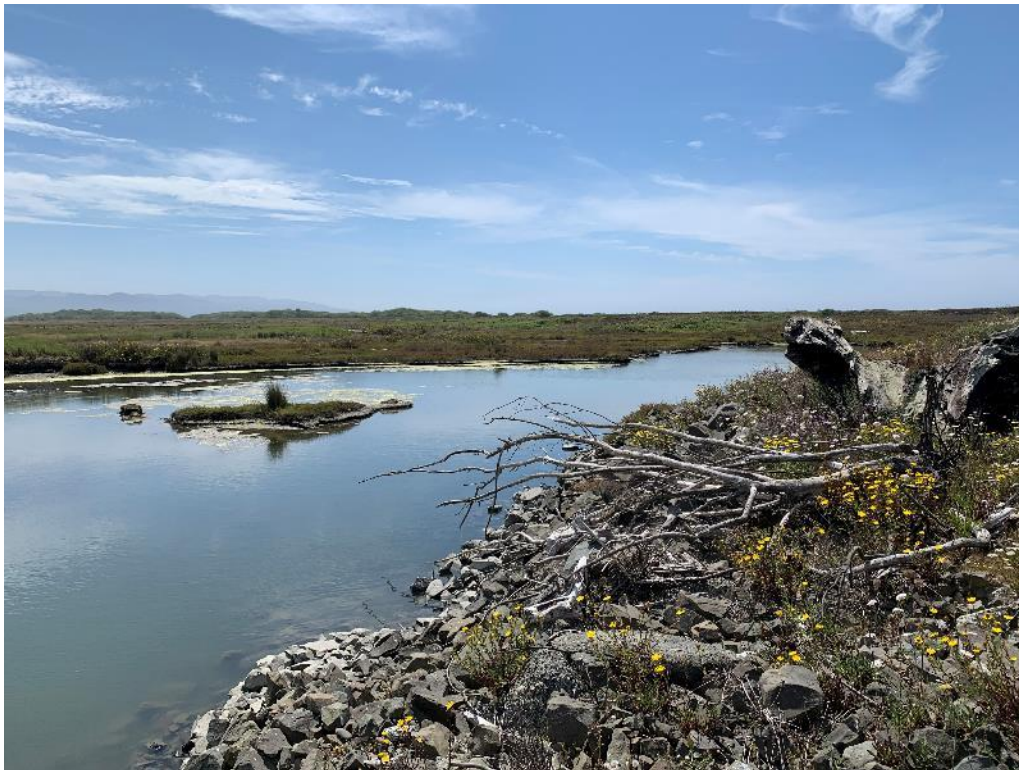
Photo 2. Rocked levees around the tide gate.
