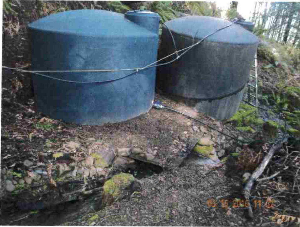
Figure 4. Two 3000-gallon storage tanks located at POD.
