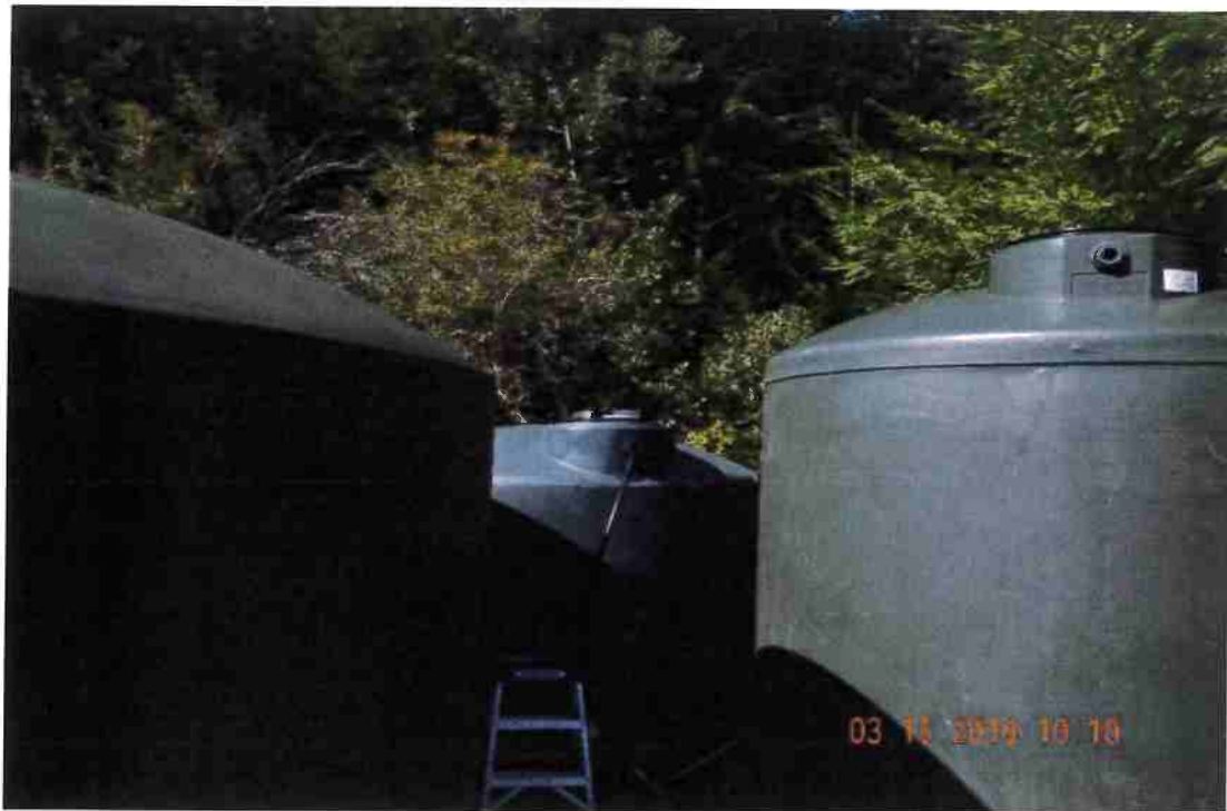
Figure 5. Storage tanks at cultivation site. At the time of field investigation, the site had 19,500 gallons of tank storage is planning on adding 100,000 gallons in tank storage.
