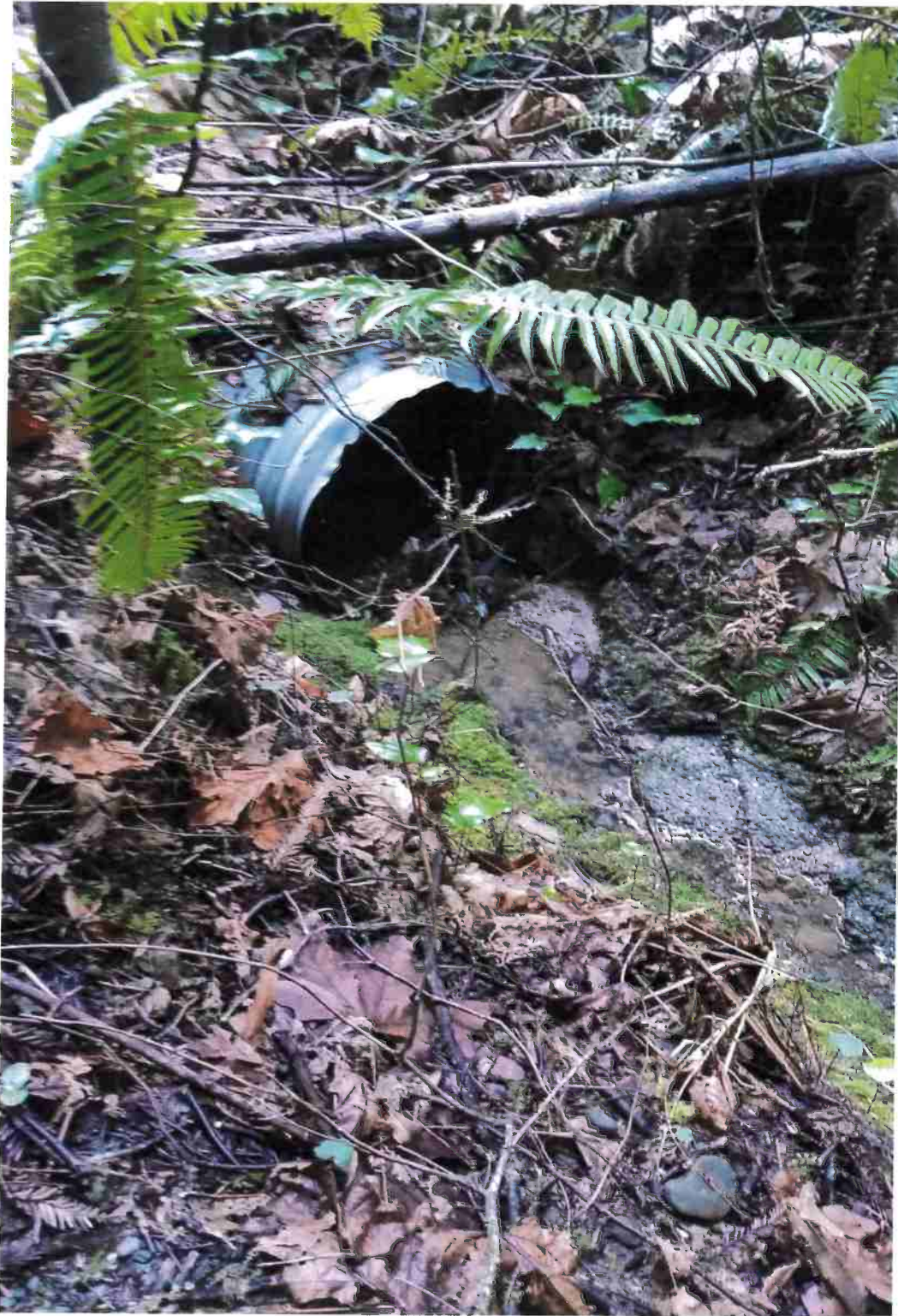
Figure 10. Inlet at 18" CMP at STX-2. Culvert will be replaced with a 24" diameter pipe.
