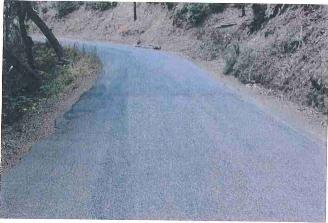
Photo 21. Mile 2.0: 15-ft road width with 1-ft shoulders.
