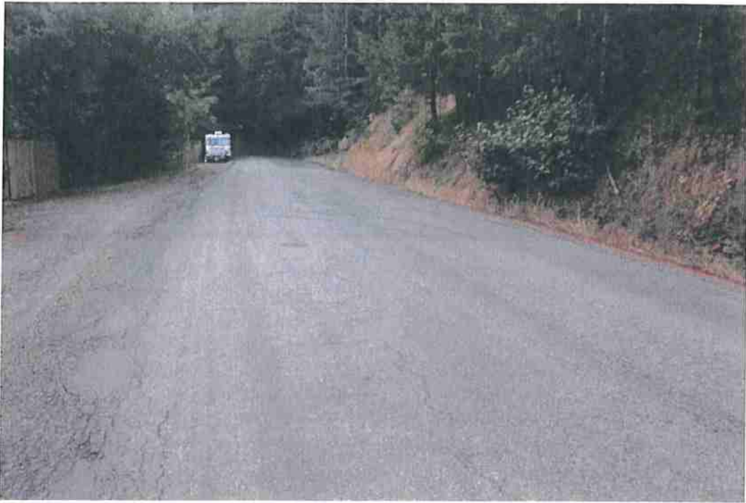
Photo 13. Mile 1.6: 24' width, 2' shoulders.
