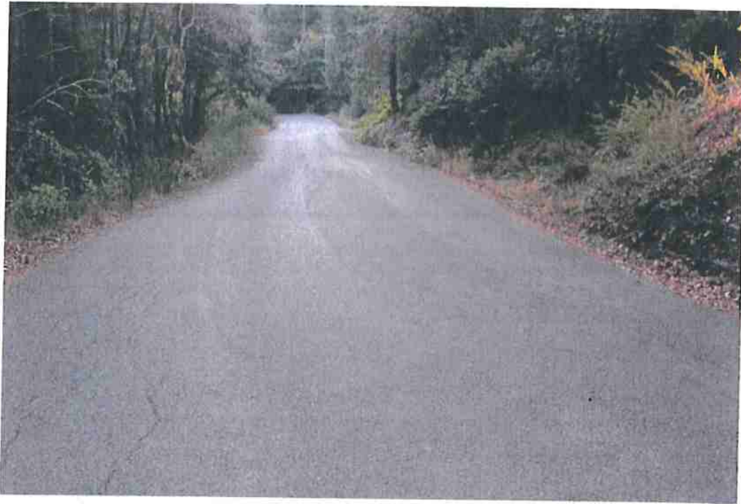
Photo 15. Mile 1.4: 22-ft road width with 1-ft shoulders.
