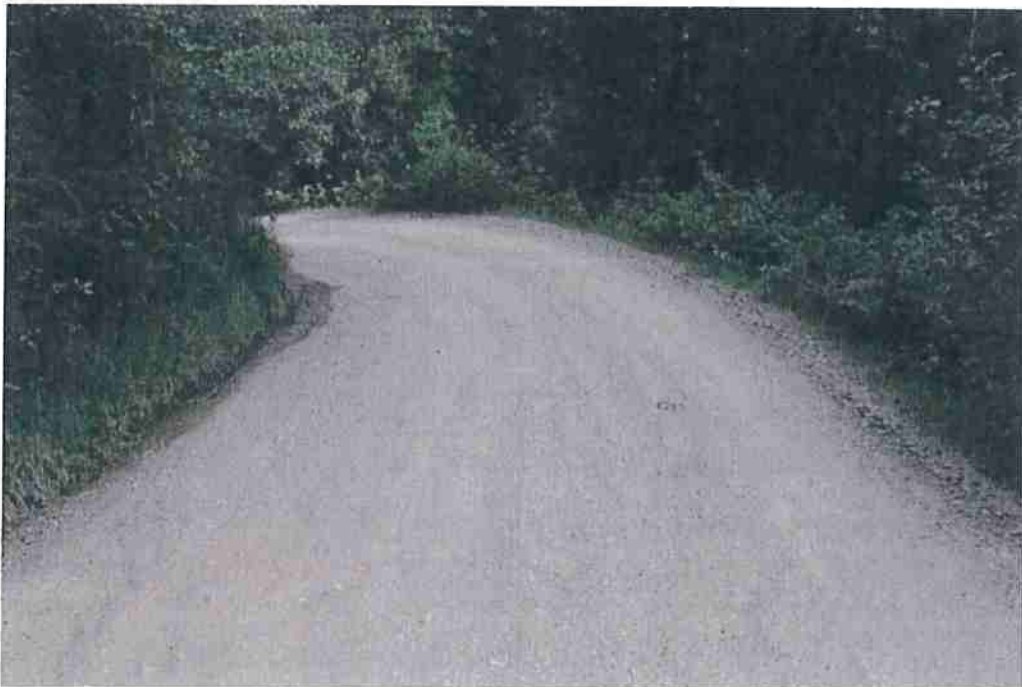
Photo 10. Mile 0.7: 16' width, 1' shoulders at blind corner, road is traversing steep area so difficult to widen.
