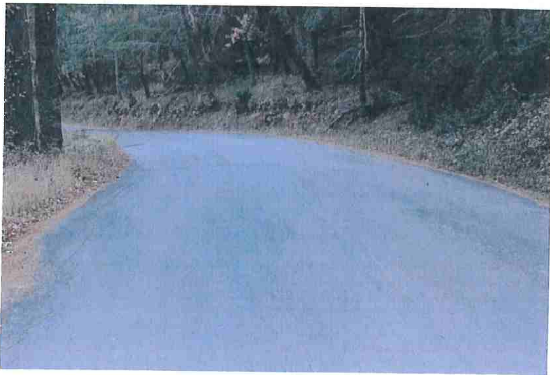
Photo 12. Mile 1.1: 20-ft road width with 2-ft shoulders.
