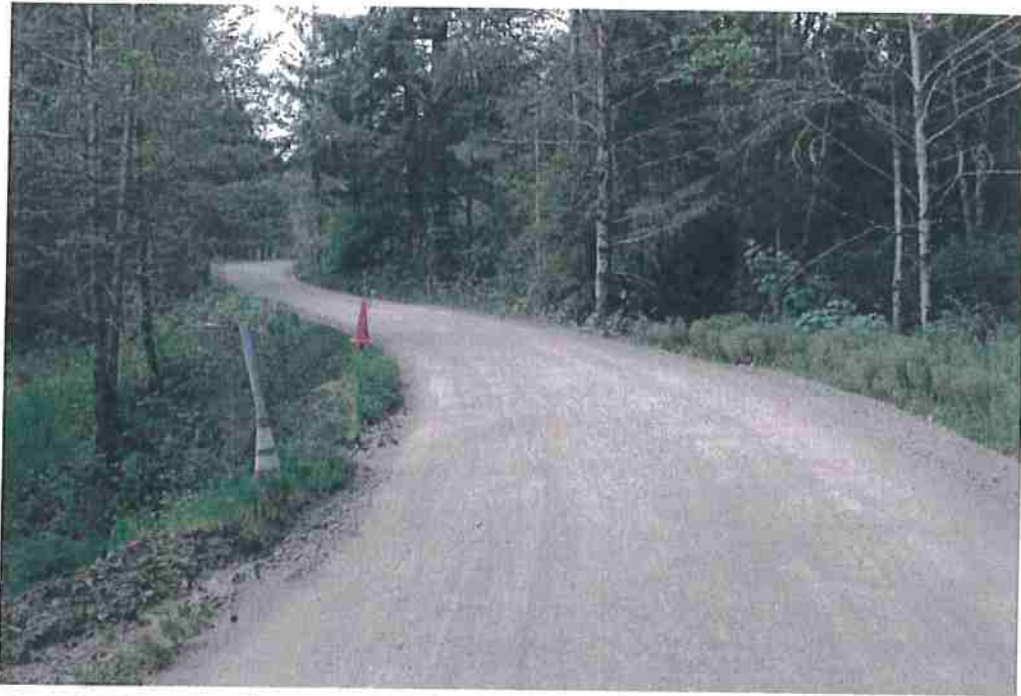
Photo 5. Mile 0.32: 16' width, no shoulders at pinch point at culvert crossing; good visibility and turnouts on both sides of crossing.
