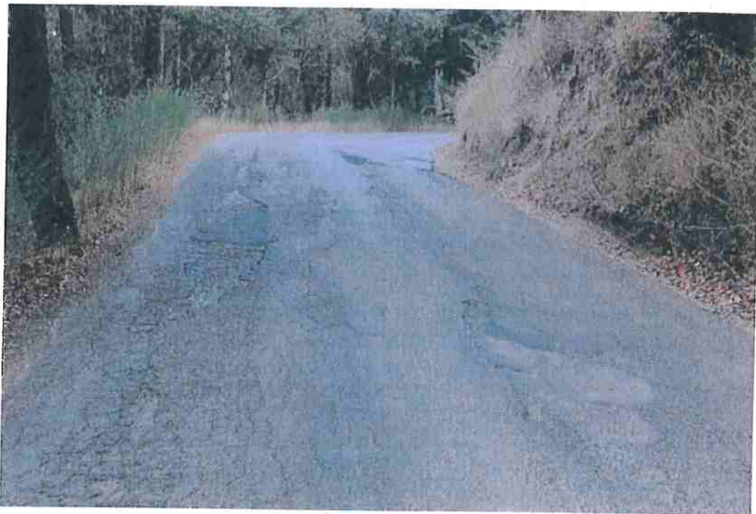
Photo 6. Mile 0.5: 18-ft road width with 1-ft shoulders.
