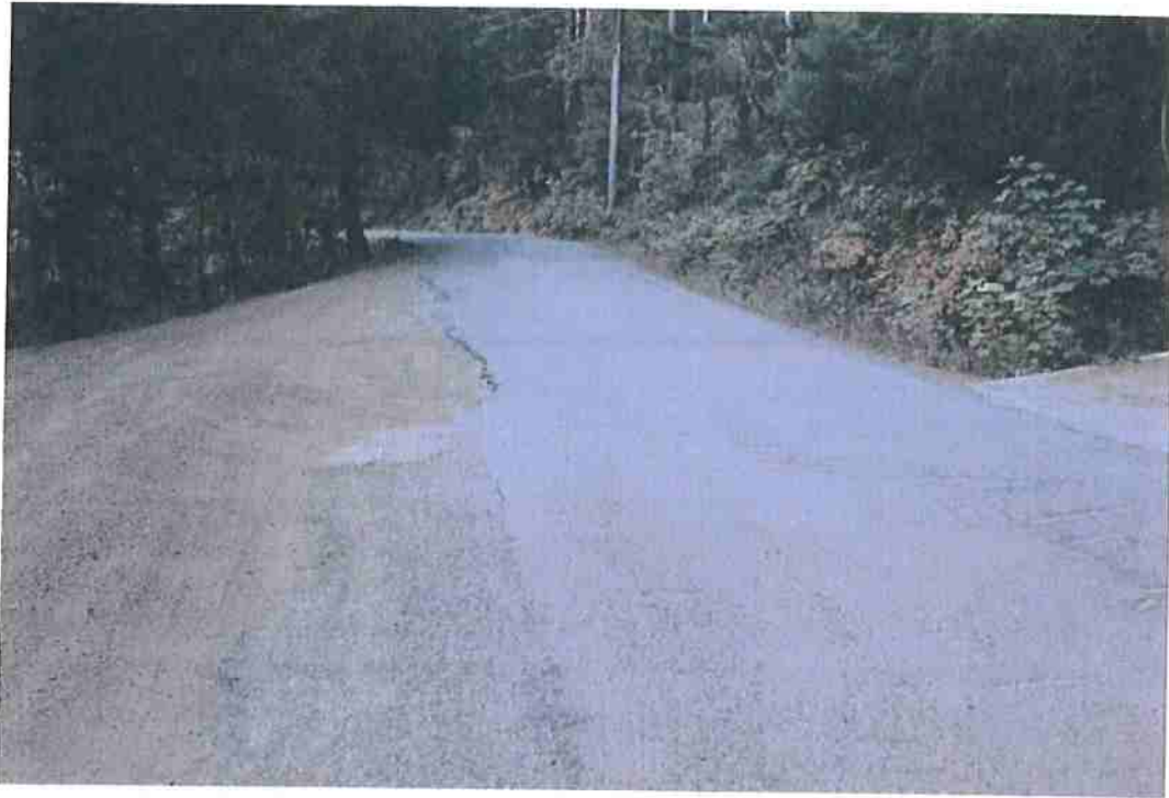
Photo 25. Mile 2.3: 20-ft road width with 2-ft shoulders.
