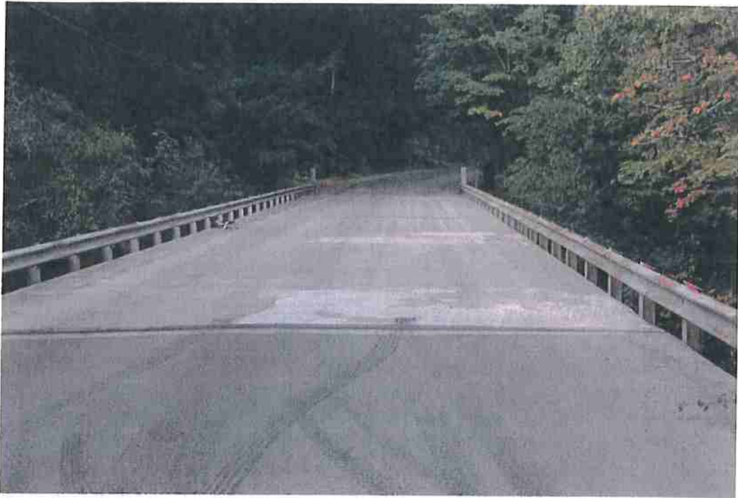
Photo 11. Mile 1.45: 28' width bridge, no shoulders.
