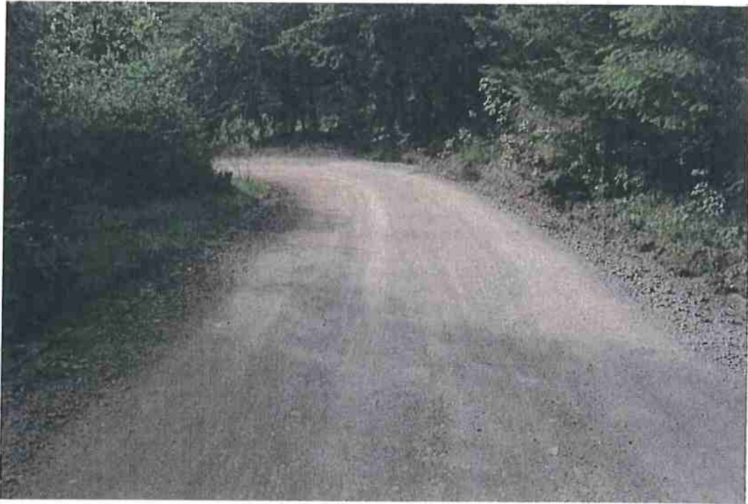
Photo 7. Mile 0.5: 18' width, 1' shoulders.
