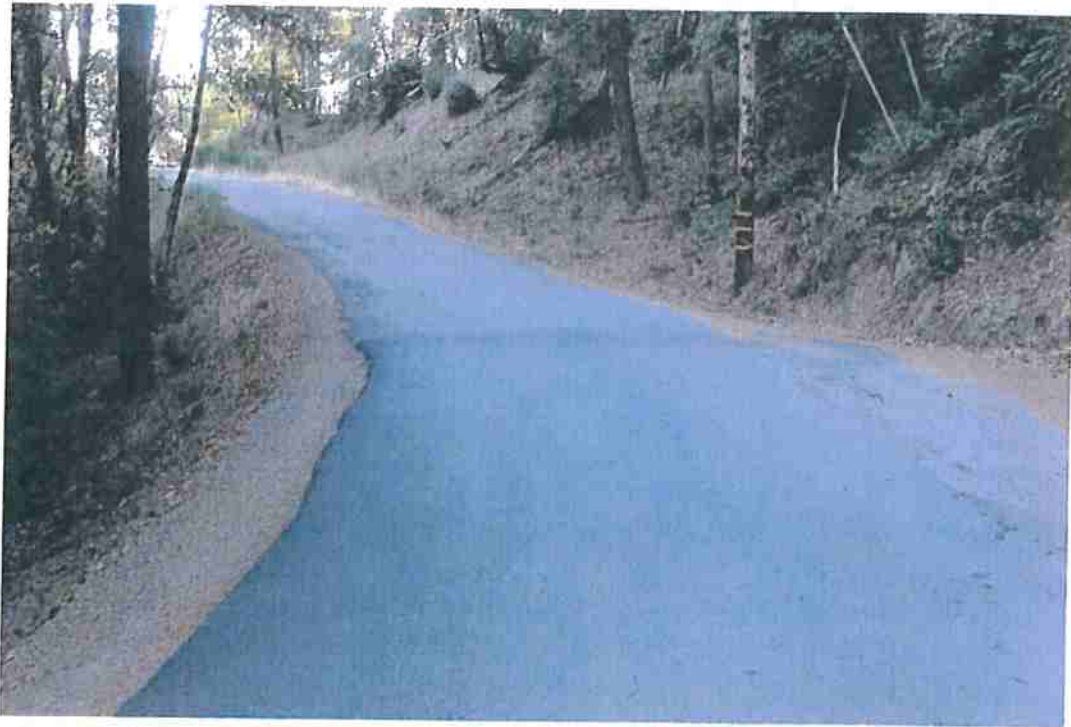
Photo 29. Mile 2.5: 18-ft road width with 2-ft shoulders.
