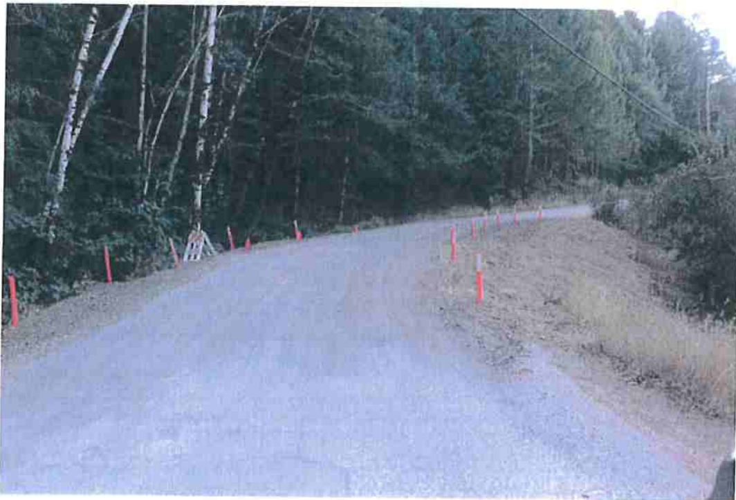
Photo 30. Mile 12.6: Recent culver repair, short gravel segment. 18-ft road width with 2-ft shoulders.
