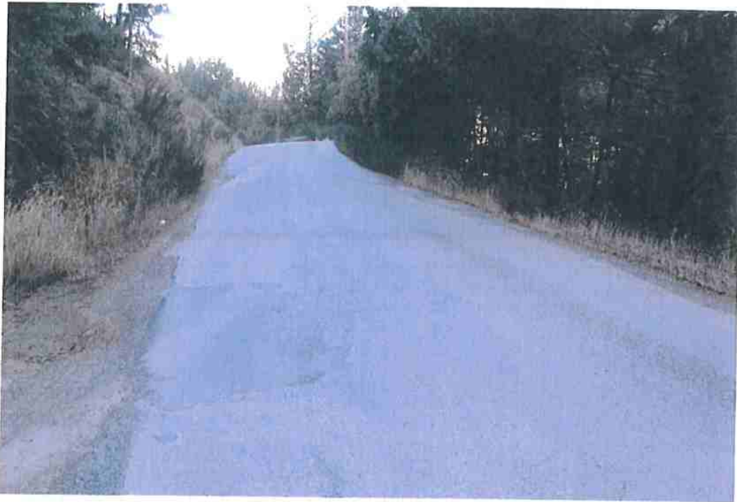
Photo 31. Mile 2.7: 20-ft road width with 2-ft shoulders.
