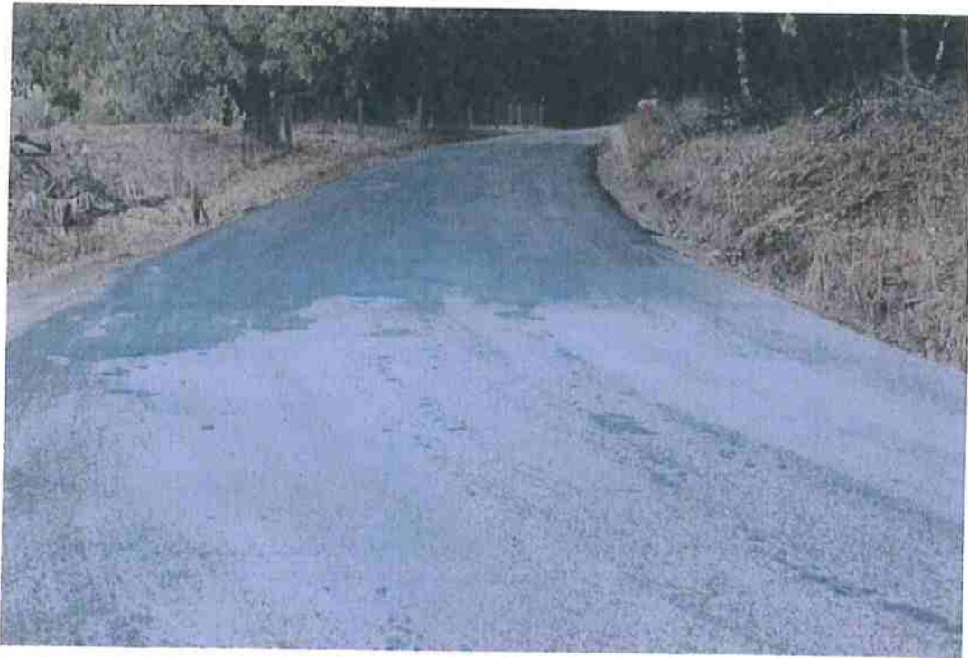
Photo 9. Mile 0.8: 30-ft road width with 1-ft shoulders.
