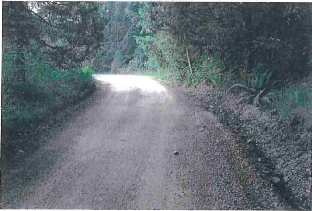
Photo 9. Mile 0.65: ~16' width pinch point with deep ditch.
