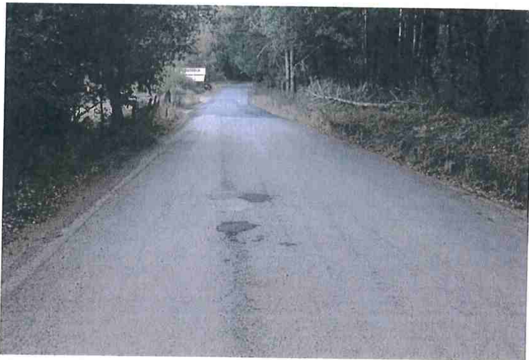
Photo 8. Mile 0.7: 20-ft road width with 2-ft shoulders.
