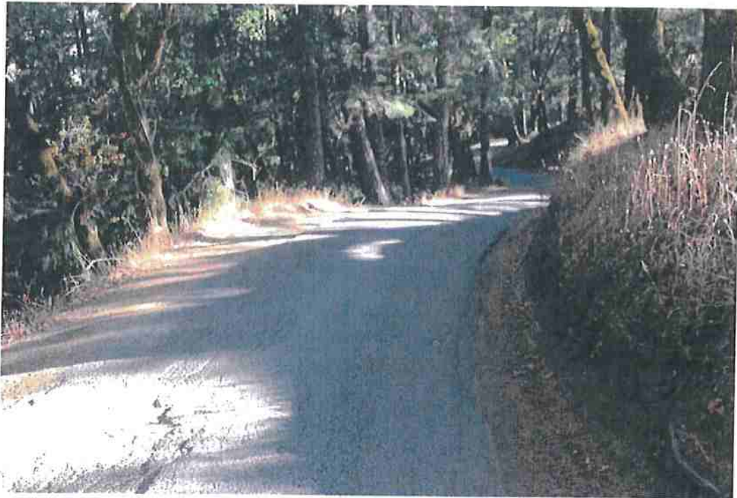
Photo 41. Mile 3.6: 12-ft road width with 2-ft shoulders. Pinch point but decent visibility with turnouts.
