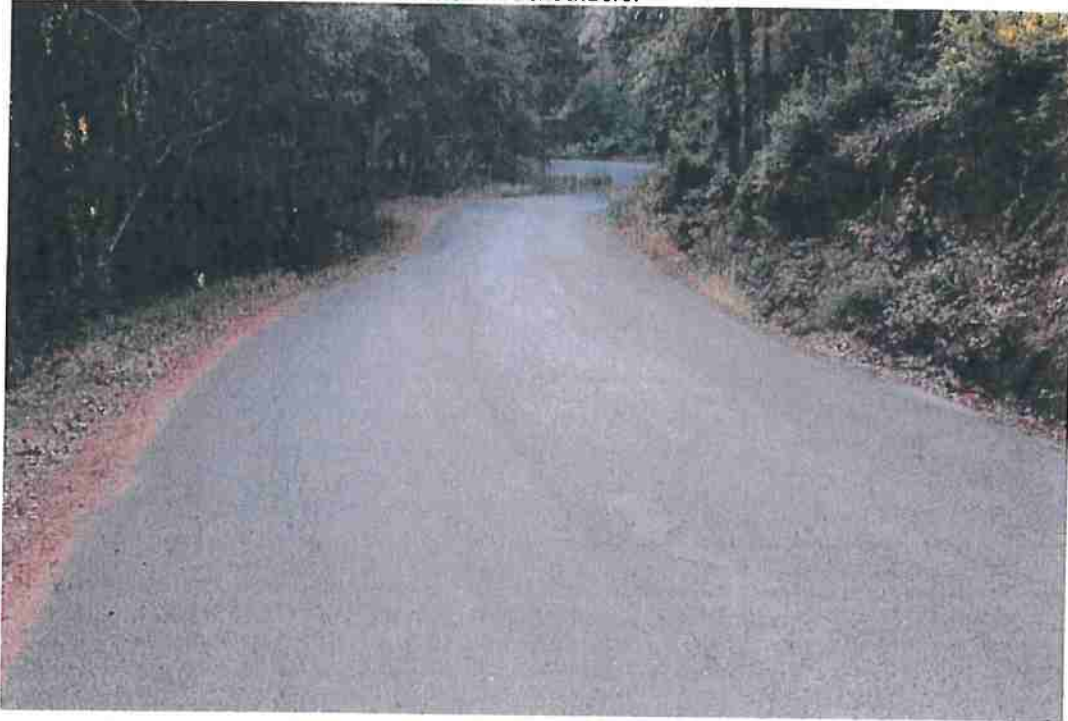
Photo 16. Mile 1.5: 20-ft road width with 1-ft shoulders.
