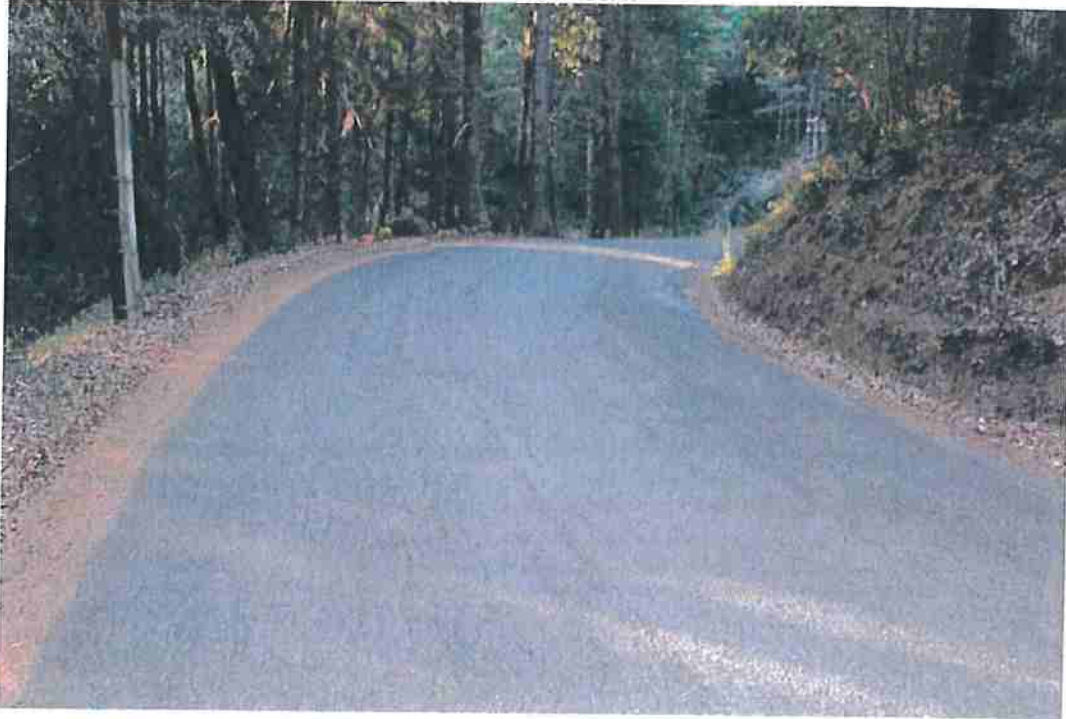
Photo 18. Mile 1.7: 20-ft road width with 1-ft shoulders.
