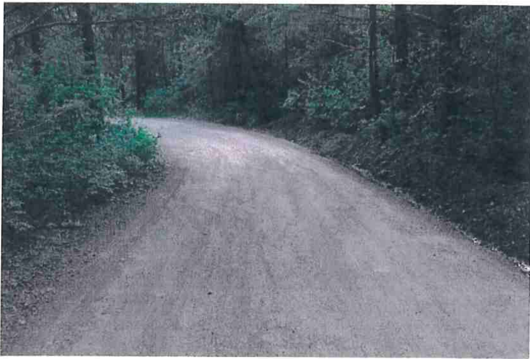
Photo 8. Mile 0.6: 18' width, 1' shoulders.
