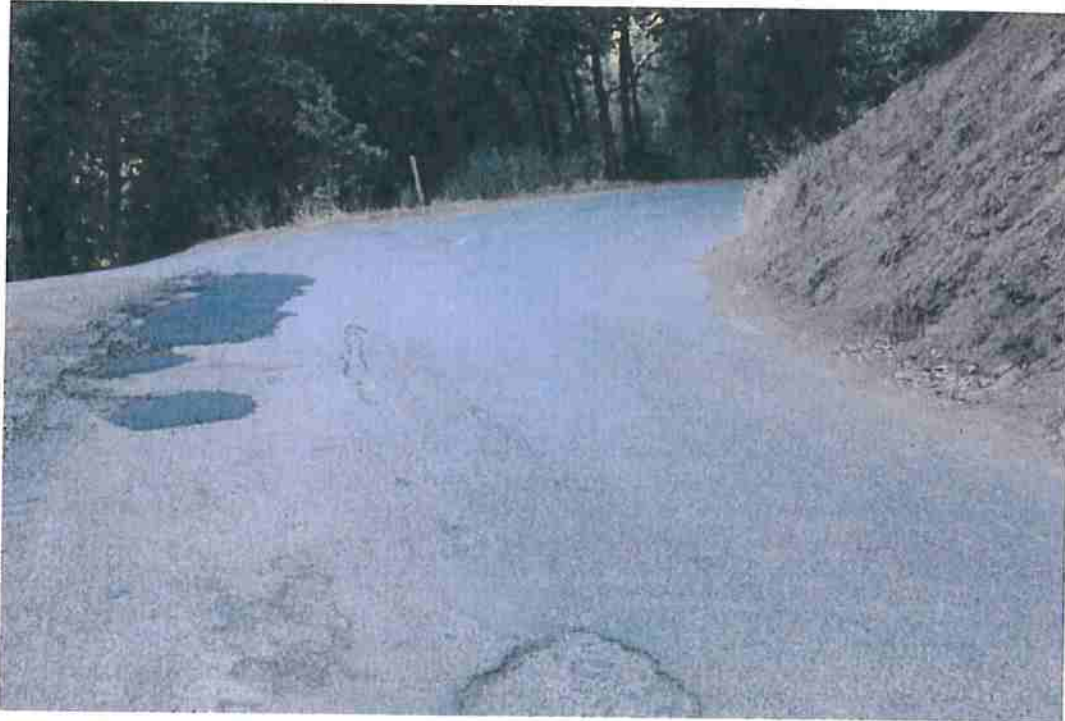
Photo 20. Mile 1.9: 18-ft road width with 2-ft shoulders.
