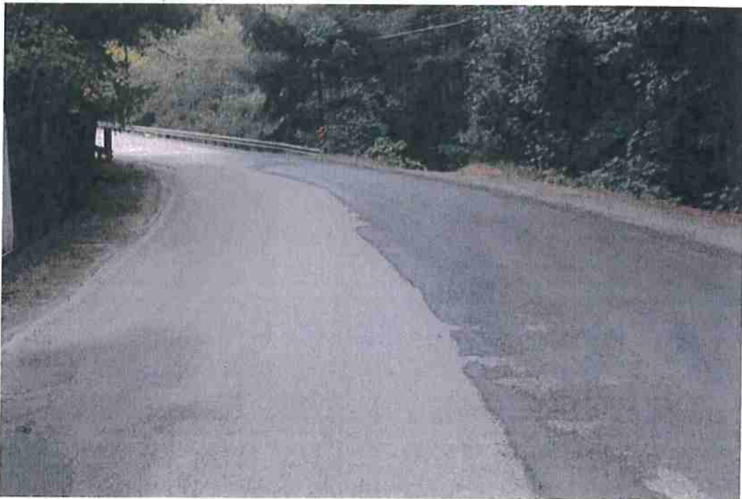
Photo 12. Mile 1.5: 24' width, 2' shoulders.
