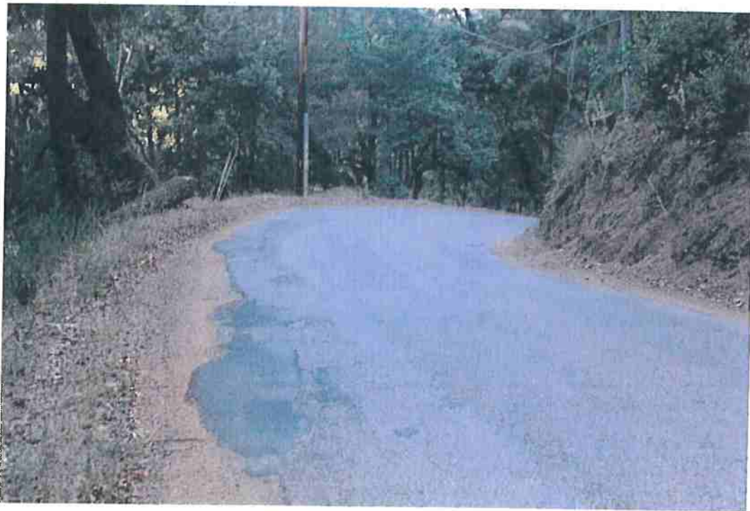
Photo 24. Mile 2.2: 20-ft road width with 1-ft shoulders.
