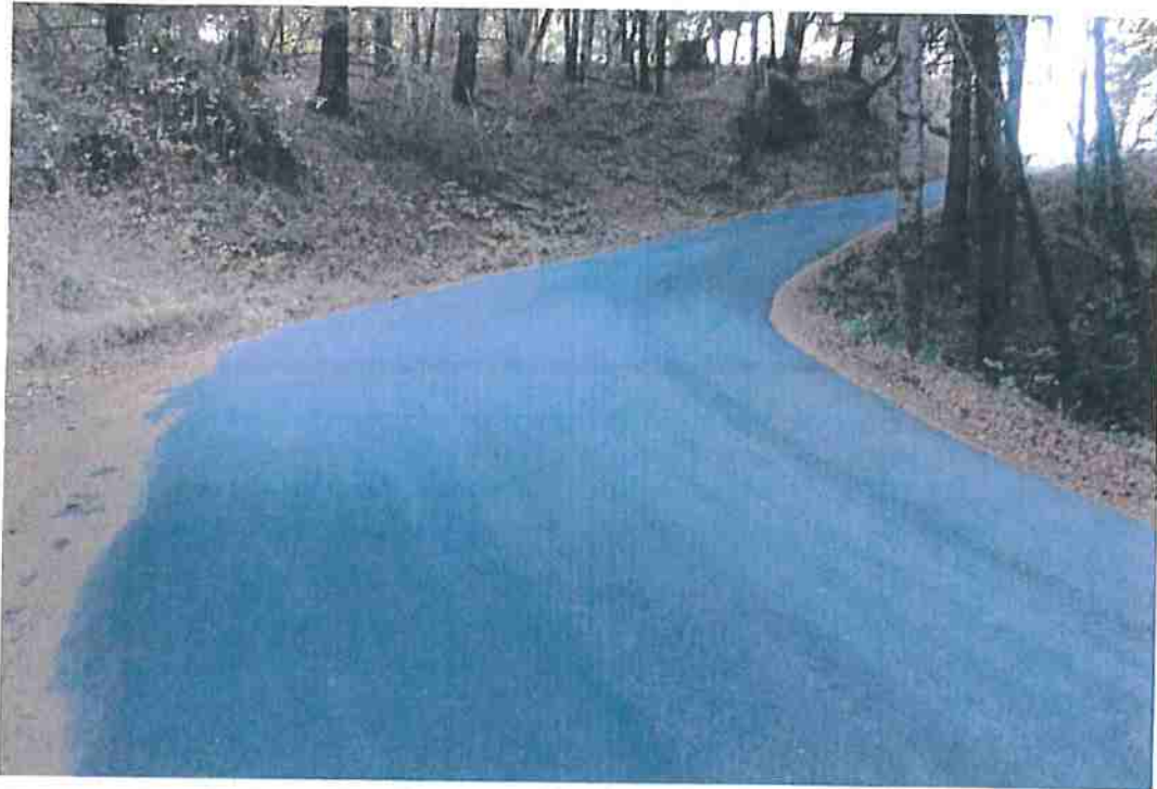
Photo 37. Mile 3.2: 20-ft road width with 2-ft shoulders.
