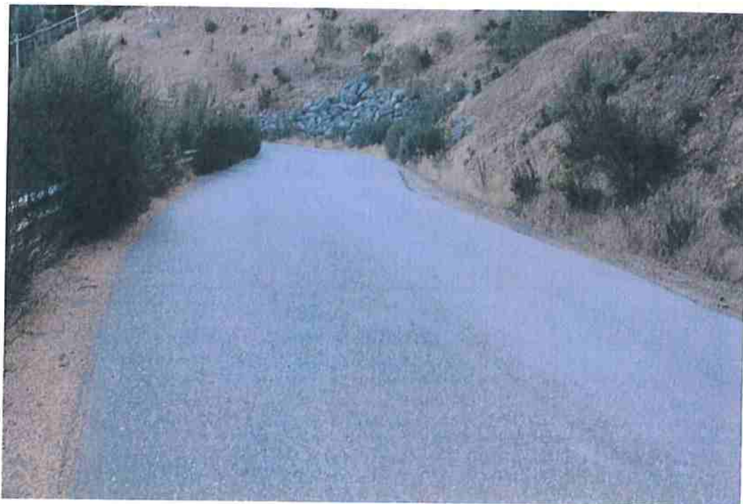
Photo 32. Mile 2.8: 18-ft road width with 1-ft shoulders.
