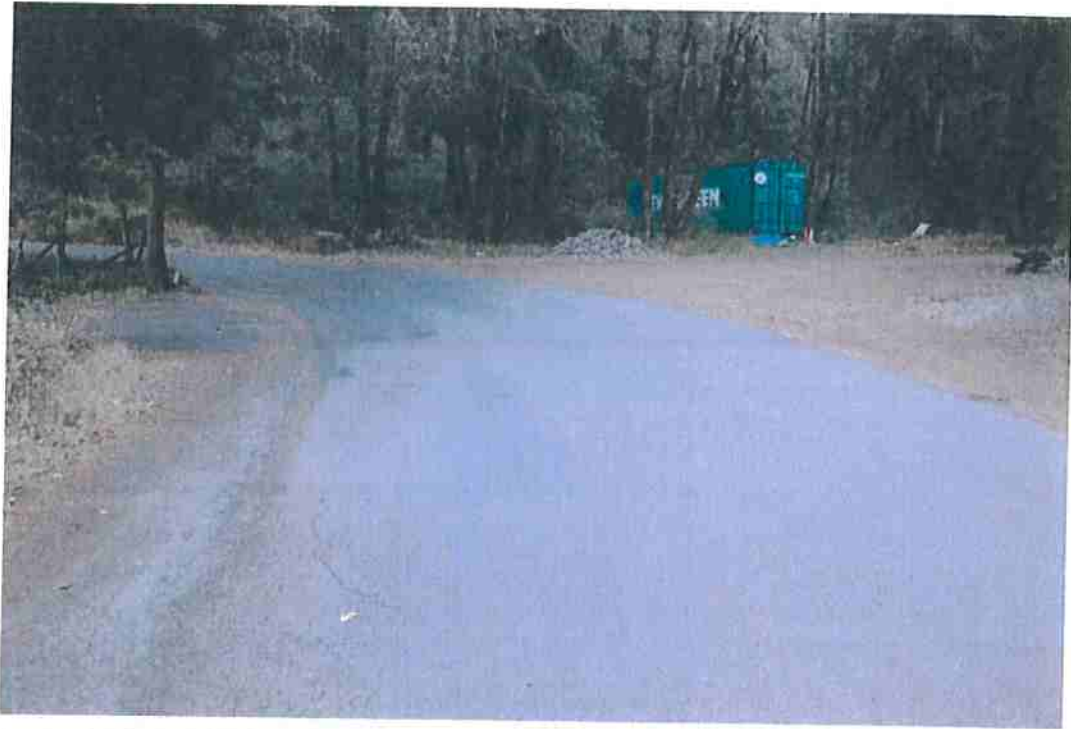
Photo 7. Mile 0.6: 24-ft road width with 2-ft shoulders.
