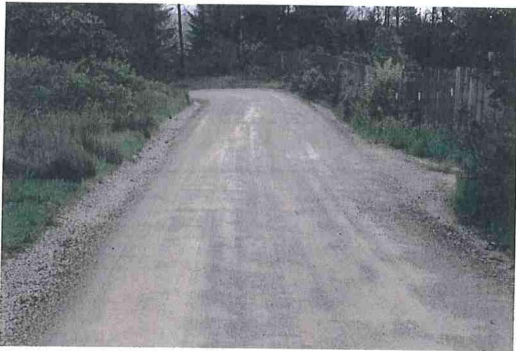
Photo 3. Mile 0.2: 18' width, 1' shoulders.
