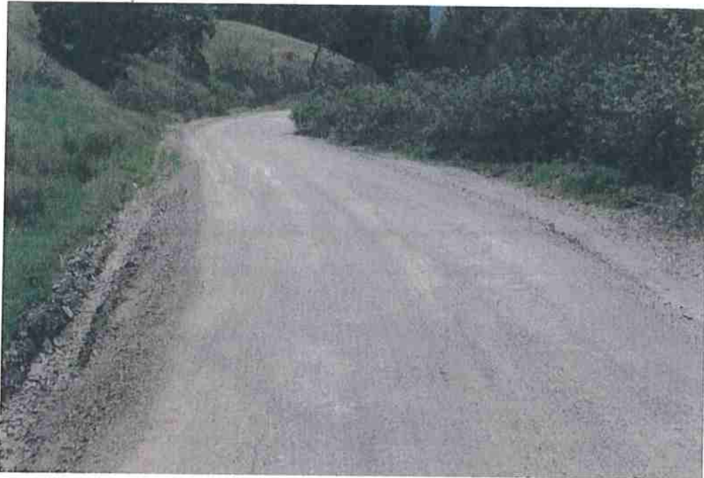
Photo 1. Mile 0.1: 16' width, 1' shoulders; road crosses geologically unstable area with some wider turnouts and brush impairing visibility.
