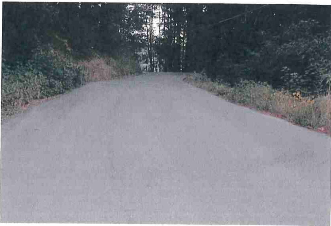
Photo 8. Mile 1.2: 24' width, 1' shoulders.
