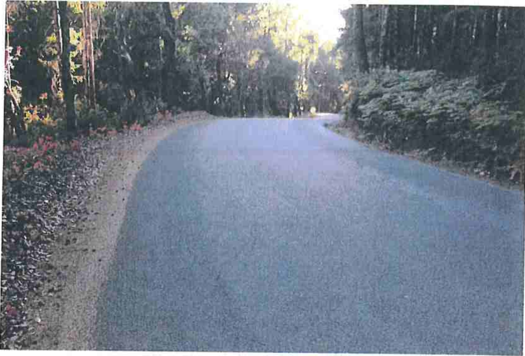
Photo 17. Mile 1.6: 20-ft road width with 2-ft shoulders.
