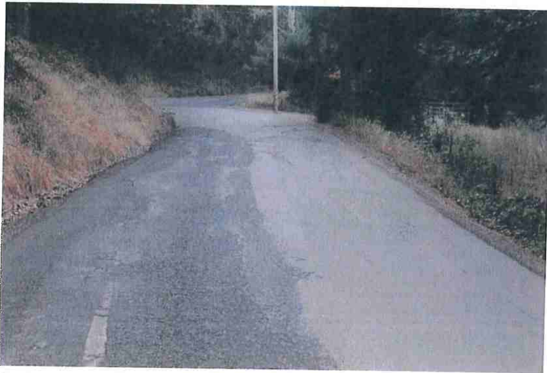
Photo 6. Mile 1.1: 20' width, 1' shoulders.
