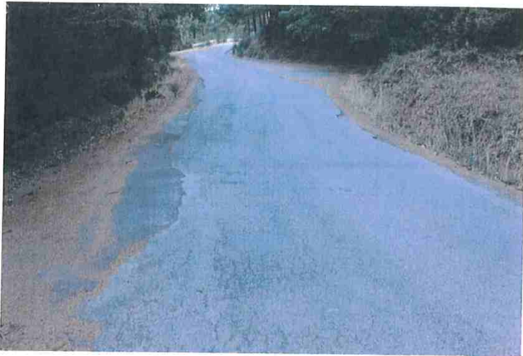
Photo 33. Mile 2.9: 18-ft road width with 1-ft shoulders.
