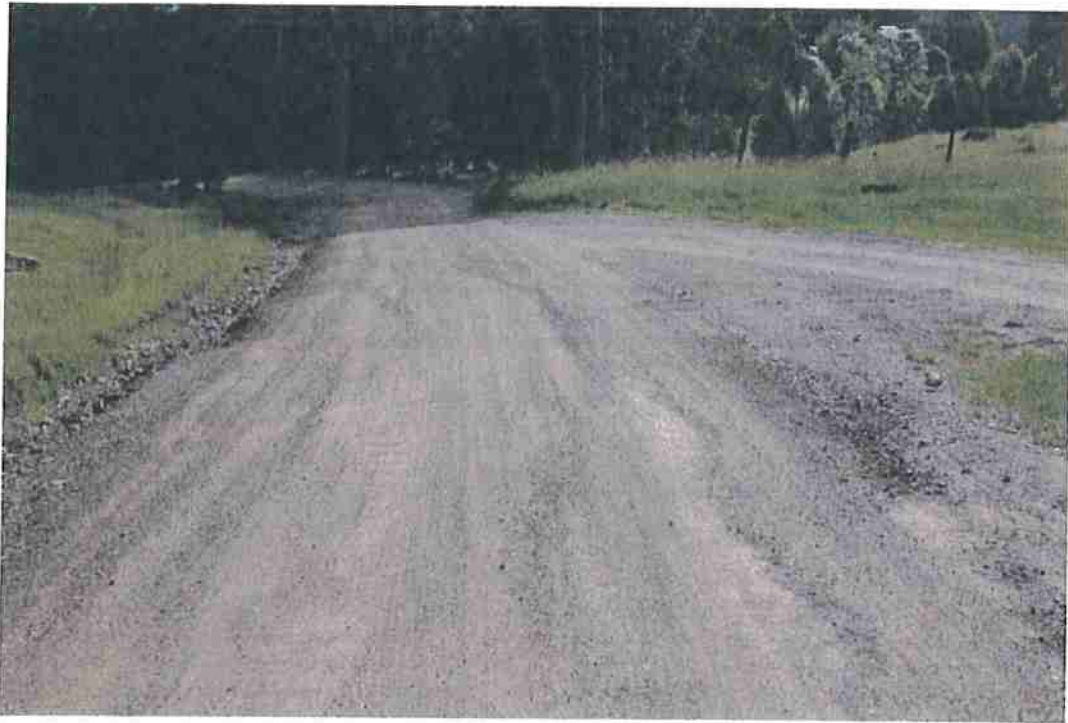
Photo 11. Mile 0.8: 18' width, 2' shoulders.
