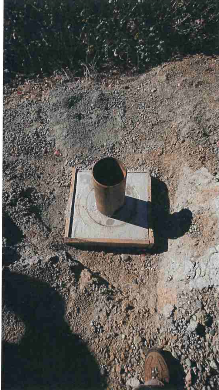
Picture 2: Recently drilled, permitted groundwater well which will be the sole source of water for the entire property. Photo date: 8/15/2019.
