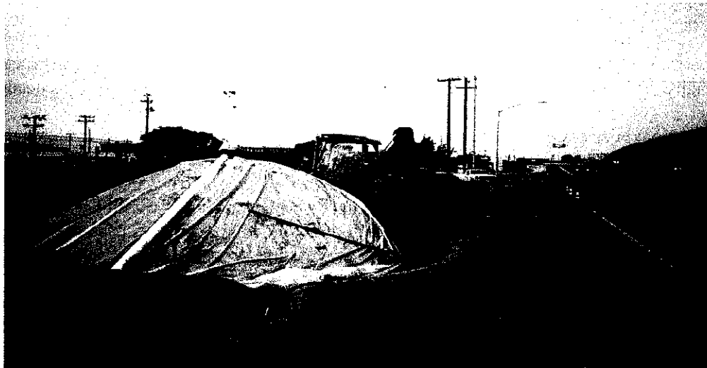
Figure 1. Stock piles should be covered with erosion and sediment control BMPs employed to keep sediment on site. From Caltrans (2003).
