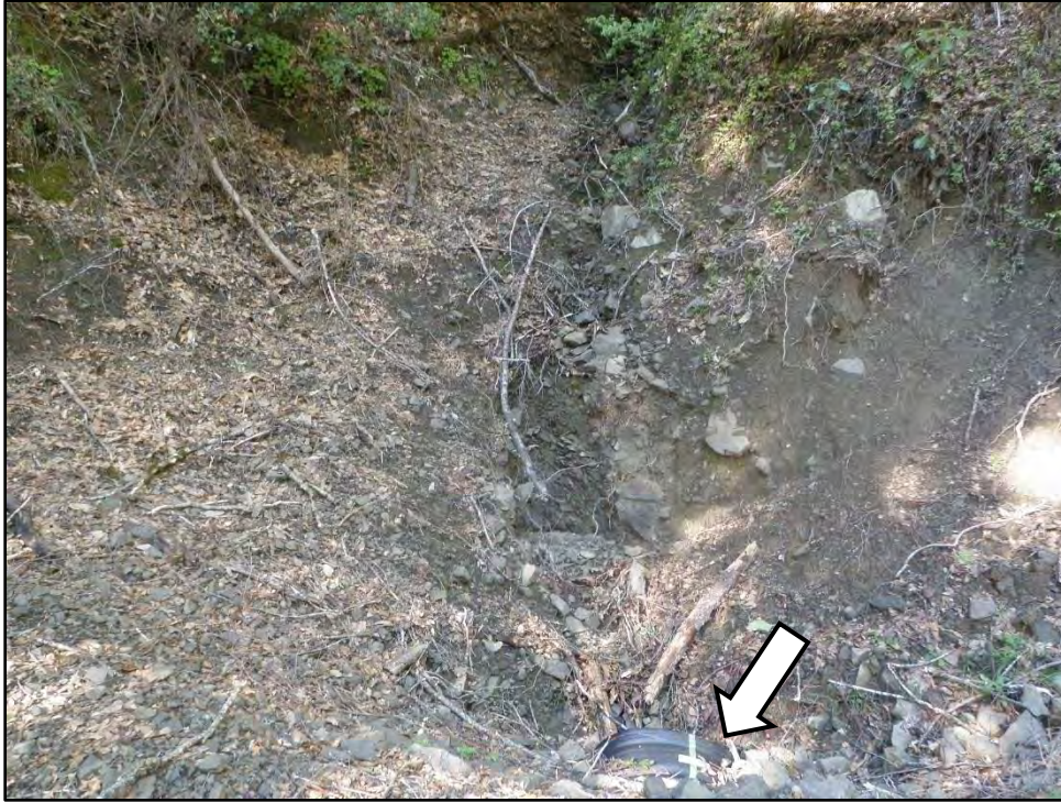
Photo 11 – Project #6, View looking upstream of SC #5 culvert inlet (arrow).
