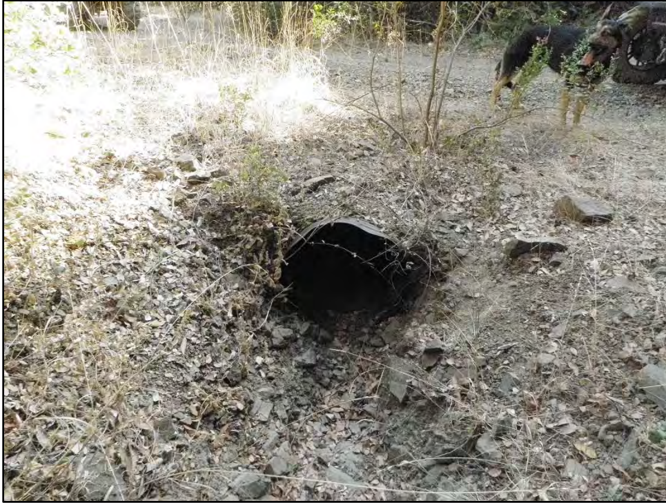
Photo 9 – Project #5, View looking downstream at SC #3 culvert inlet.
