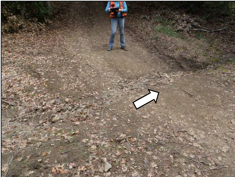
Photo 8 – Project #4, View of the fill crossing, SC #2B from the right road. Note the flow direction depicted by the arrow. This crossing is on a quad trail used seasonally by the applicant to get to House #2 from House #1.
