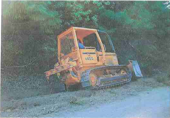
Figure 29. Bulldozer clearing out a road ditch. Photo: Jared Gerstein.
