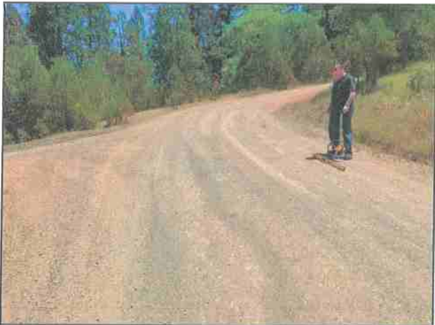
Photo #183 Thomas Rd @ Curve w/ Pullout Looking NE
