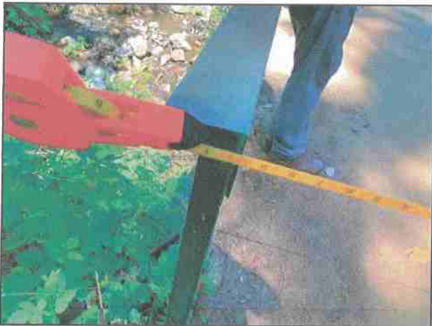
Photo #33 Private Access Rd APN 221-071-020 @ Bridge, Width 12'0"
