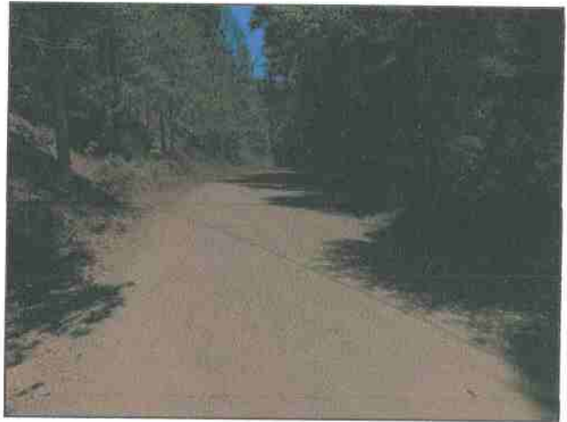
Photo #166 Thomas Rd @ Curve w/ Pullout Looking NE
