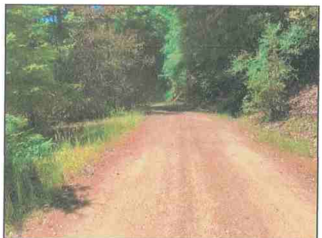
Photo #108 Private Access Rd APN 221-071-020 @ Curve w/ Pullout Looking SW
