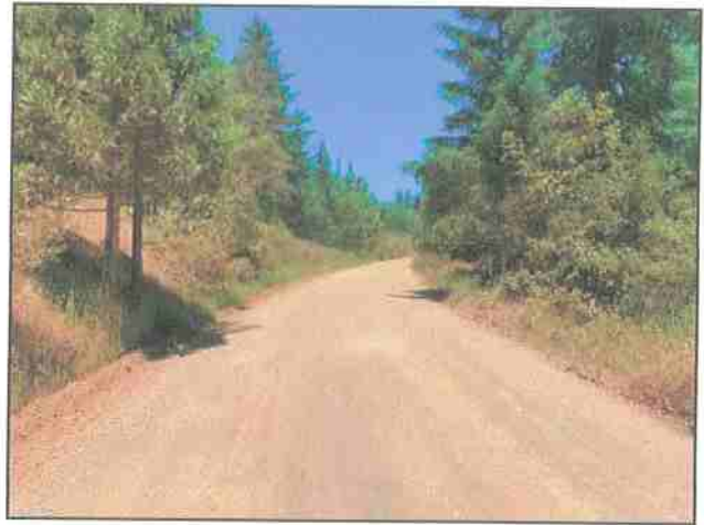
Photo #224 Thomas Rd @ Curve w/ Pullout Looking NE
