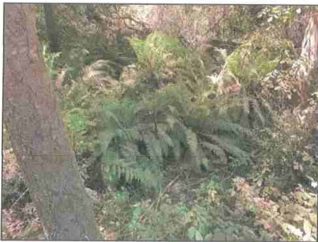
Photo #227 Thomas Rd Looking @ Clogged & Short Culvert In
