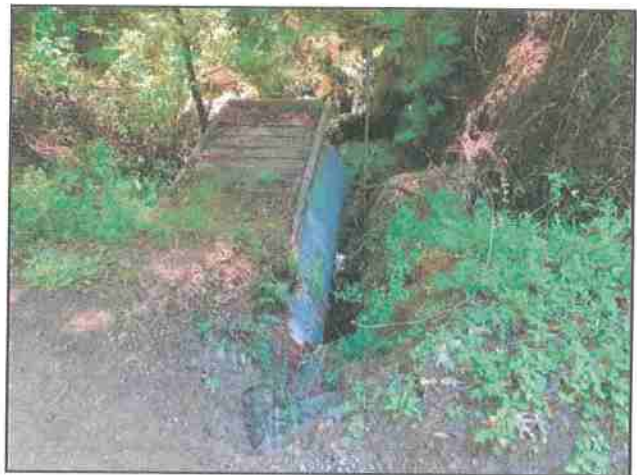
Photo #130 Salmon Creek Rd Looking @ Culvert Outlet
