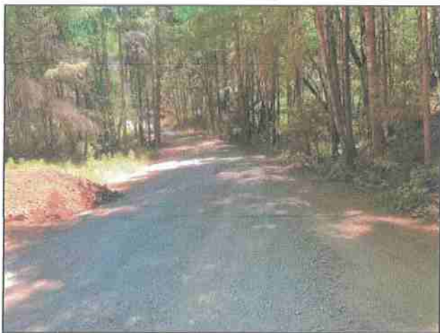
Photo #245 Thomas Rd @ Curve w/ Pullout Looking SE
