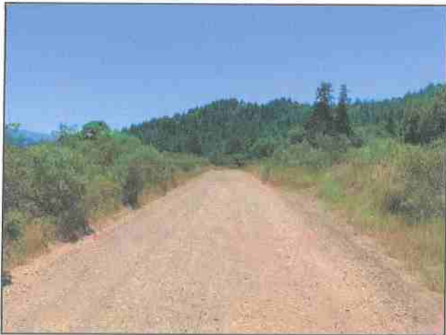
Photo #219 Thomas Rd Looking SE
