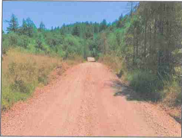
Photo #175 Thomas Rd Looking SE
