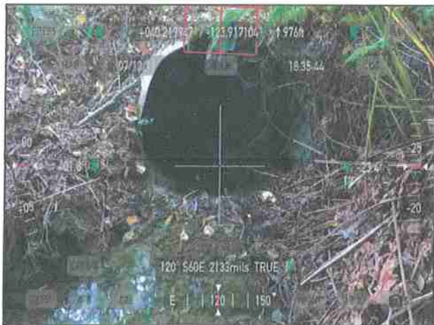
Photo #105 Private Access Rd APN 221-071-020 Looking @ 30" Culvert Outlet
