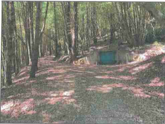
Photo #117 Private Access Rd APN 221-071-020 @ Curve w/ Pullout Looking SW Towards Storage
