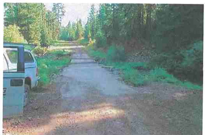
Figure 7. Concreted low-water crossing placed on bedrock outcrop in intermittent stream. Photo: Angela Wilson, Central Valley Regional Water Quality Control Board.
