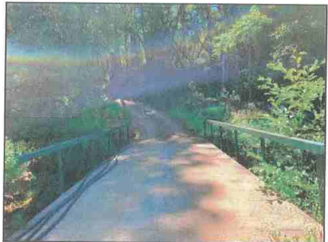
Photo #34 Private Access Rd APN 221-071-020 @ Bridge Looking SE
