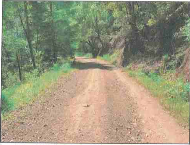
Photo #55 Private Access Rd APN 221-071-020 @ Pullout Looking SE @ Curve
