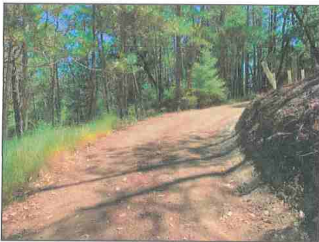
Photo #5 Private Access Rd APN 221-071-020 @ Curve w/ Pullout Looking SW
