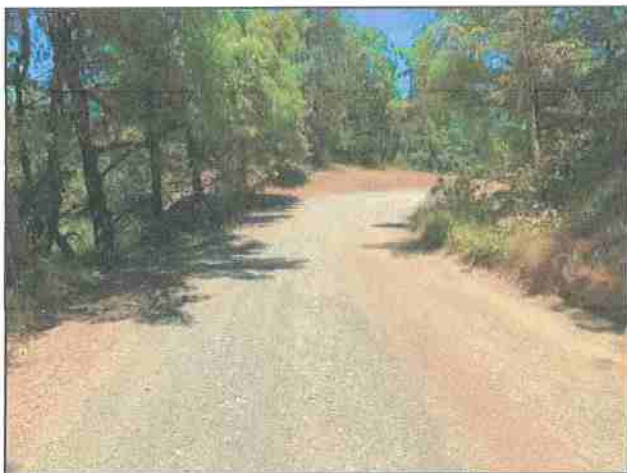
Photo #305 Thomas Rd @ Curve w/ Pullout Looking NE
