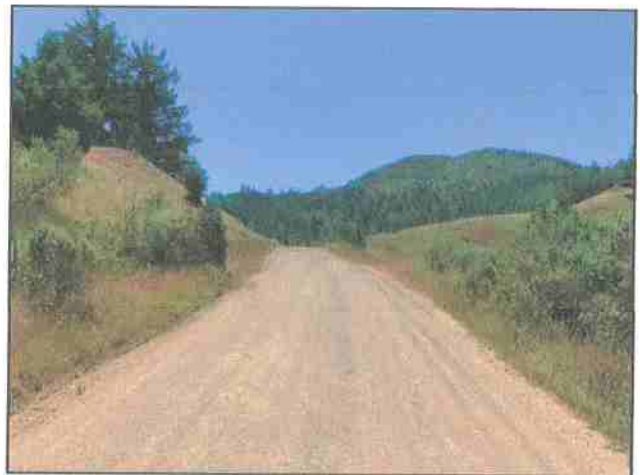
Photo #204 Thomas Rd Looking SW
