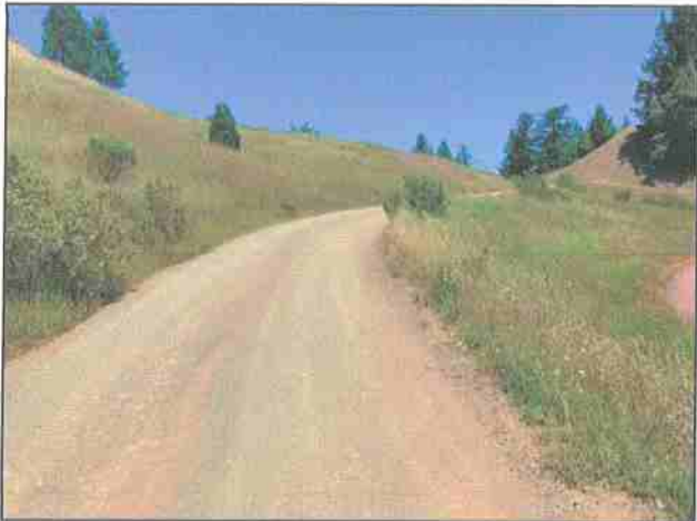
Photo #213 Thomas Rd @ Curve w/ Pullout Looking NE
