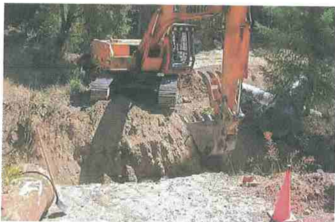
Figure 32. Excavator removing a crossing, including culvert and fill. Photo: Jared Gerstein.
