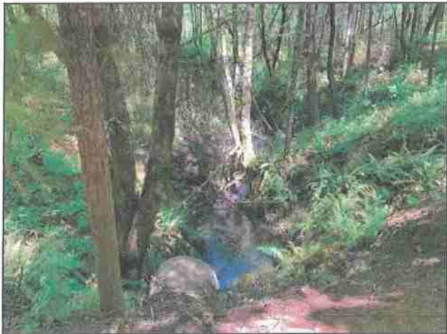
Photo #249 Thomas Rd Looking @ Culvert Outlet
