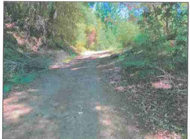
Photo #106 Private Access Rd APN 221-071-020 @ Curve w/ Pullout Looking NE
