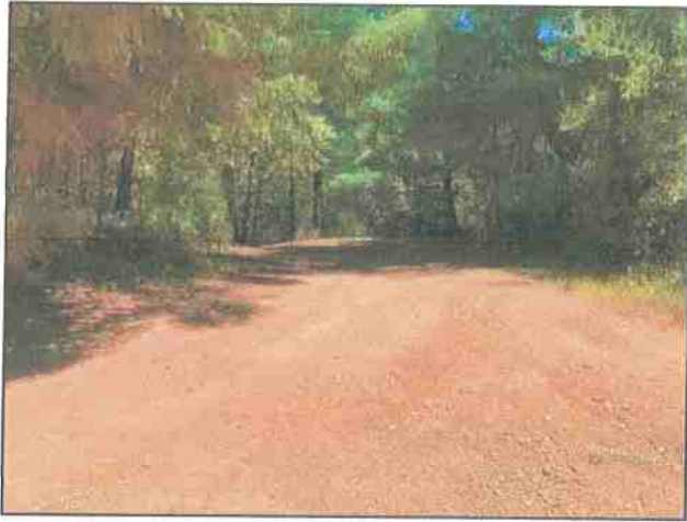
Photo #235 Thomas Rd @ Curve w/ Pullout Looking SE
