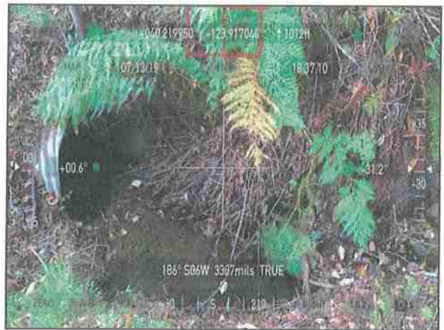
Photo #104 Private Access Rd APN 221-071-020 Looking @ 30" Culvert Inlet
