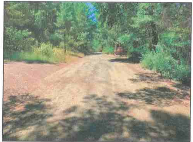
Photo #314 Thomas Rd @ Pullout Looking NW @ Curve & Private Driveway
