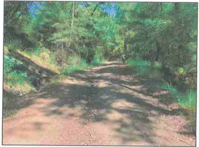
Photo #56 Private Access Rd APN 221-071-020 Pullout Looking NW @ Drainmage Issue
