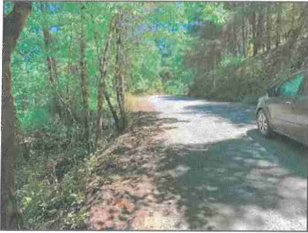
Photo #313 Thomas Rd @ Pullout Looking SE @ Curve
