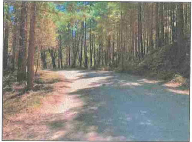
Photo #230 Thomas Rd @ Curve w/ Pullout Looking SE
