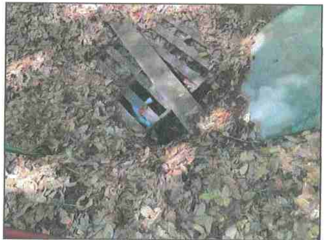
Photo #114 Private Access Rd APN 221-071-020 Looking @ Irrigation Piping Outside of Shoulder
