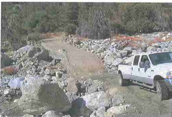
Figure 6. Low-water crossing on a perennial stream, San Bernardino County. Photo: Richard Harris.
