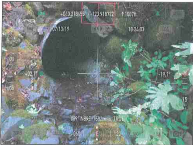
Photo #75 Private Access Rd APN 221-071-020 Looking @ 30" Culvert Size Outlet
