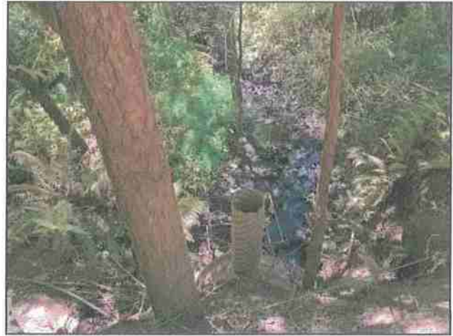
Photo #248 Thomas Rd Looking @ Culvert Inlet
