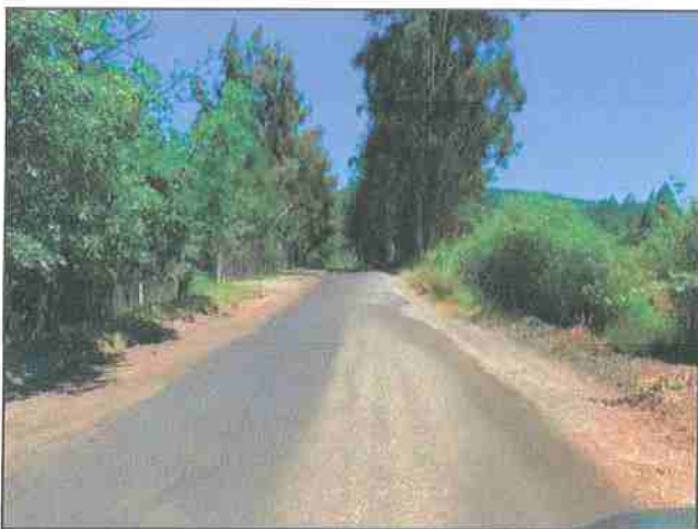
Photo #317 Thomas Rd @ End of County Maintained Road Looking SE
