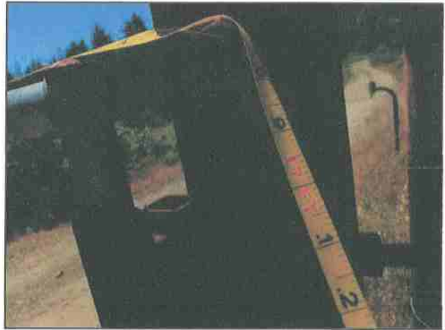
Photo #152 Salmon Creek Rd Gate Width 17'0"
