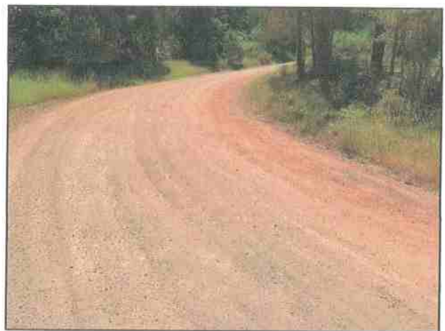
Photo #186 Thomas Rd @ Curve w/ Pullout Looking SE
