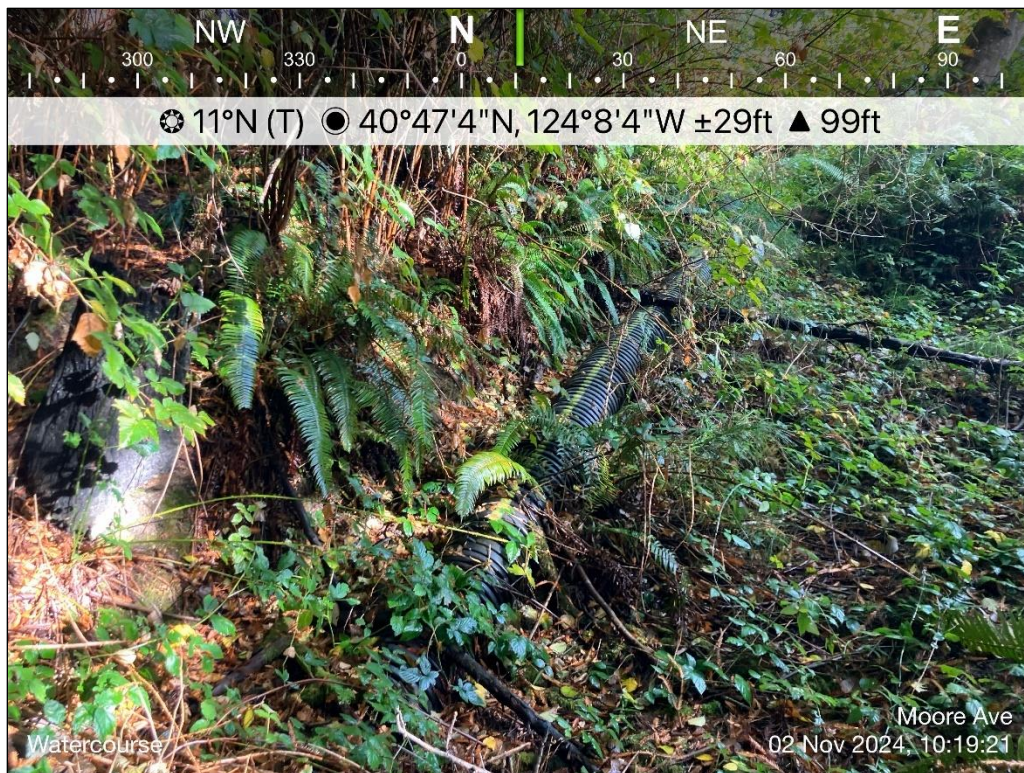
Photo 1. A culverted section of the intermittent Class II watercourse.
