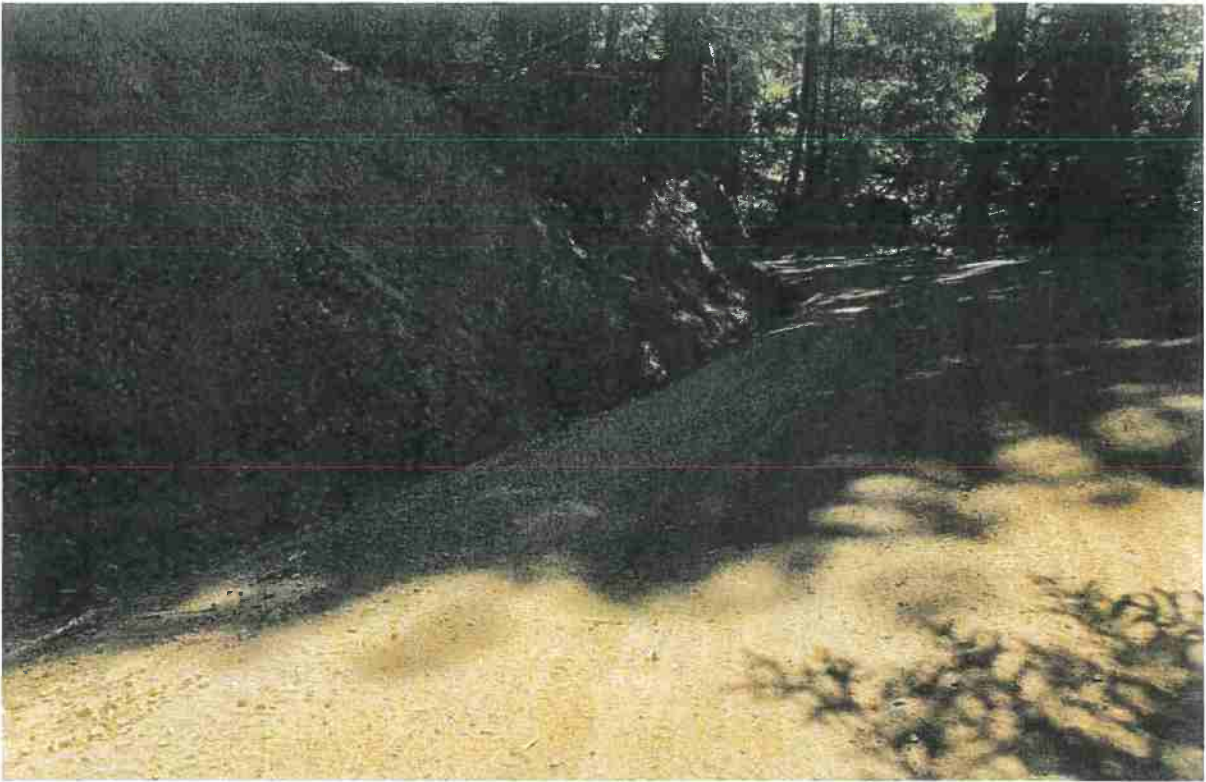
Photo looking up grade at the inside ditch that starts at Site 14 and extends down to Site 13.
