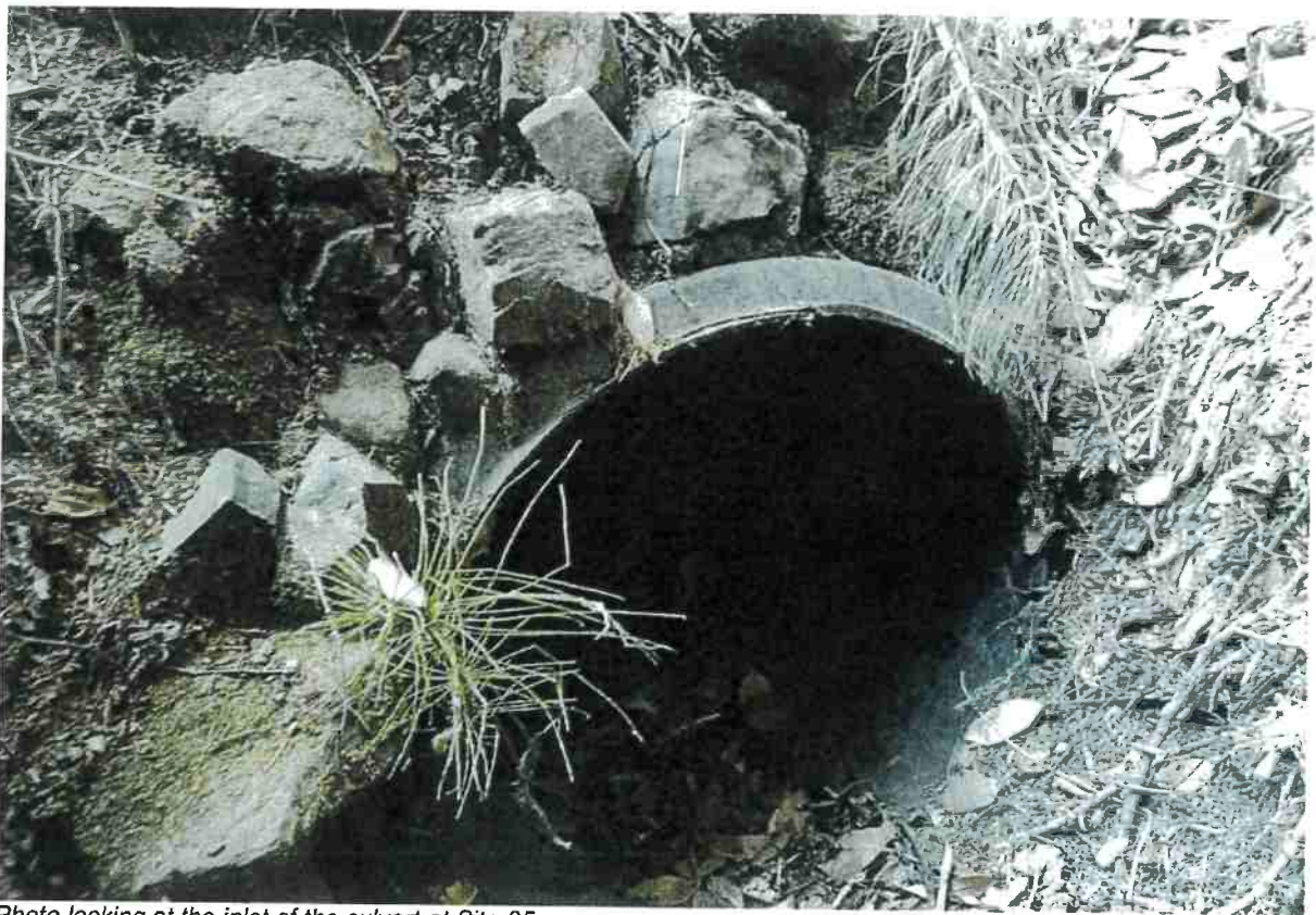
Photo looking at the inlet of the culvert at Site 05.
