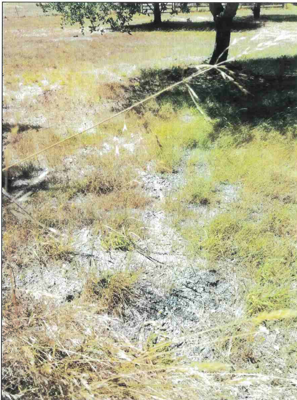
RP-4: Mobilized and deposited road material illustrating larger angular rock is need for road surfacing.
