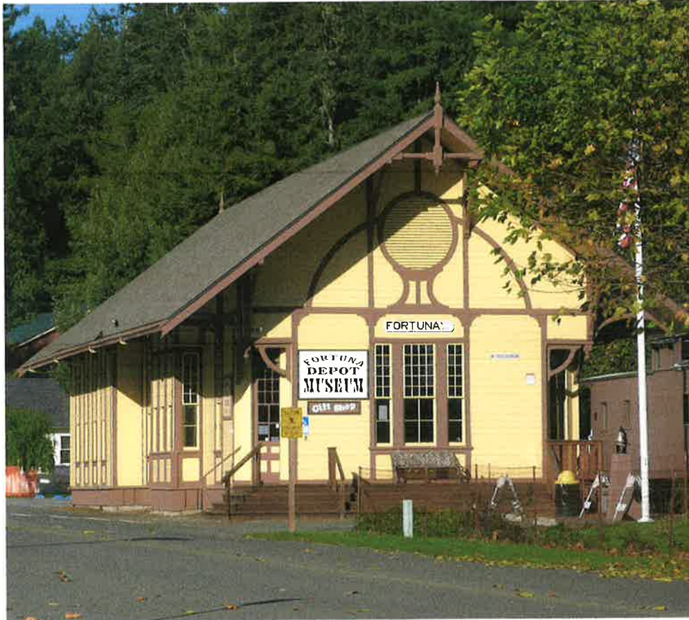
Fig 12. NWP (and predecessor) depot building 1893-1965, now Fortuna Depot Museum, after move to Rohner Park. A bell visible adjacent to the flag pole commemorates the loss of the engineer, fireman and brakeman who died at Scotia Bluff while working for the railroad 17 January 1953.
