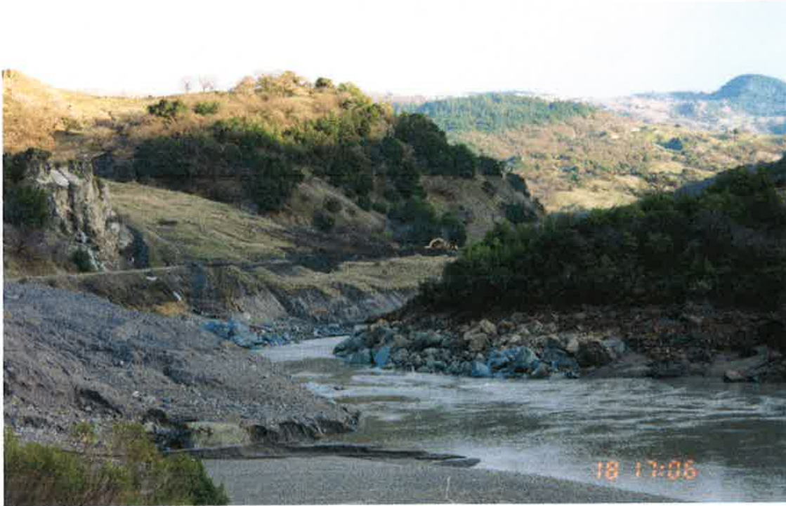
Fig. 9. MP 201 mud glacier c. late 1990's; J. Buck collection, photo attributed to Dan Hauser; note excavator recontouring grade for NCRA. (Slide is 900 feet wide, est. 2.75 miles long, 1600 feet over top of rail, 18 million cubic yards of material 31 )
