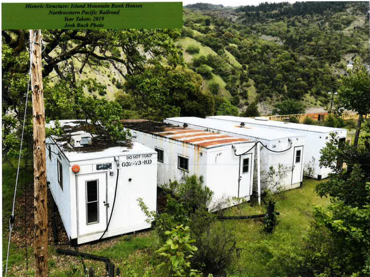
14 Island Mountain Metal Structures
