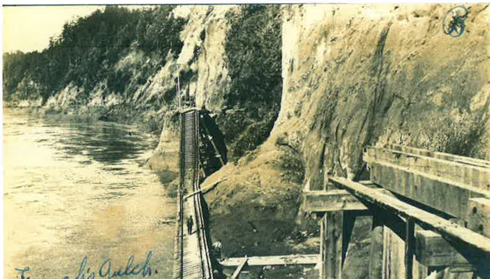
Fig 11. French's Gulch portion of Scotia Bluffs, postcard photo showing slide circa 1890-1906 knocking out TPLC trestle and roadbed, photographer unknown, from J. Buck collection. (Same route used by NWP.)
