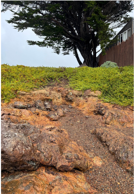
Exhibit 5a. Photo taken September 2025 showing erosion occurring below property at 495 Sea Ct.
