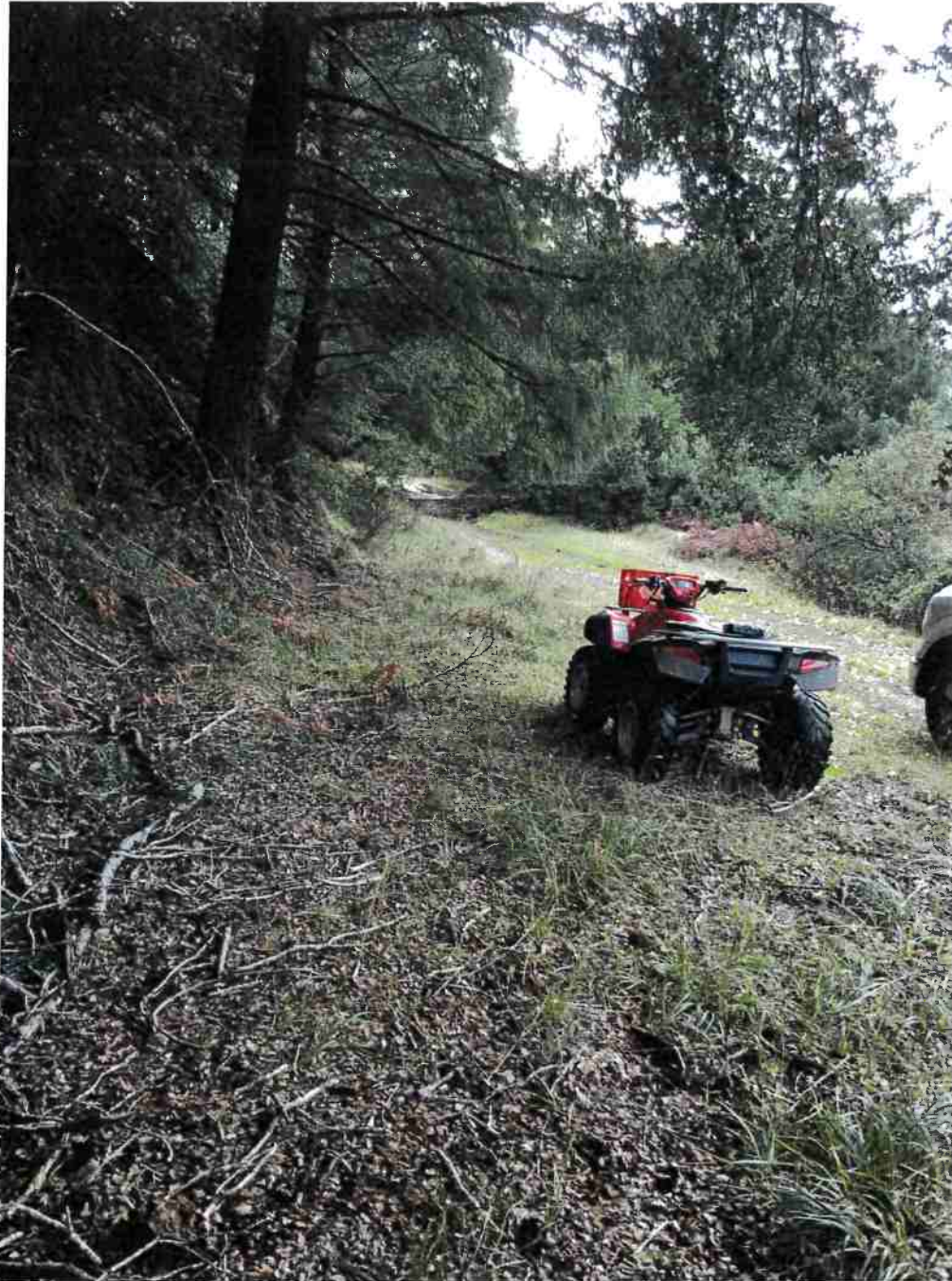
Picture 14: Map Point #3. Picture taken from outlet of Crossing #2 looking southerly to the inlet of Crossing #4. The rock-lined ditch shall be constructed east (photo left) of the access road shown above. Photo date 12-2-2016.
