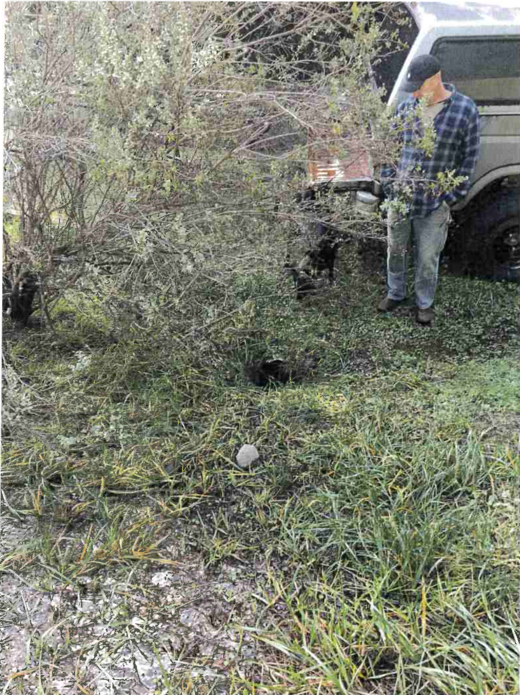
Picture 21: Inlet of Crossing #7. Photo date 8-31-2016.
