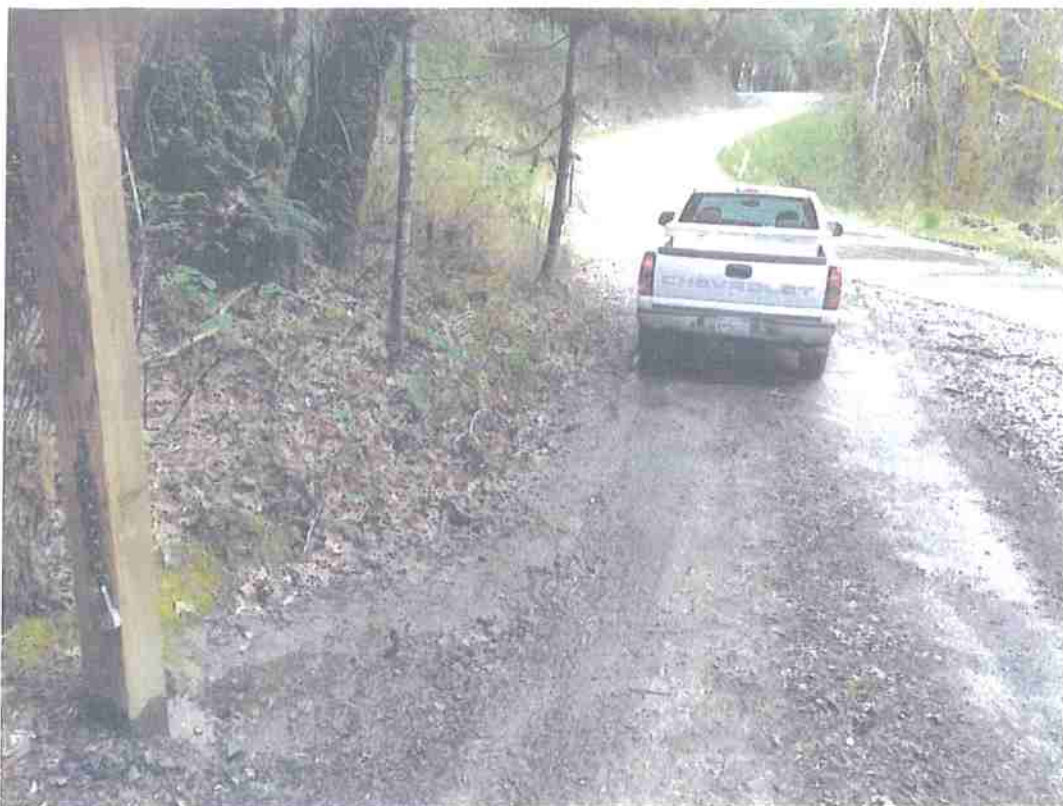
Photo 8. Seep at entrance gate. Construct rolling dip or French drain to diver surface flow to road-right.
