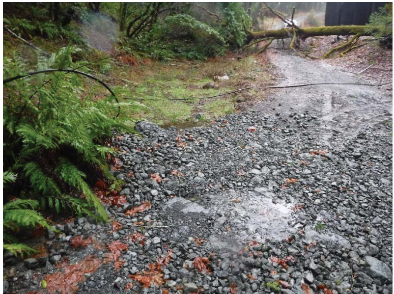
Figure 1: Before (4/25/18) and after (1/18/19) photos of the crossing at MP-1. An armored rock ford has been installed across the road temporarily to allow vehicle and equipment access to the site. Photos taken looking upstream (west).
