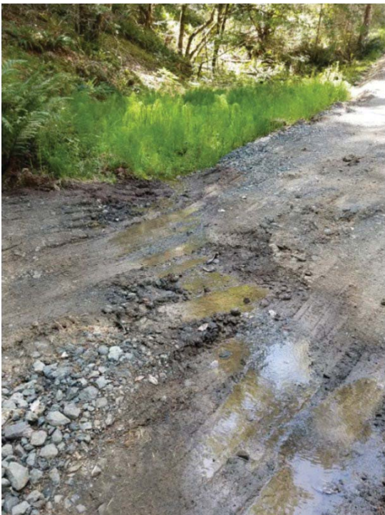
Figure 1: Before (4/25/18) and after (1/18/19) photos of the crossing at MP-1. An armored rock ford has been installed across the road temporarily to allow vehicle and equipment access to the site. Photos taken looking upstream (west).
