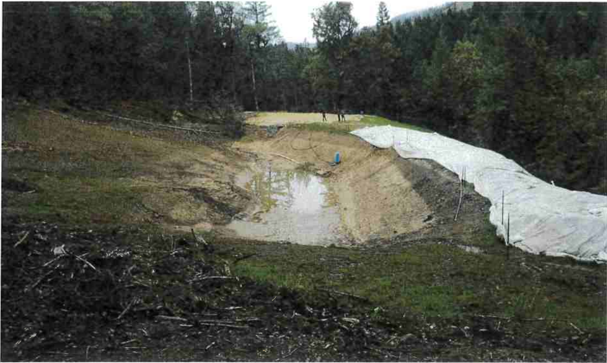
IMG 0826 1.3 acre illegal clearing with large pond in center
