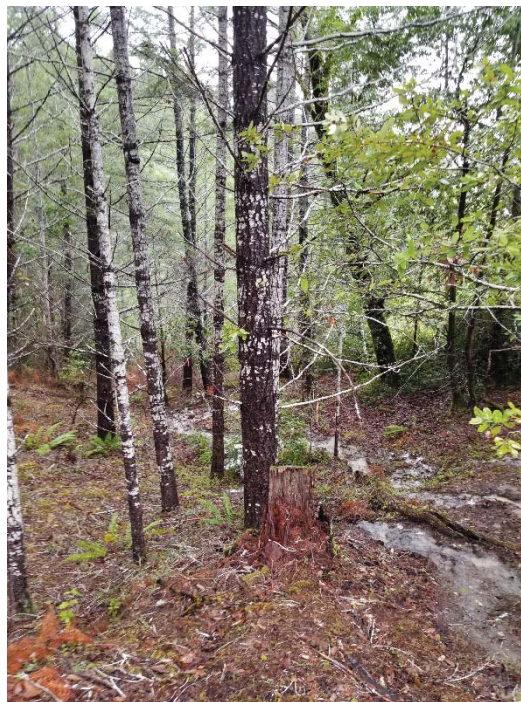
Figure 27: Path of flow from constructed drainage swale into forest just downstream of the armored interface shown in Figure 26. This flow joins an existing Class III watercourse approximately 200 linear feet from this point, which discharges ultimately into Salmon Creek. Photo taken looking northwest on 1/8/19.
