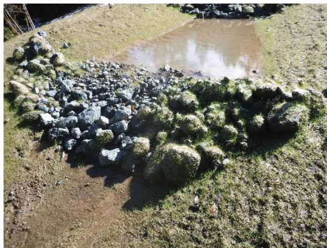
Figure 25: Typical checkdam installed in drainage swale. Photo taken looking upstream (east) on 2/5/19.
