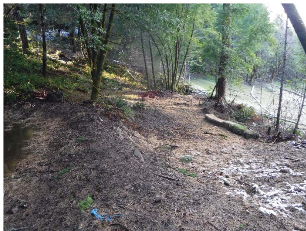
Figure 8: View of the rerouted reach of MP-5 looking upstream. This is approximately where the decommissioned road intercepted the watercourse. The reconstructed slope can be seen in the background. Photos taken looking west on 2/5/19.
