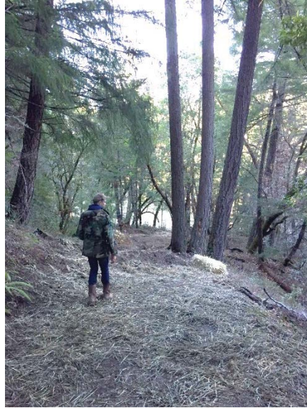
Figure 14: Water bar installed between MP-5 and MP-6. A straw bale was installed at the outlet of the bar and straw mulch placed for erosion control. Photo taken looking northwest on 12/6/18.
