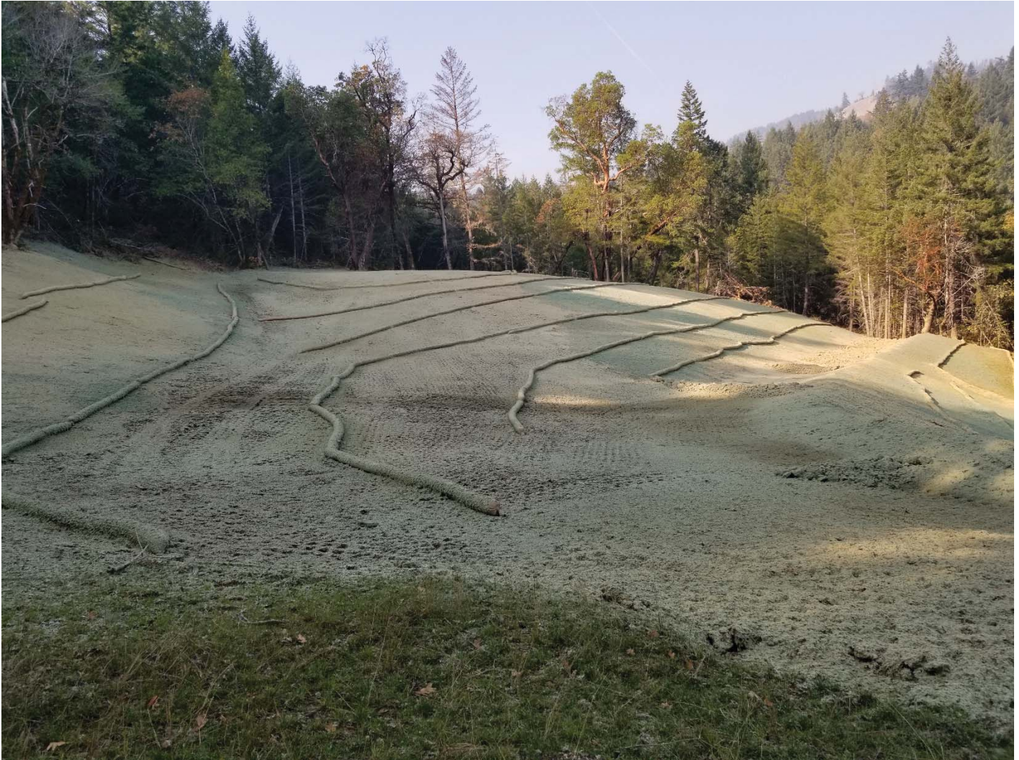
Figure 20: Reconstructed slopes showing hydroseed application and fiber rolls on contours. The former pond site is approximately in the center of this photo. All disturbed surfaces received surface treatment including hydroseed, straw mulch, and/or fiber rolls or jute netting to prevent erosion. Photo taken looking northwest on 11/14/2018.
