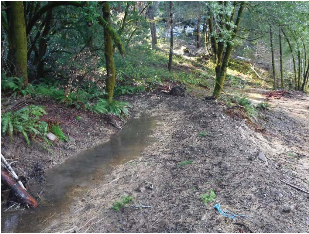
Figure 8: View of the rerouted reach of MP-5 looking upstream. This is approximately where the decommissioned road intercepted the watercourse. The reconstructed slope can be seen in the background. Photos taken looking west on 2/5/19.
