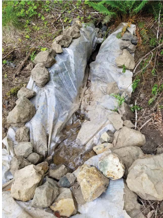
Figure 5: Before (4/25/18) and after (5/9/18) installation of the cofferdam diversion on MP-5. This temporary measure will be removed before October 2019. Photo taken looking southeast.
