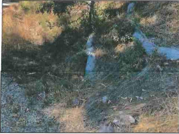
Photo #169 River Rd Looking @ Partially Clogged 24" Culvert Under Approach Running E to W
