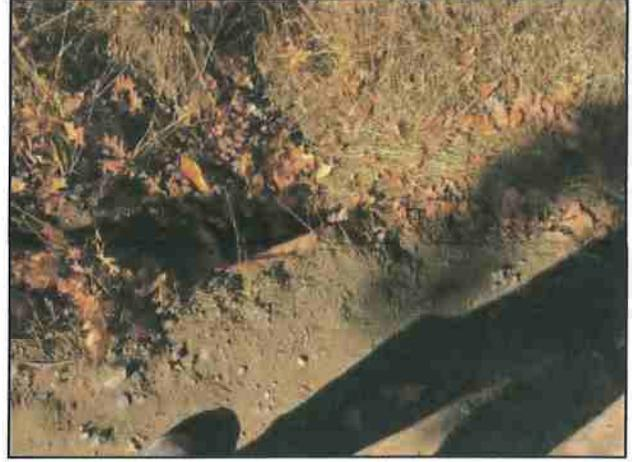
Photo #50 River Rd Partially Clogged 12" Culvert In
