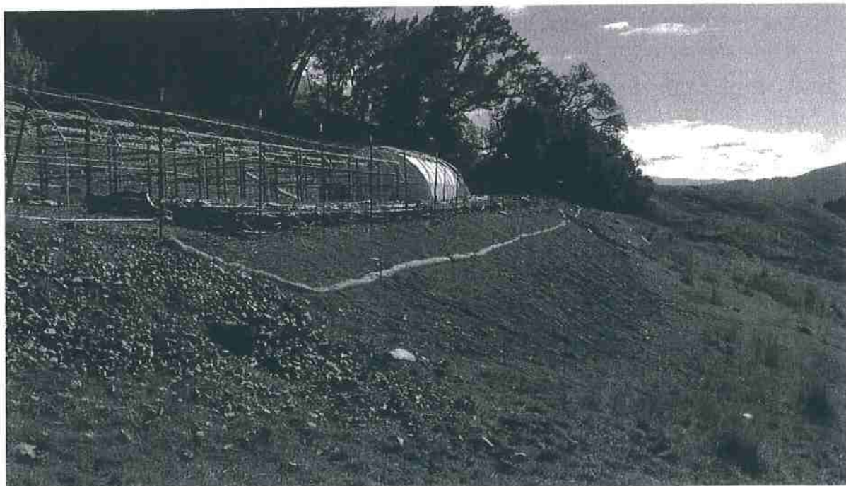
Cultivation Area A looking at the fillslope below the cultivation area. The outlet for the ditch relief culvert at Site 09 can be seen in the bottom left.
