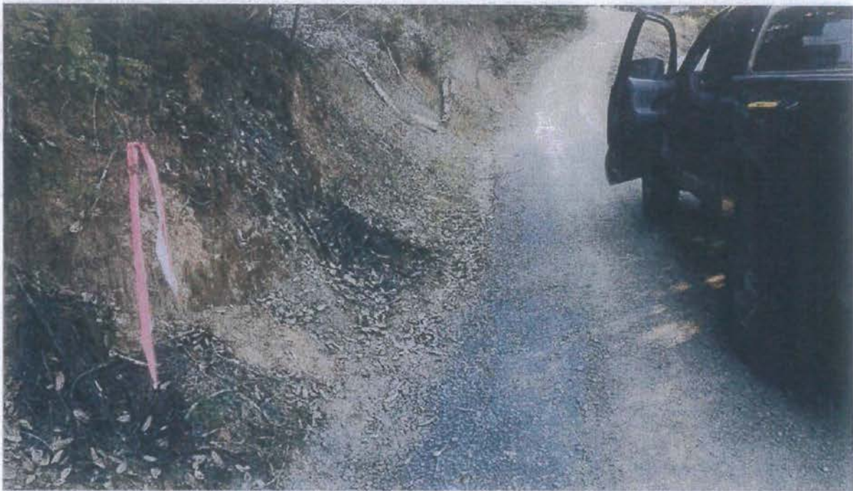
Photo looking up grade at Site 06. Staked straw wattles will be installed across the inside ditch to capture sediment eroding away from a cutbank slump.
