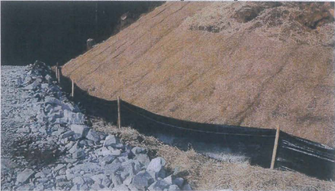
Erosion Control Matting & Silt Fencing
