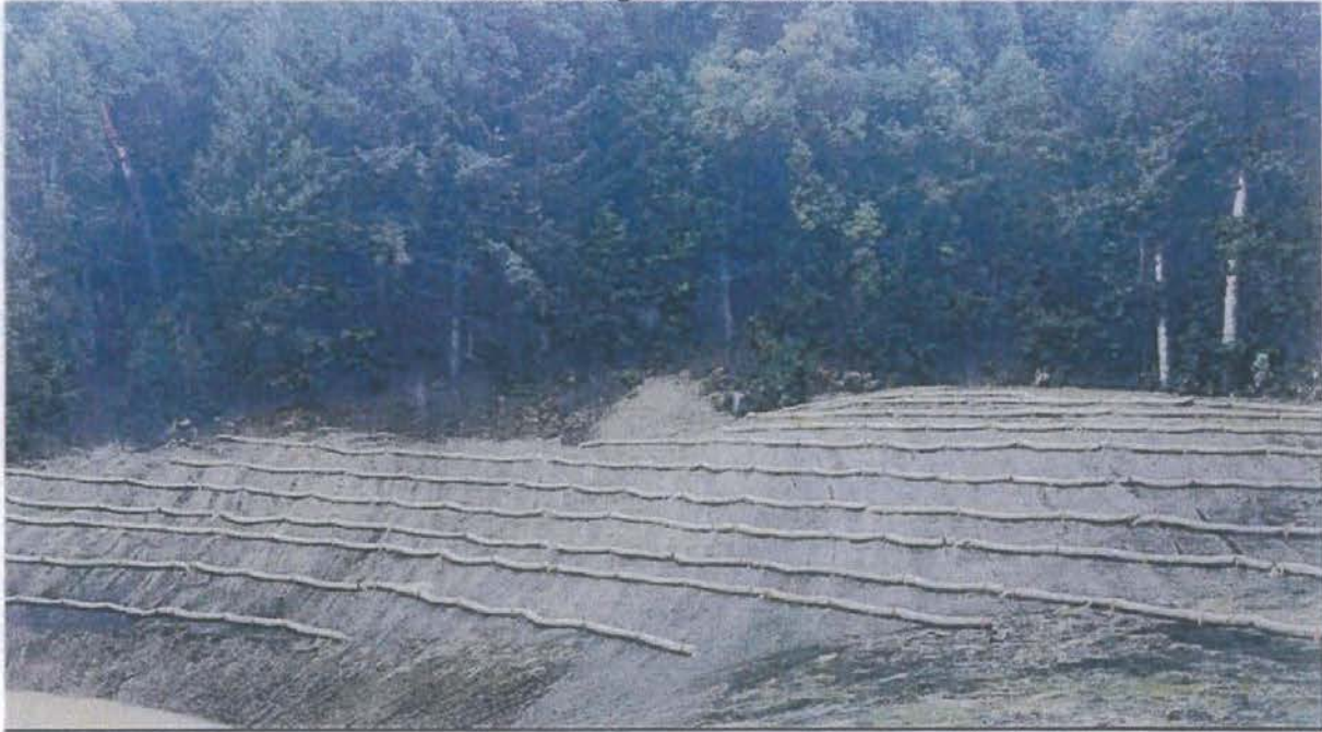
Jute netting & Straw-wattles
