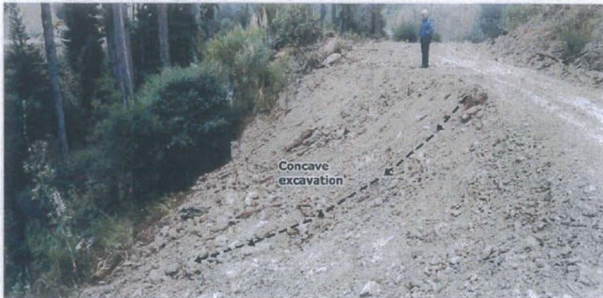
FIGURE 230. The most cost-effective treatment for unstable fills along the outside of a forest, ranch or rural road is simply the direct excavation of the unstable material. If road width is too narrow, additional width can often be derived from cutting into the bank. The excavation should encompass the unstable fill materials, beginning at the inside crack or scarp, and extending out and down the fill slope as far as possible. For proper surface drainage, and to retrieve most of the unstable fill, the excavation should have a concave profile when completed. Typically, the bulk of the fill is within 20 to 25 feet of the outside edge of the road and is easily reached by a mid-sized excavator. Any remaining fill is likely to be small enough that it will not fail or travel far enough to reach the stream.
