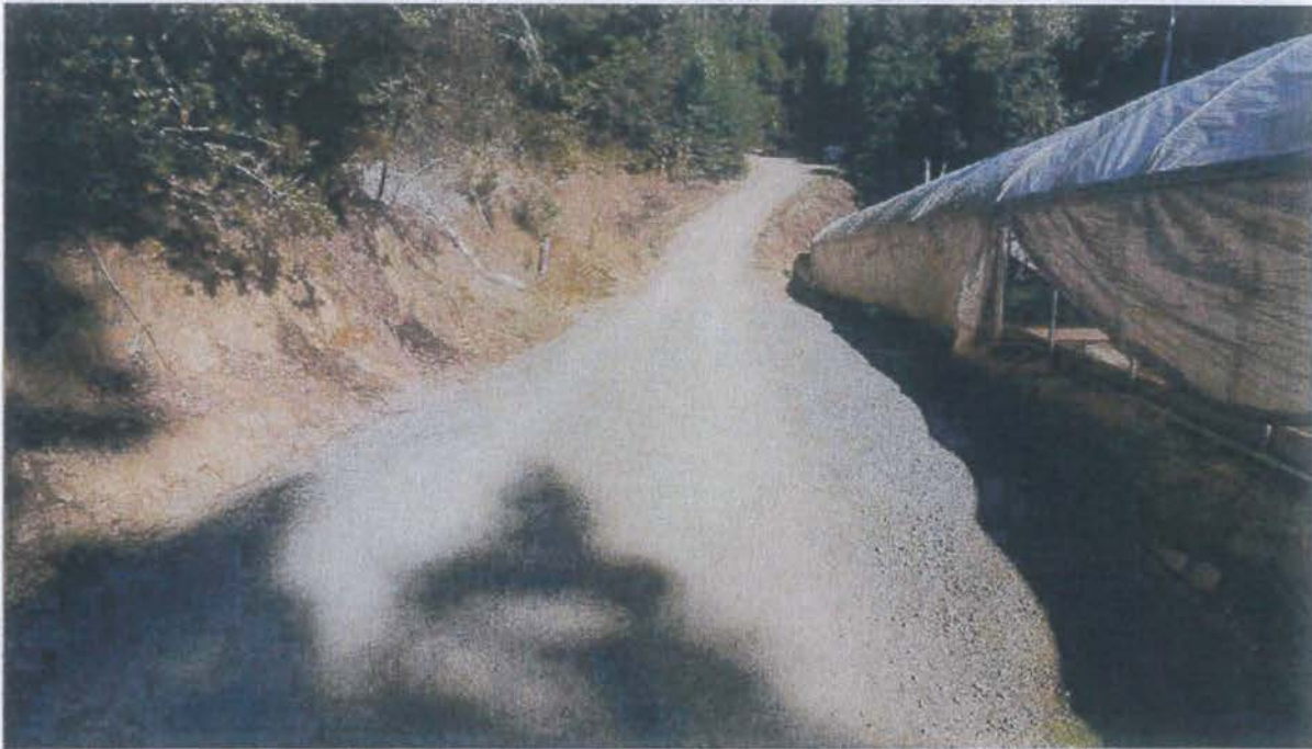
Photo looking up grade at Site 06.
