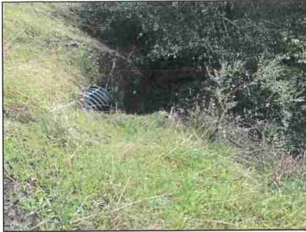
Photo #13 Private Access Rd Looking @ 18" Culvert Out
