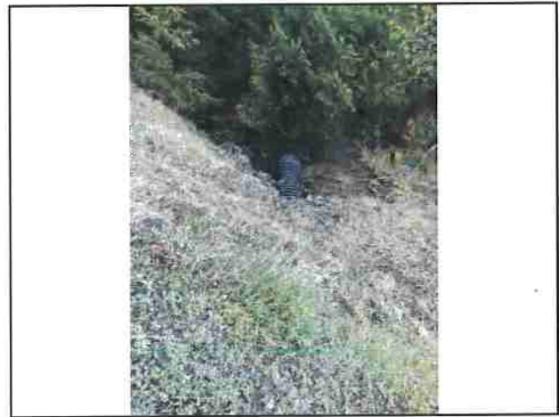
Photo #64 Private Access Rd Looking @ 18" Culvert Out
