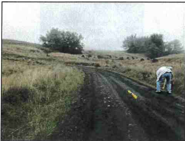
Photo #71 Private Access Rd @ Pullout Looking SW @ Curve
