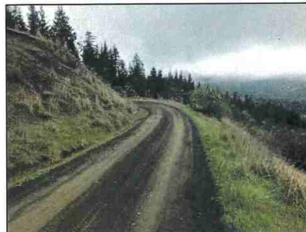
Photo #17 Private Access Rd @ Curve w/ Pullout Looking NW
