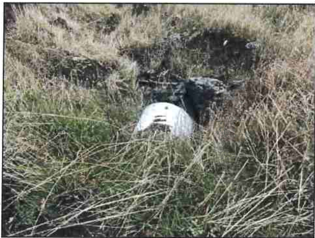
Photo #21 Private Access Rd Looking @ 18" Culvert Out
