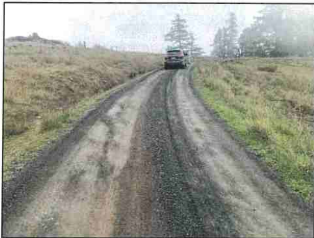
Photo #93 Private Access Rd @ Pullout Looking NE @ Curve
