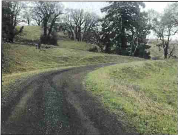
Photo #57 Private Access Rd Looking @ Curve w/ Pullout Looking SW
