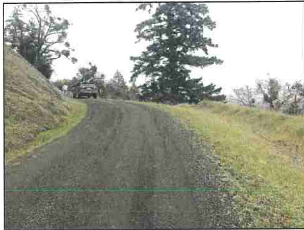
Photo #51 Private Access Rd Looking @ Curve w/ Pullout Looking NE
