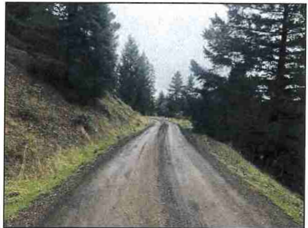
Photo #10 Private Access Rd @ Pullout Looking SW @ Curve
