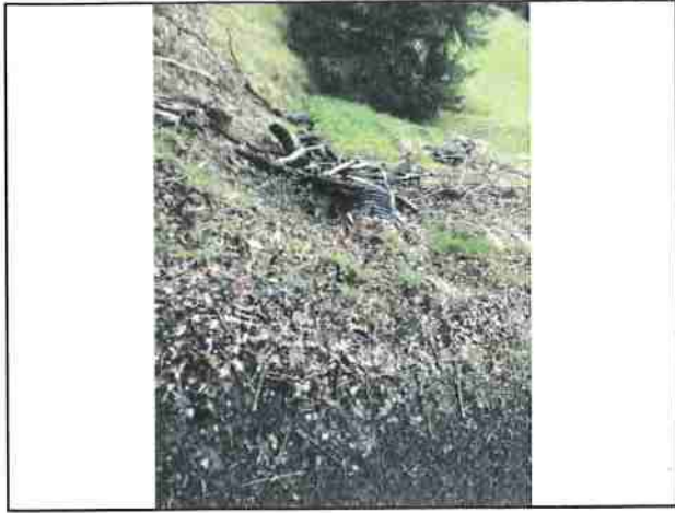
Photo #49 Private Access Rd Looking @ 12" Culvert Out
