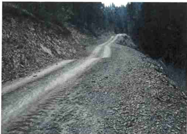
Figure 8. Rolling dips installed to drain an out-sloped road. Source: Bill Weaver, Pacific Watershed Associates.
