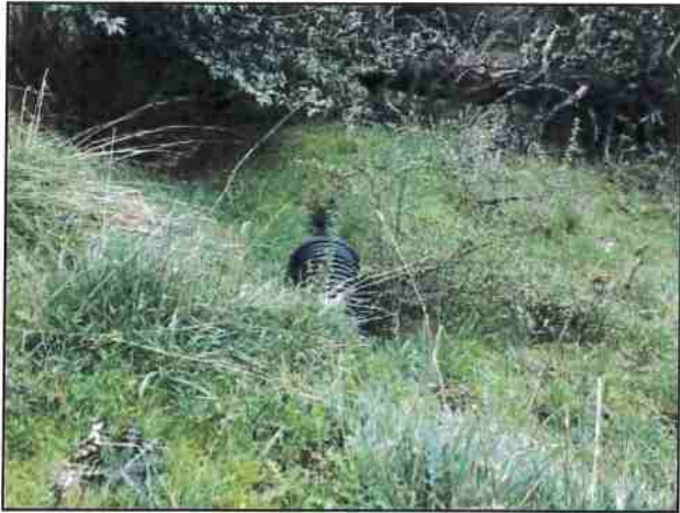
Photo #9 Private Access Rd Looking @ 18" Culvert Out
