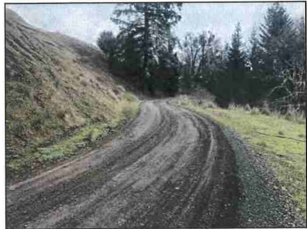
Photo #4 Private Access Rd @ Curve w/ Pullout Looking SW
