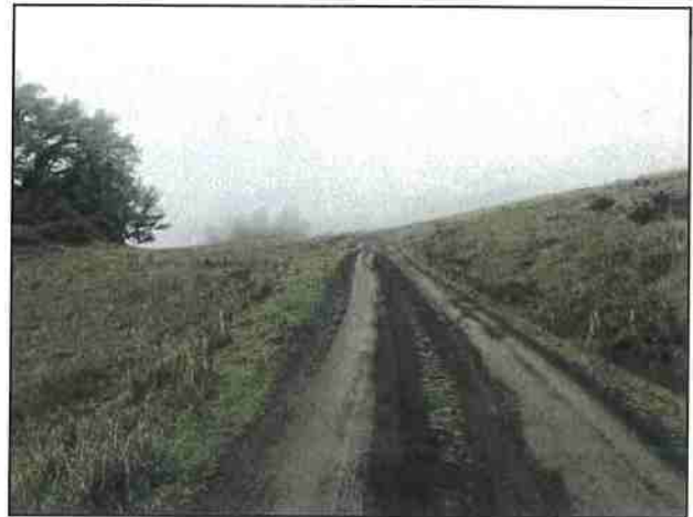
Photo #92 Private Access Rd @ Pullout Looking NE @ Curve
