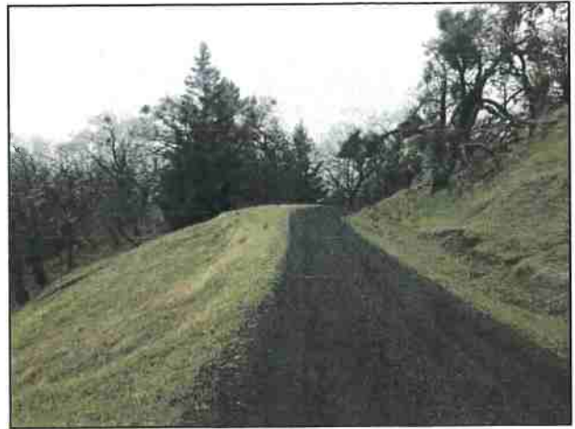
Photo #50 Private Access Rd Looking @ Curve w/ Pullout Looking SW
