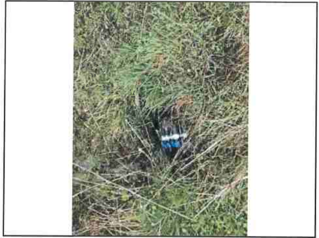
Photo #32 Private Access Rd Looking @ 18" Culvert In
