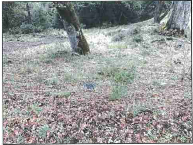
Photo #38 Private Access Rd Looking @ 12" Culvert Out
