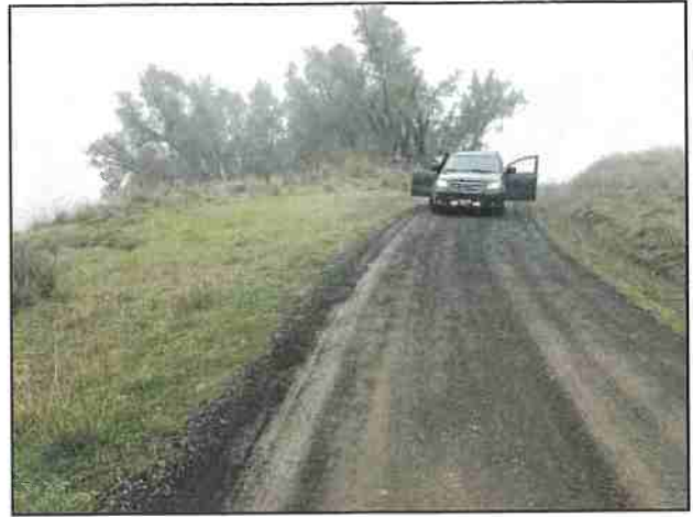
Photo #86 Private Access Rd @ Pullout Looking SW @ Curve
