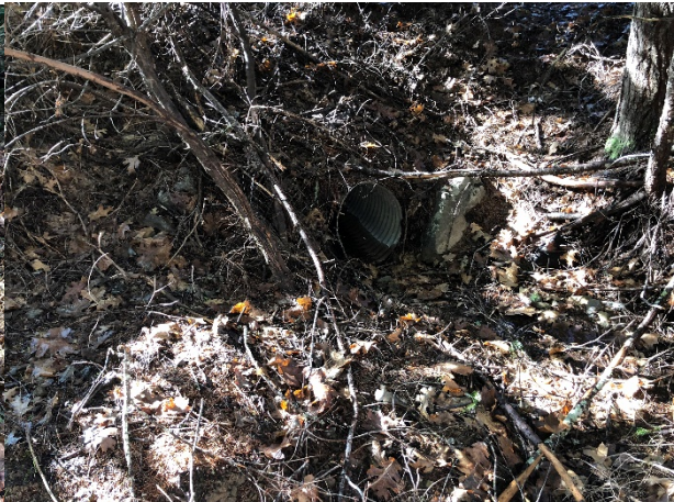
Picture #42 Cobb Rd looking @ inlet of 12" culvert
