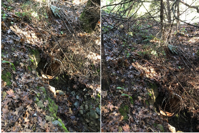
Picture #43 Cobb Rd inlet of 12" culvert Picture #44 Cobb Rd outlet from culverts in Pictures 42 & 43.
