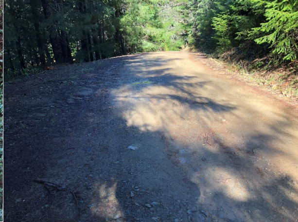
Picture #50 Cobb Rd looking SW towards curve.
