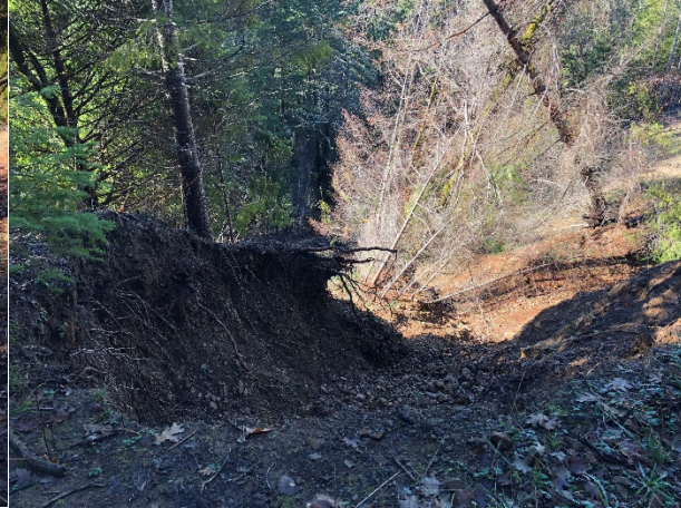
Picture #20 On PG&E esmt looking SW @ erosion.
