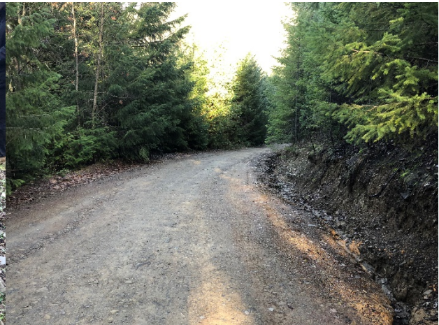
Picture #4 Cobb Rd @ curve looking NW
