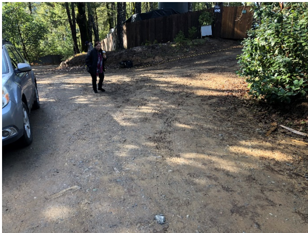
Picture #35 Cobb Rd looking SW towards curve
