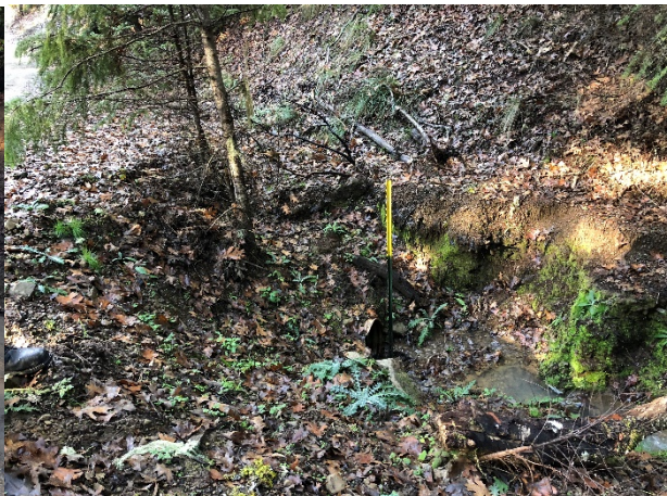
Picture #30 Cobb Rd 12" culvert inlet
