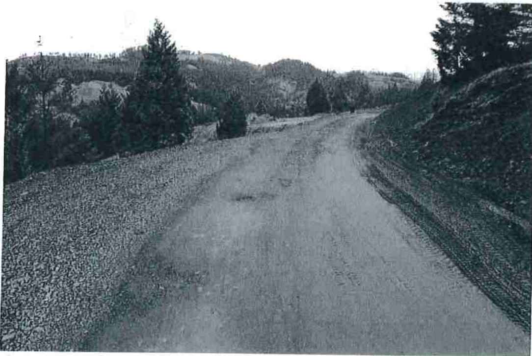
Photo 32 - Mile 2.8: 18' width 2' shoulders, dangerous corner, perhaps add some signage to slow down
