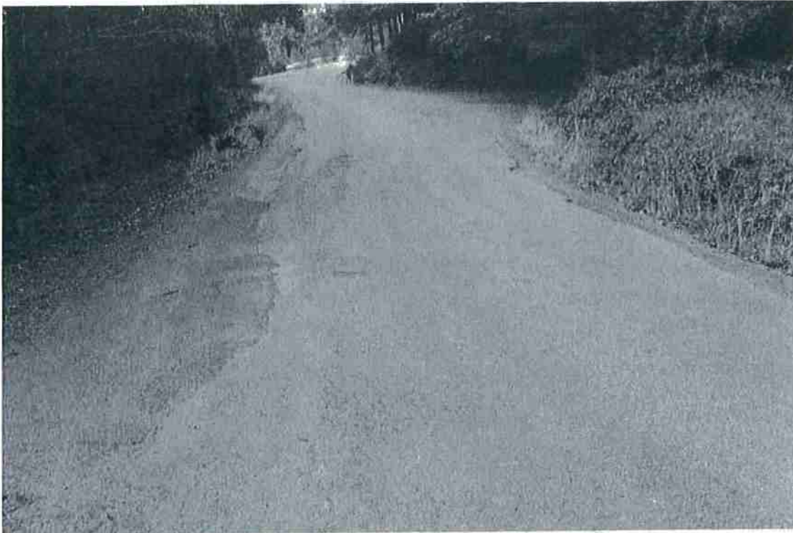
Photo 33. Mile 2.9: 18-ft road width with 1-ft shoulders.
