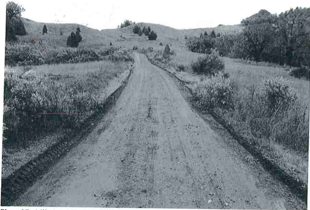
Photo 27 - Mile 2.4: 15' width 2' shoulders, great visibility, with turnouts
