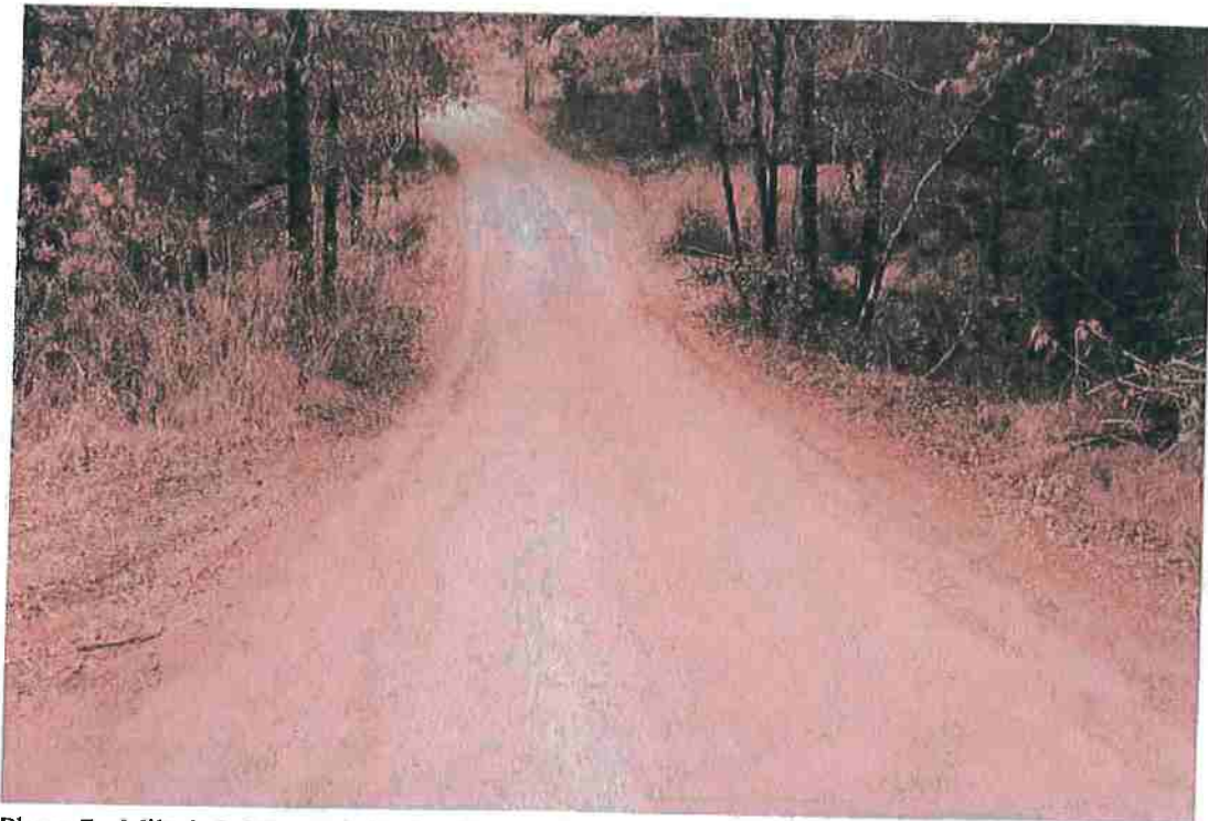
Photo 7 - Mile 0.6: 16' width 1' shoulders, culvert crossing, good visibility
