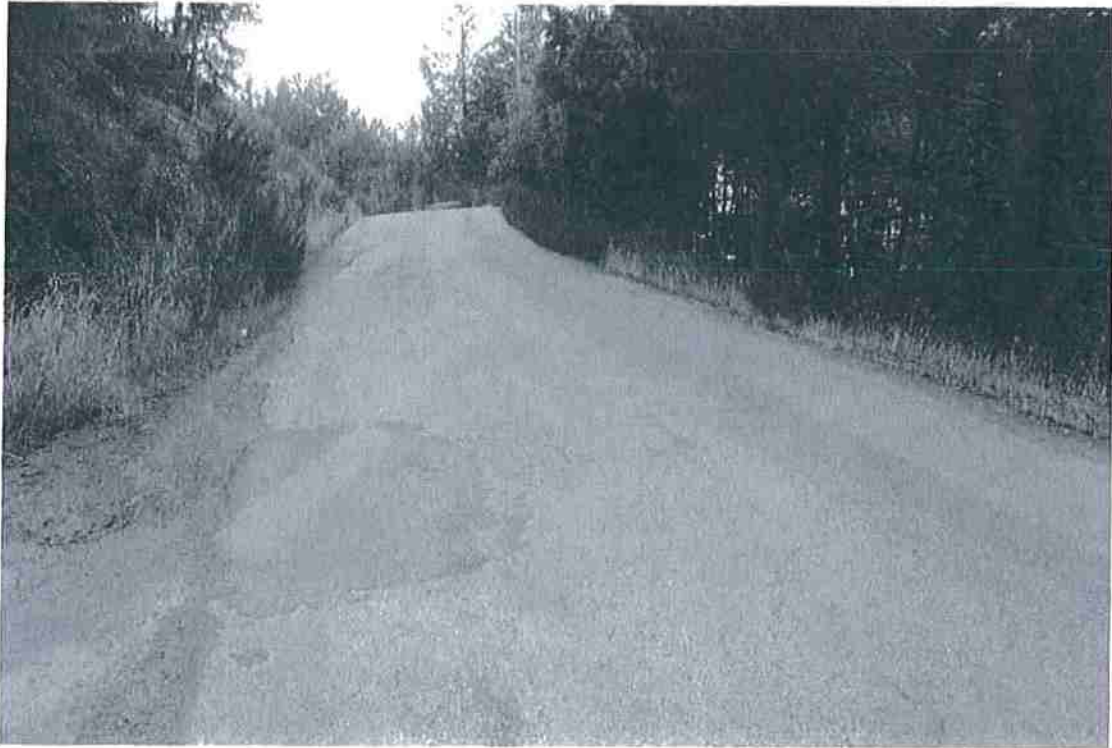
Photo 31. Mile 2.7: 20-ft road width with 2-ft shoulders.
