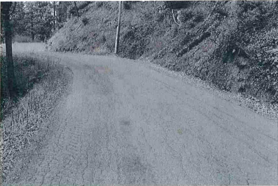
Photo 22. Mile 2.1: 18-ft road width with 1-ft shoulders.
