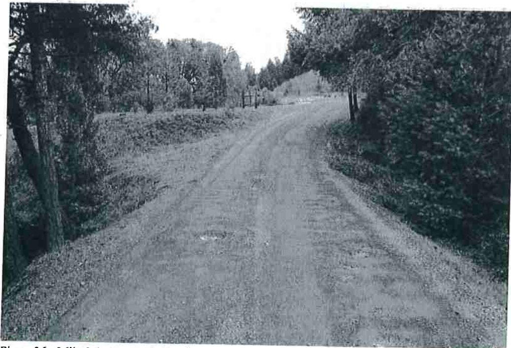
Photo 36 - Mile 3.1: 14' width @ culvert crossing, good visibility with turnouts on both sides
