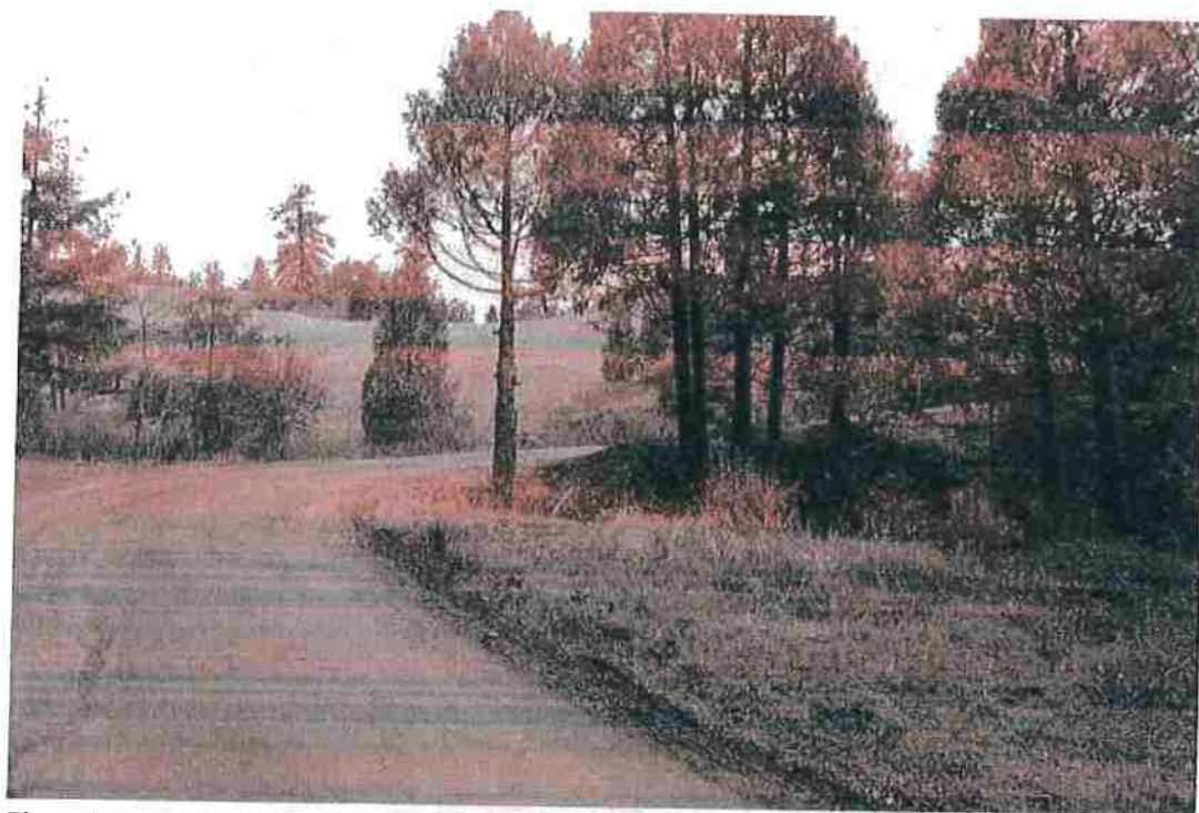
Photo 16 - Mile 1.35: Tight corner but has 18' width, 1' shoulders, remove more vegetation to improve visibility
