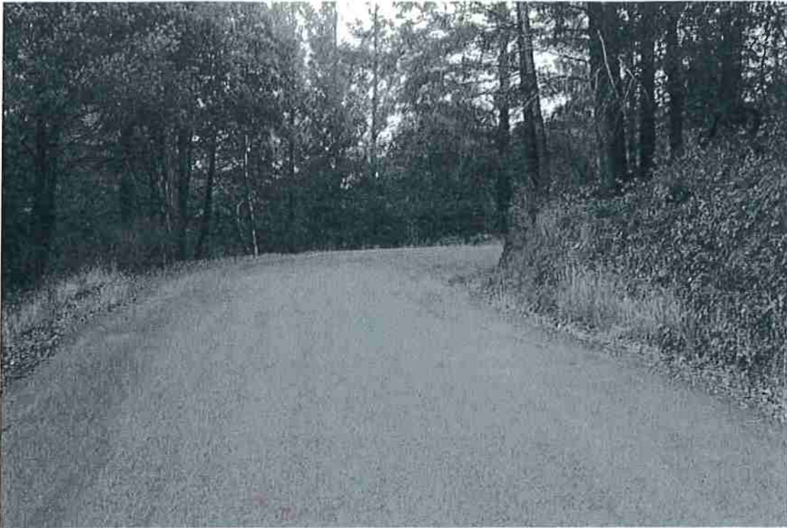
Photo 13. Mile 1.2: 20-ft road width with 1-ft shoulders.
