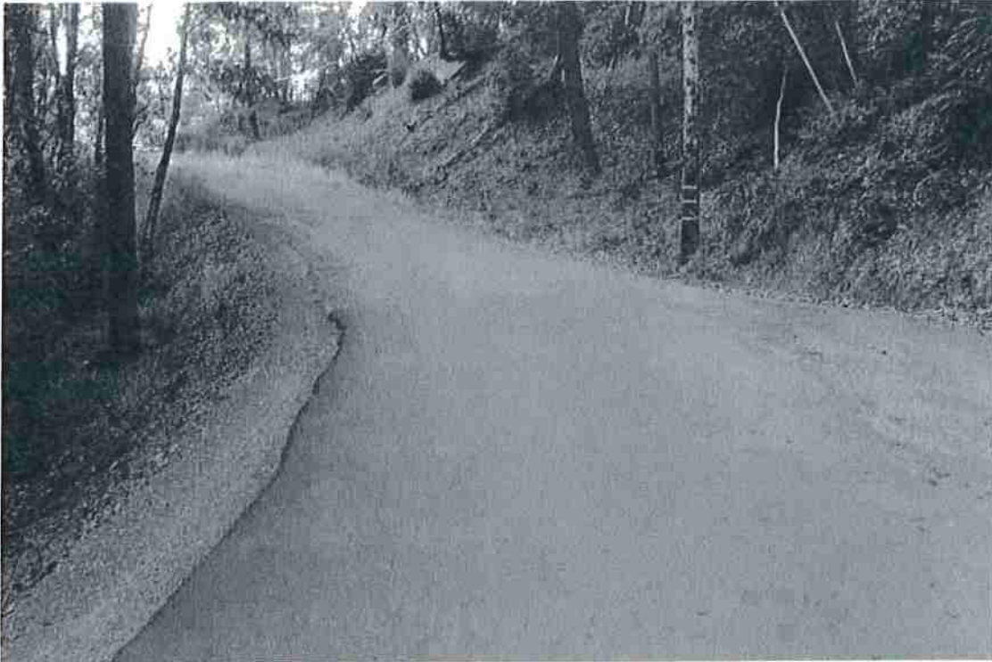
Photo 29. Mile 2.5: 18-ft road width with 2-ft shoulders.
