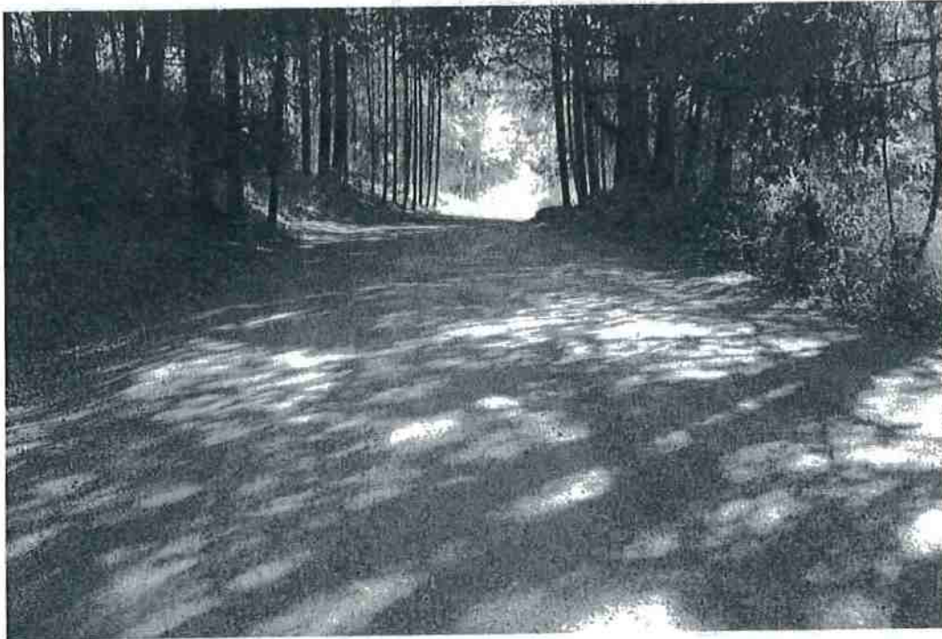
Photo 17. Mile 1.4: 20-ft road width with 2-ft shoulder.
