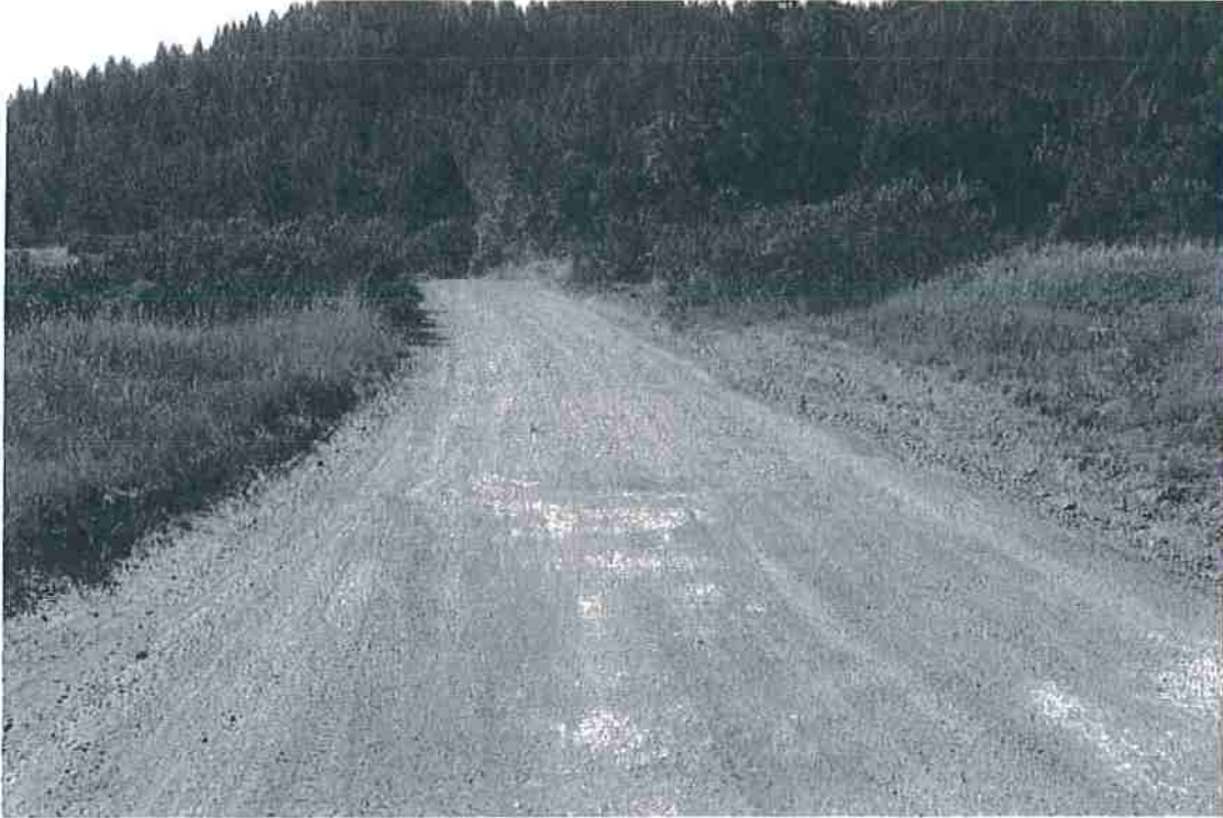
Photo 19. Mile 1.6: 18-ft road width with 1-ft shoulder. End of Segment 3 at Salmon Creek School.
