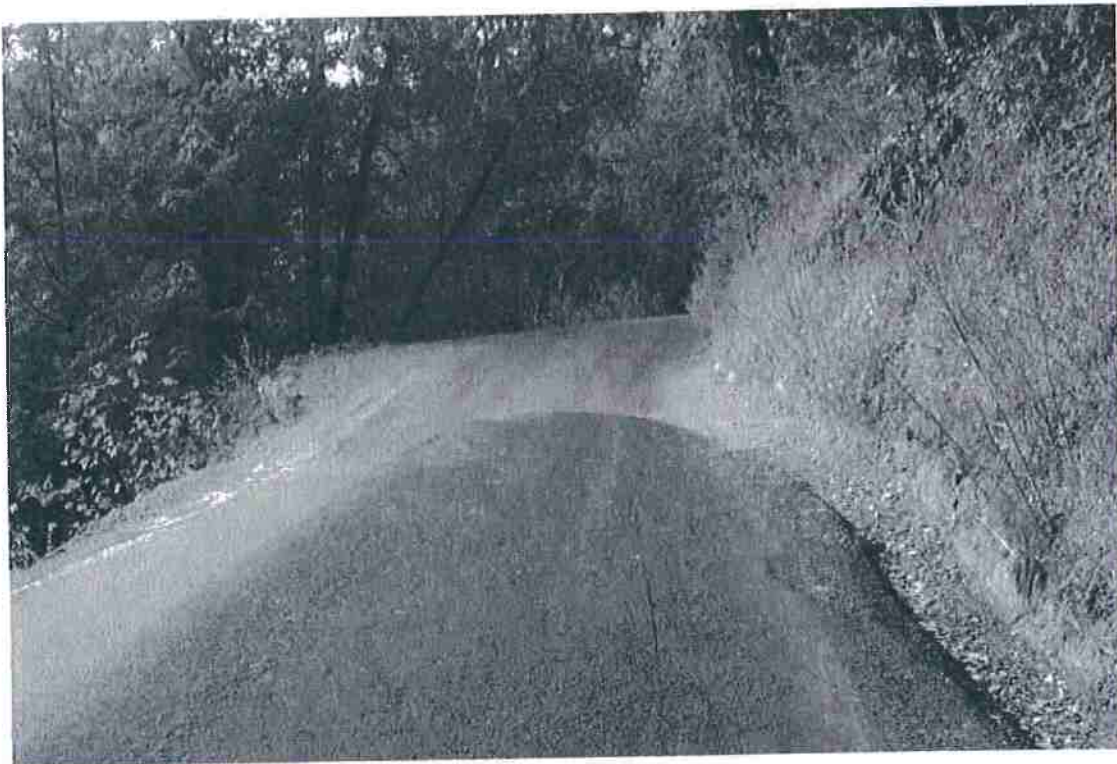
Photo 4. Mile 0.9: relatively narrow section, 15' width, 1' shoulders.
