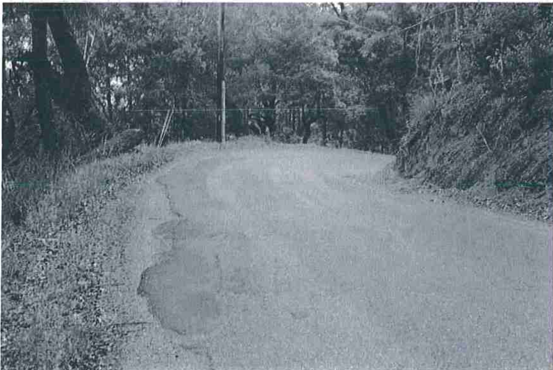
Photo 24. Mile 2.2: 20-ft road width with 1-ft shoulders.
