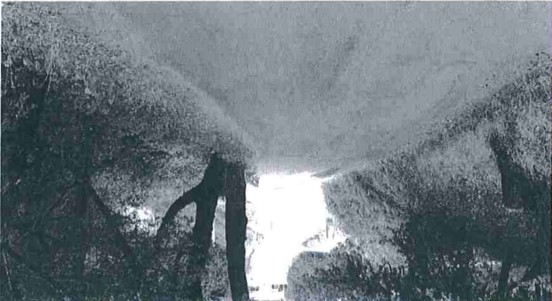
Photo 5. Mile 0.45: Pinch point at tree, 16-ft road width, decent visibility.
