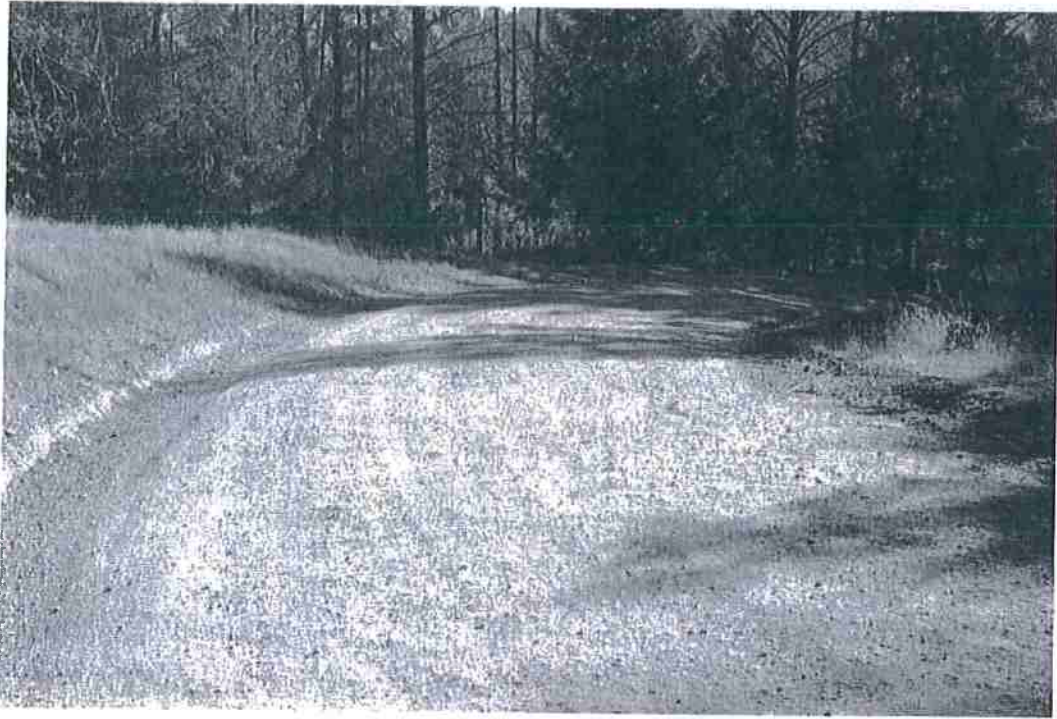
Photo 3. Mile 0.3: 20-ft road width with 2-ft shoulder.
