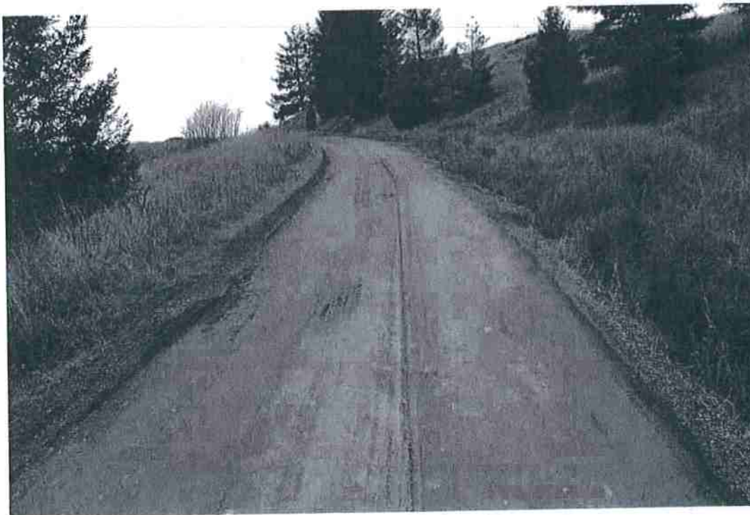
Photo 22 - Mile 1.9: 14' width 2' shoulders, great visibility, with turnouts
