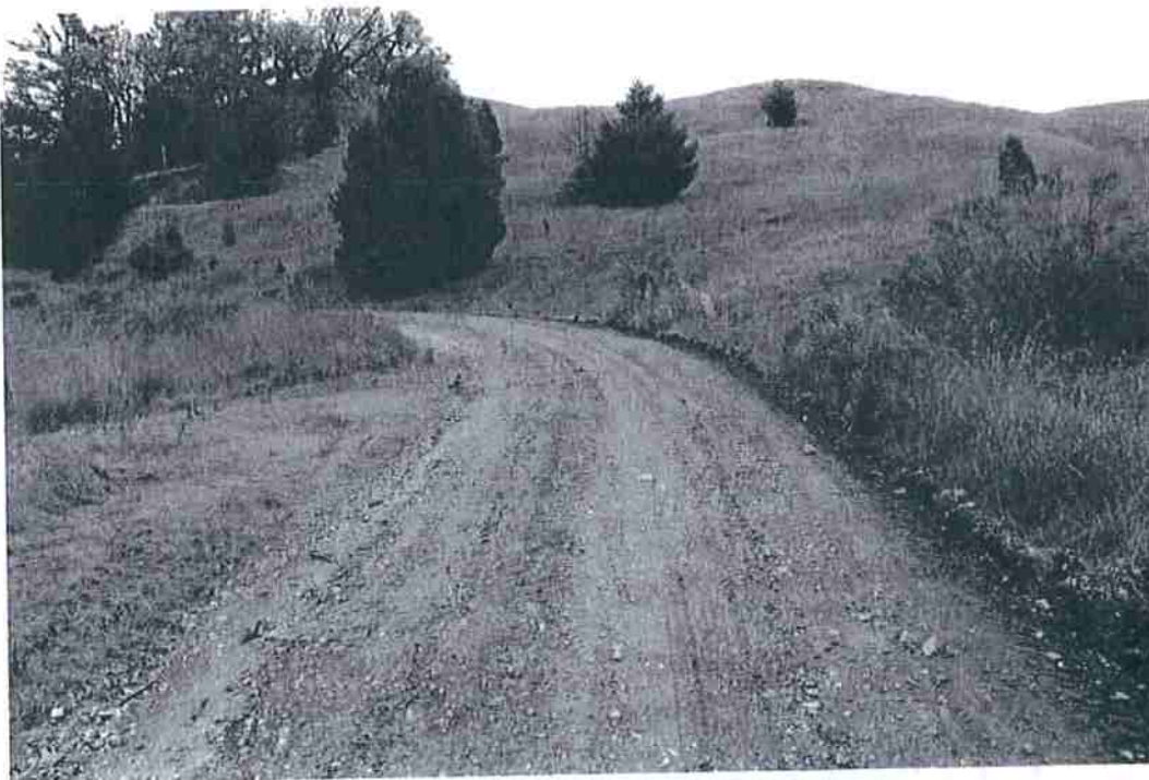
Photo 26 - Mile 2.3: 15' width 2' shoulders, great visibility, with turnouts
