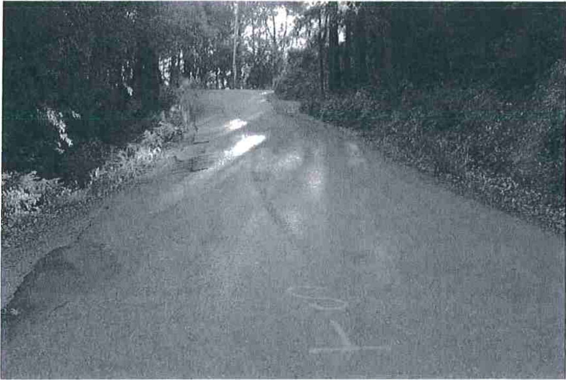
Photo 19. Mile 1.8: 20-ft road width with 2-ft shoulders.
