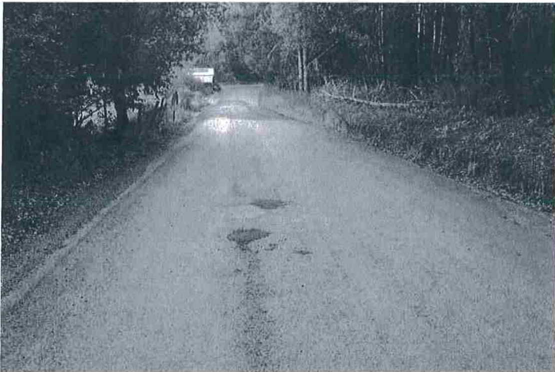
Photo 8. Mile 0.7: 20-ft road width with 2-ft shoulders.
