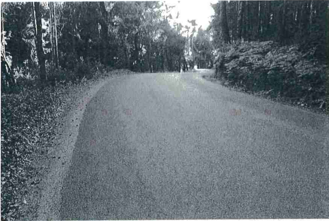
Photo 17. Mile 1.6: 20-ft road width with 2-ft shoulders.
