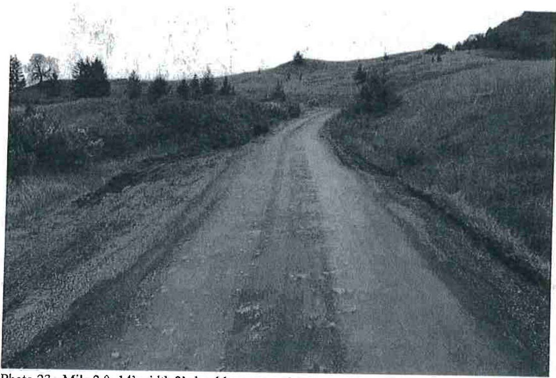
Photo 23 - Mile 2.0: 14' width 2' shoulders, great visibility, with turnouts
