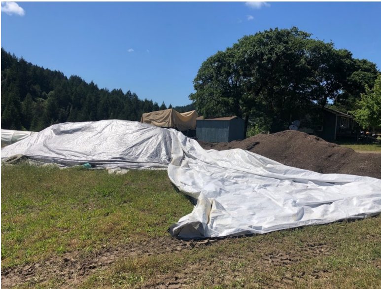
Photo 4: Soil pile with tarp.
