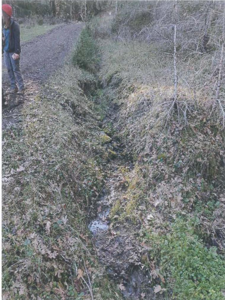
*The photo is facing up the ditch from Site 04. Runoff from off property to the west reaches the seasonal road approximately 120 feet up the ditch line at Site 03. This has resulted in minor ditch erosion from Site 03 to the existing ditch relief culvert at Site 04. This site was described in the recently submitted CDFW LSA Notification No. EPIMS HUM-22462. See treatment prescribed in the Mitigation Report for Site 03. Photo date 1/26/2022.*
