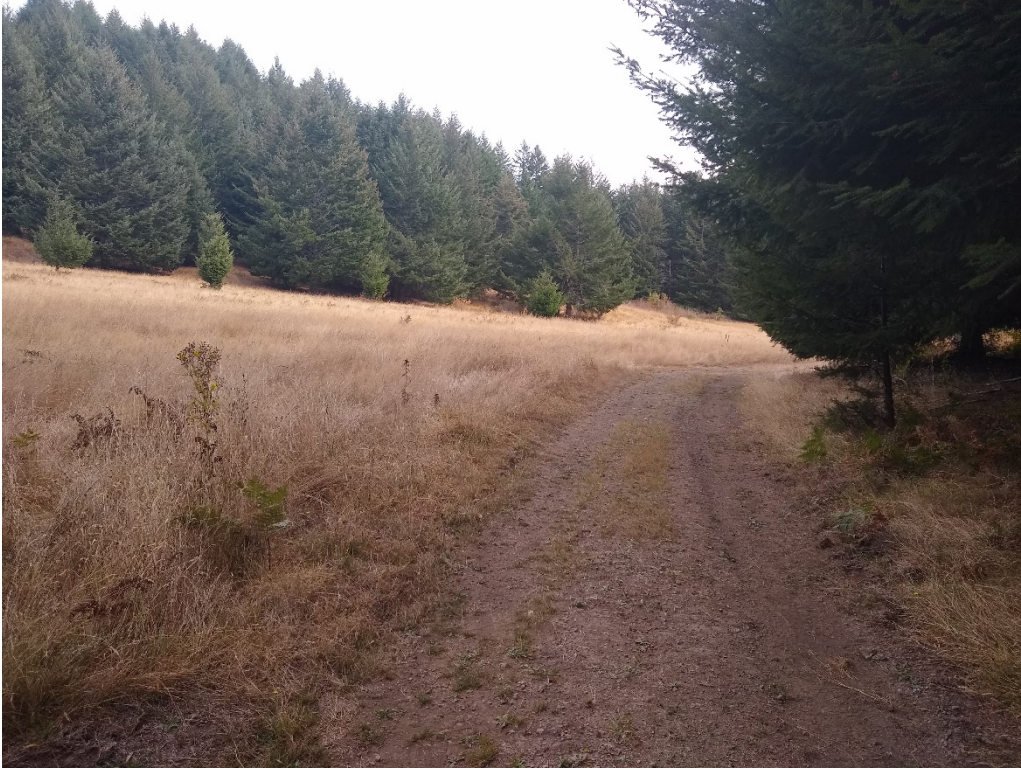
Photo 5. Mile 0.4, looking downslope: 10' road width with 2' shoulders
