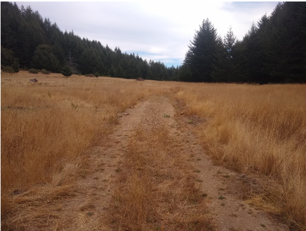
Photo 6. Mile 0.5, looking downslope: 10' road width with 2' shoulders
