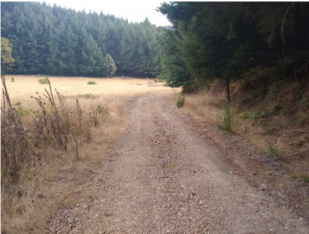
Photo 4. Mile 0.3, looking downslope: 10.5' road width with 2' shoulders.
