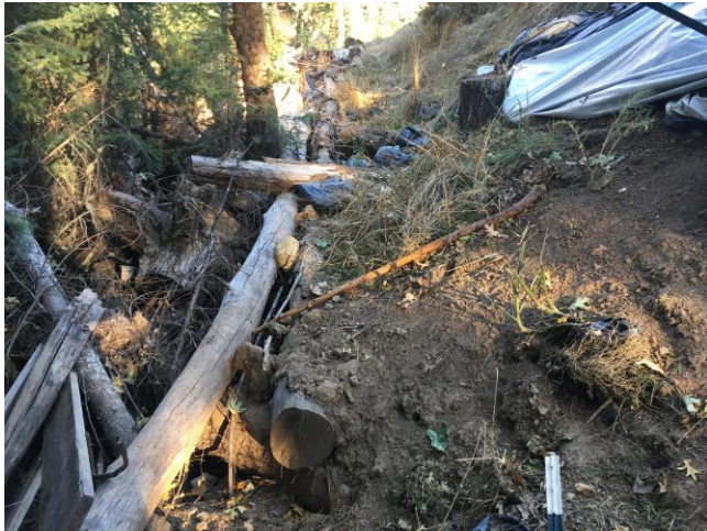
Figure 7. Slash piles and logs supporting fill soil.
