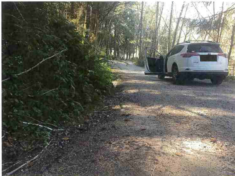
Figure 8: RP4. Outlet of 12' ditch relief culvert. Image facing west; toward Dows Prairie Rd.
