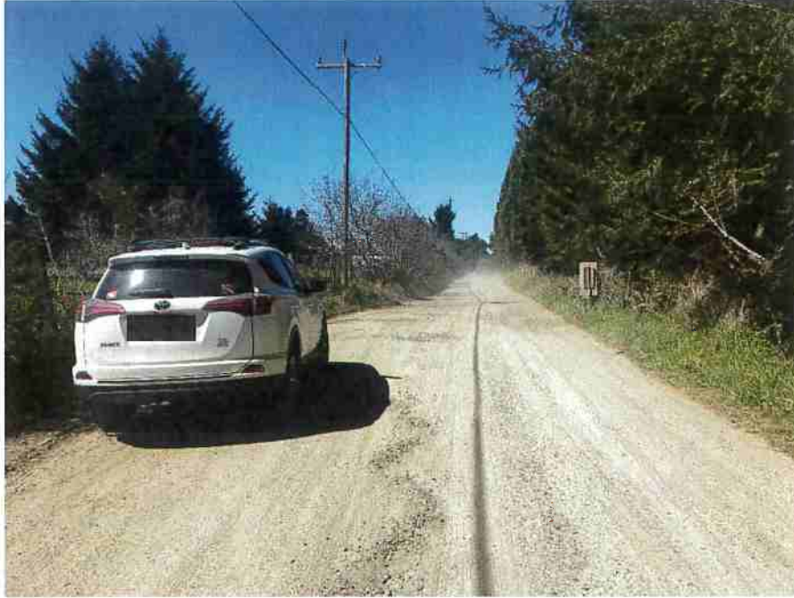
Figure 3: RP 2. Graveled Road Width 16' with 7' wide and 90' long righthand turnout. Image shown facing west.
